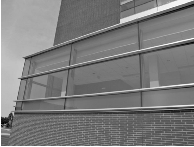
Fig. 8-13. Example of a two-sided SSG curtain wall (capped horizontally and SSG vertically)
