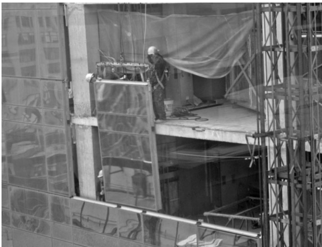
Fig. 8-11. Example of a unitized curtain wall system under installation in a multistory building
