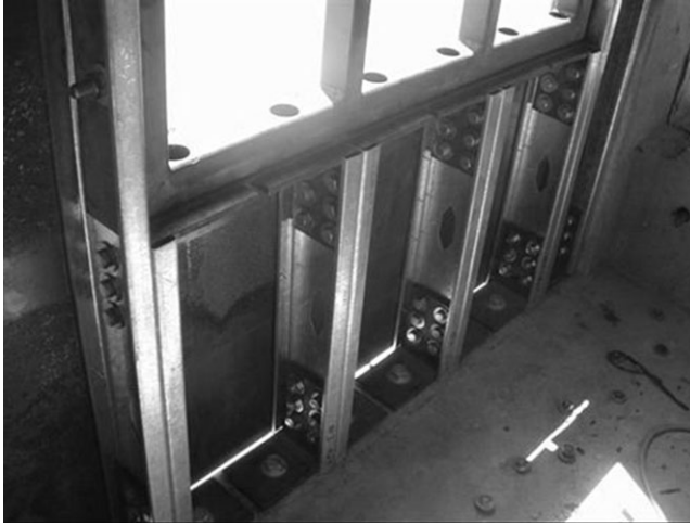
Fig. 9-21. Steel stud blast system
