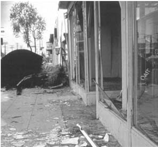
Fig. 8-2. Damage to storefront during Northridge (magnitude 6.7) earthquake of January 17, 1994
