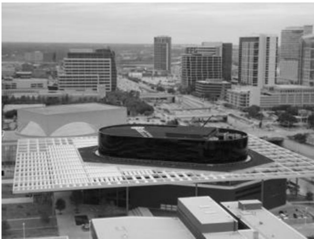
Fig. 3-6. Winspear Opera House, Dallas, TX; example of unique glass color to define aesthetics
