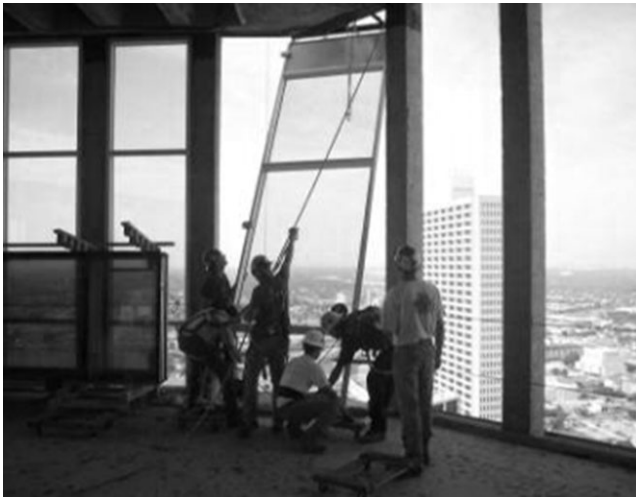
Fig. 3-21. Installing a structurally glazed unit in Ft Worth, TX
