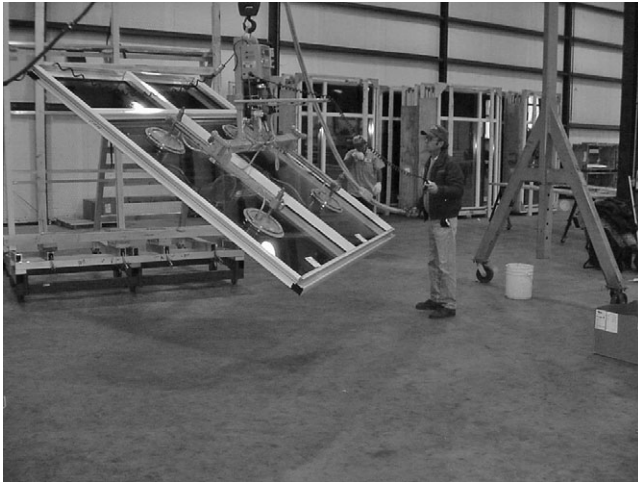
Fig. 4-22. Frame storage and handling
