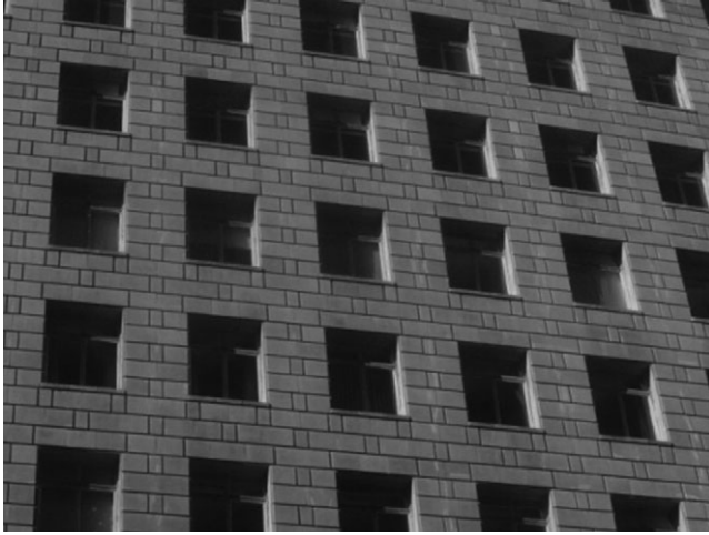
Fig. 9-2. Punched windows Source: FEMA (2009)
