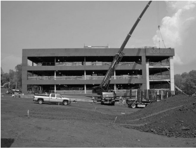
Fig. 3-8. Stone truss panel being installed
