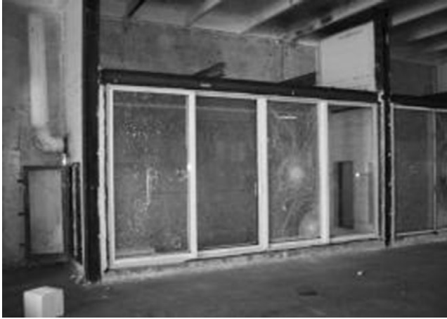
Fig. 4-11. Example of small-frame testing: cyclic testing Source: Courtesy of Thornton Tomasetti; reproduced with permission
