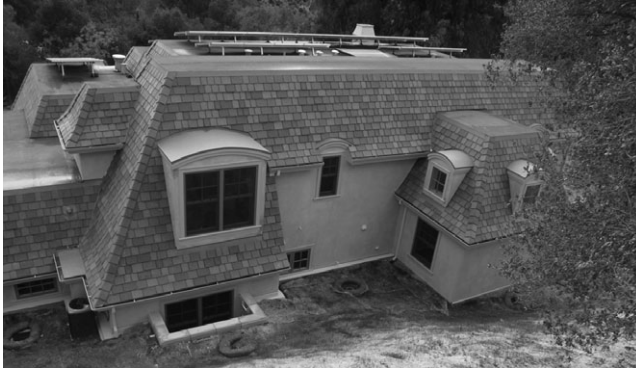
Fig. 11-4. Roof-mount solar arrays and support framing on a house in Los Altos Hills, CA (view from hilltop, solar panels facing downhill)
