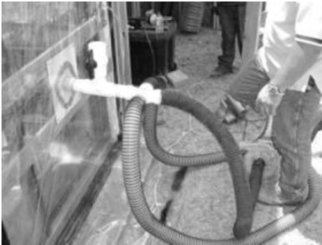
Fig. 4-14. Applying a vacuum to the chamber
