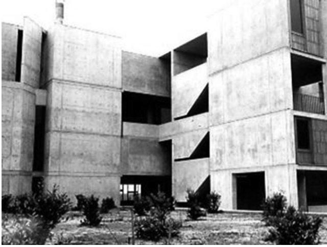
Fig. 9-6. Cast-in-place reinforced concrete envelope Source: FEMA (2009)
