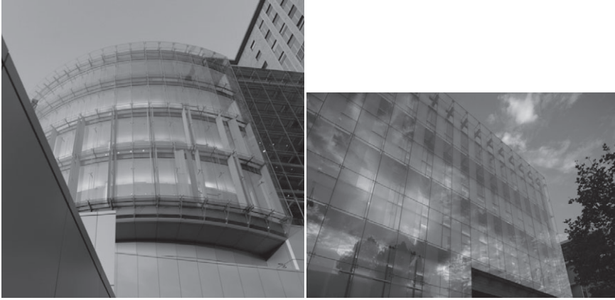
Fig. 3-26. University of Southern California Stem Cell Research Facility, Los Angeles, CA
