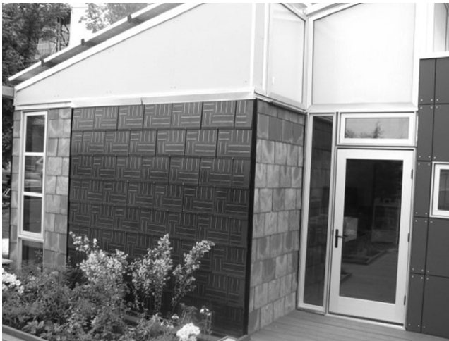
Fig. 11-5. Use of wall-mount (sidings) solar arrays on Solar Decathlon House at Penn State University
