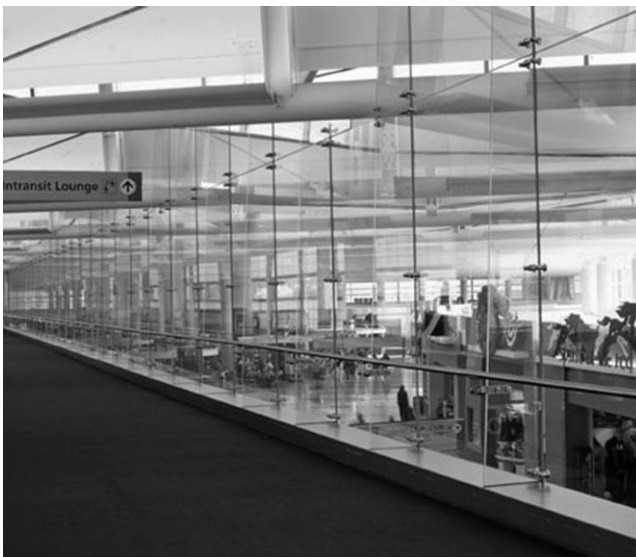
Fig. 3-22. Newark International Airport, NJ; example of point-supported glass and glass fins
