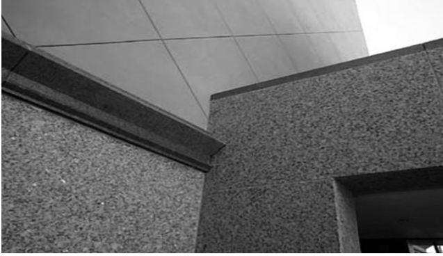
Fig. 3-7. Naples Philharmonic Museum, Naples, FL; an example of natural stone façade (granite)
