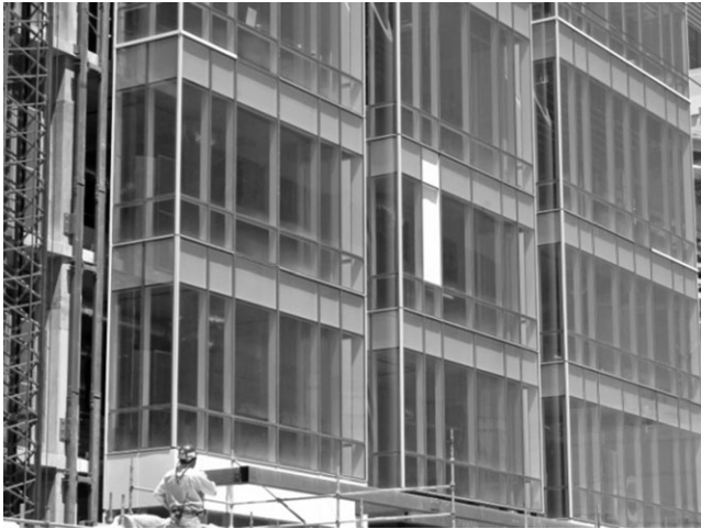
Fig. 8-14. Example of a four-sided SSG curtain wall
