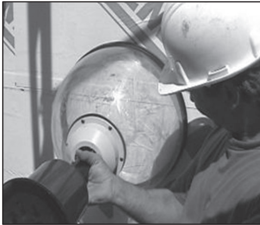
Fig. 4-4. Air tightness test of an envelope component ASTM 1186 Source: Courtesy of Construction Consulting International; reproduced with permission
