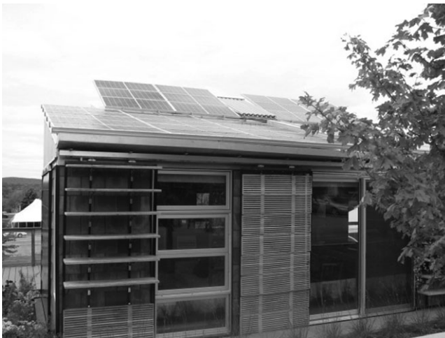
Fig. 11-3. Use of roof-mount solar arrays on Solar Decathlon House at Penn State University
