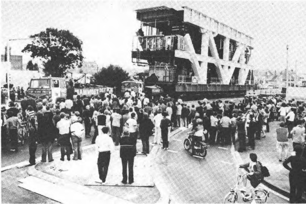
Figure 21.4. A 759-tonne module in the centre of Dunkirk
