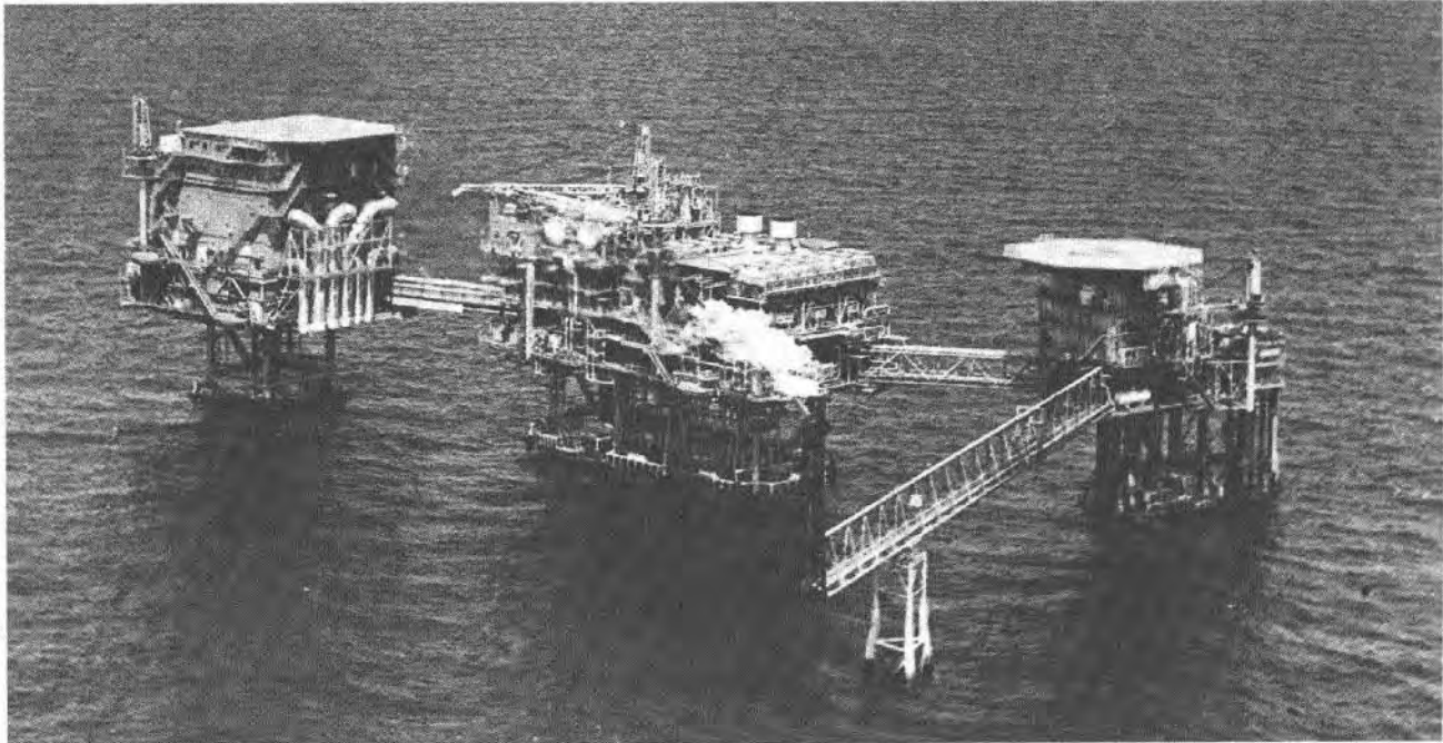
Figure 18.3 The BHS Platform Complex
