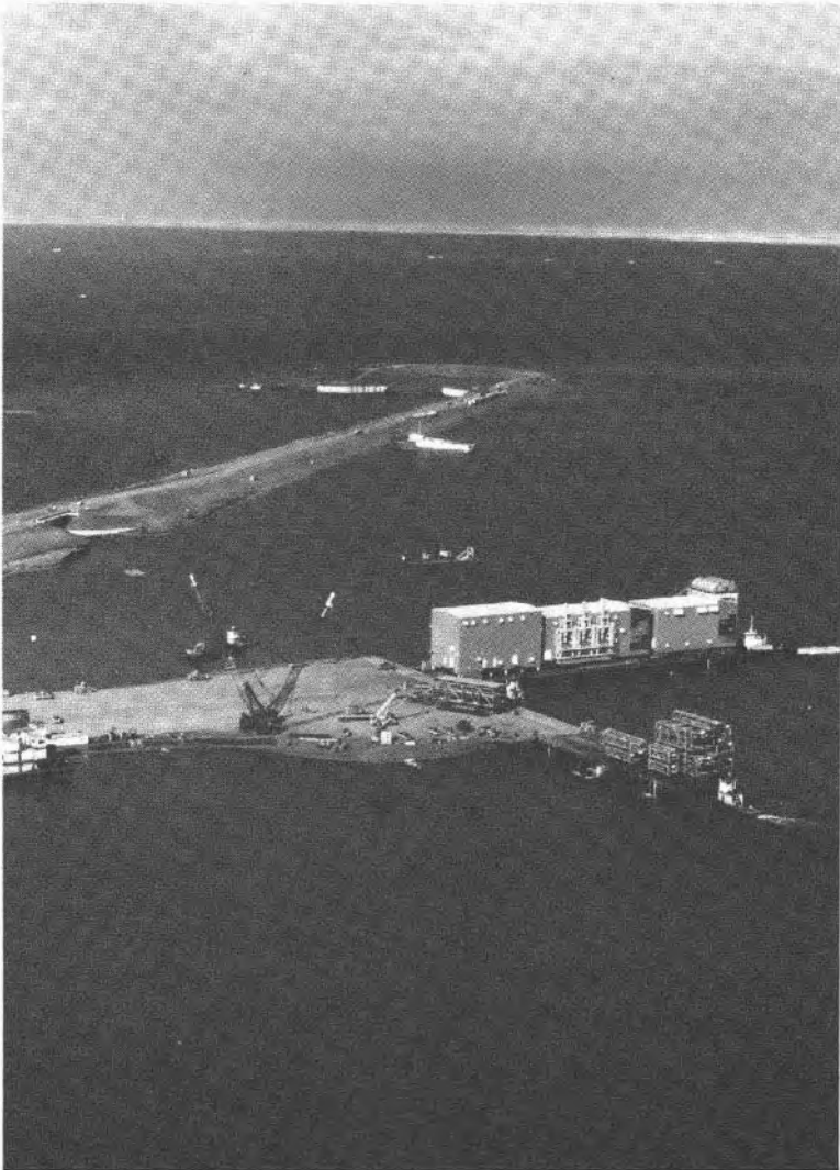
Figure 3.4 Arco's Seawater Treatment Plant
