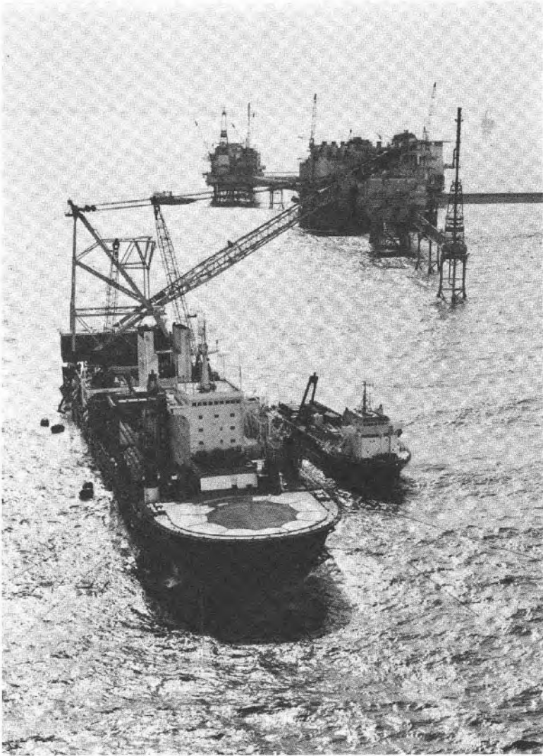
Figure 17.3 Pipelaying vessel ETPM 1601
