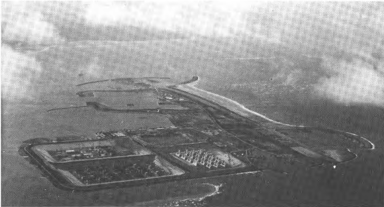
Figure 19.5 The work-island Neeltje Jans This aerial view shows two compartments nearly full of piers in the course of construction and before flooding. (Photograph by permission of Rijkswaterstaat)
