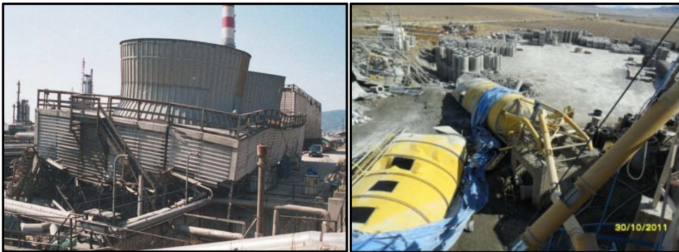
Figure 6: Collapsed silo at SEKA Factory in Izmit (left) and cement silo in Van
