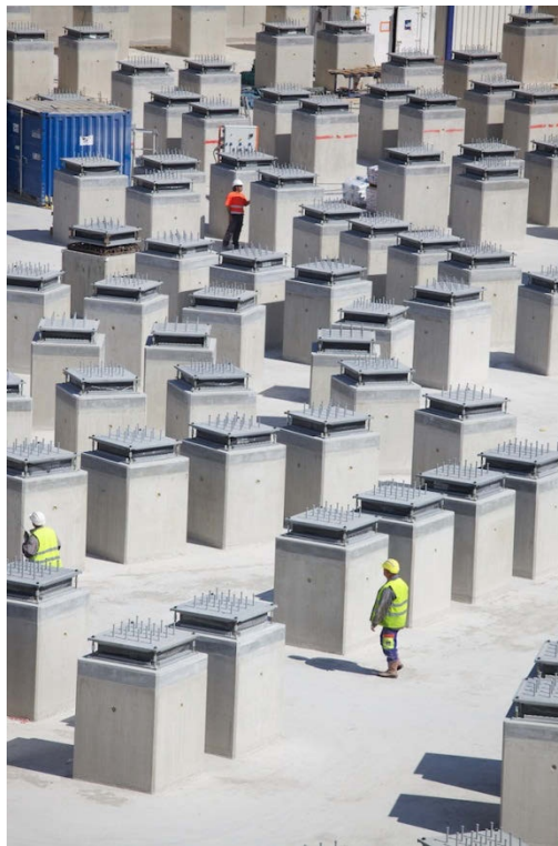
215 Figure 8: Fan-shaped arrangement of the seismic isolation system under the cryostat and 216 Tokamak machine supporting structure
