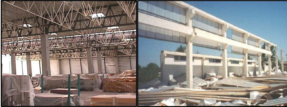
92 Figure 3: Damaged prefabricated buildings at Ford Otosan Plant
