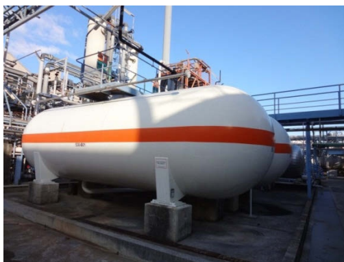
90 Figure 1: Horizontal cylindrical reservoirs resting on four legs system support
