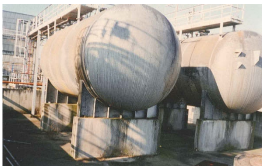
92 Figure 2: Horizontal cylindrical reservoirs resting on saddles of support
