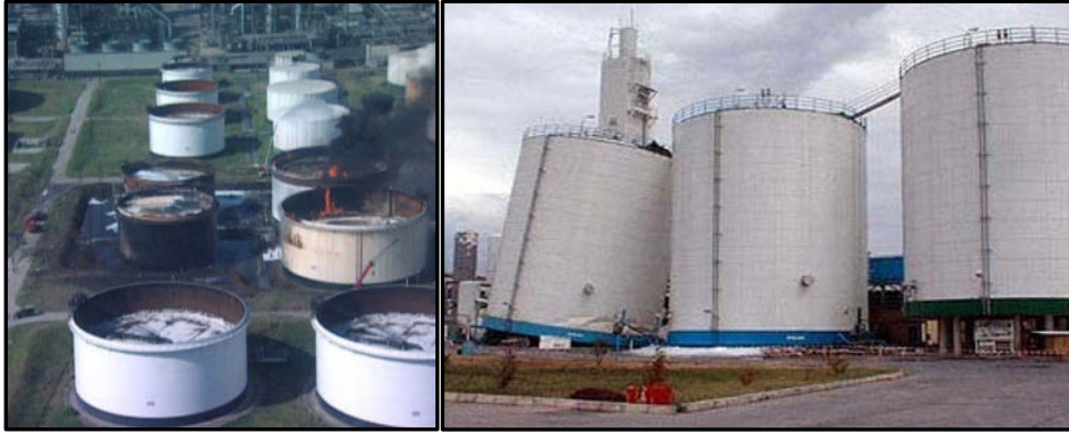
186 187 Figure 8: Damaged tanks at TUPRAS and insulated tanks at HABAŞ Facility
