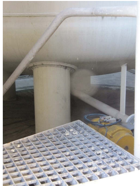
140 Figure 1: Drawing of the analysed Isobutene tank and connection 141 between vessel bottom and steel support feet
