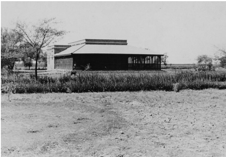
Figure 5.4 Sudan Plantations Syndicate cotton inspector’s house, probably B-type. Reproduced by permission of Durham University Library (F. B. Hunt; SAD.692/19/6)
