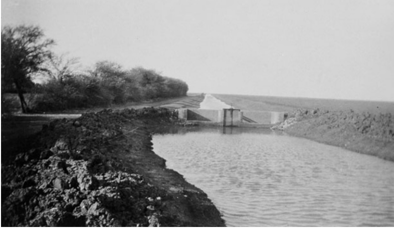
Figure 3.1 Weir on a minor irrigation canal in the Gezira. Reproduced by permission of Durham University Library (F.B. Hunt; SAD.692/19/8)
