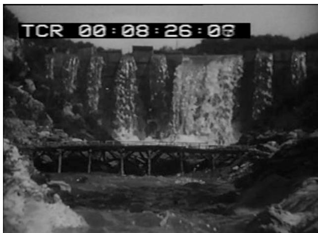
Fig. 7.3 Ken Hall’s image of a scaled-down model of Woronora Dam as seen in Cinesound Productions, Australia is Developing a Dust Bowl (1943). National Film and Sound Archive, Australia
