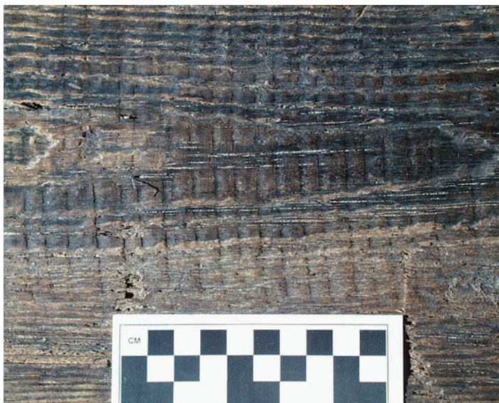
Fig. 6.10 Detail of saw marks visible on interior surface of Bottom Plank B at midships area ( top of image is outboard). These are believed to have been made by a mechanical pit saw, which would date to sometime after ca. 1840
