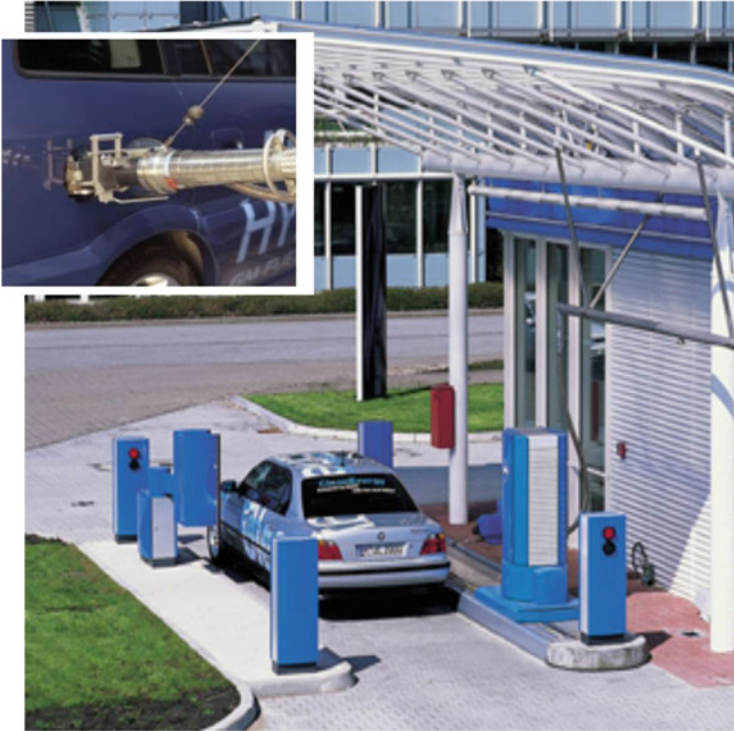
Fig. 3.33 Hydrogen filling station for automobiles (Source: BMW)
