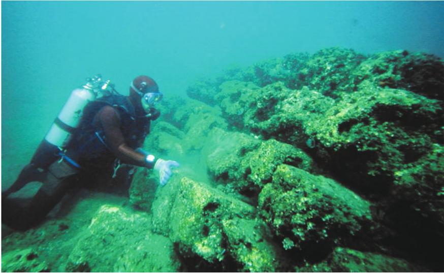
**Fig. 6.3** Diver investigating a collapsed wall made of limestone blocks in the interior of the Temple of Amun-Gereb (*photo* C. Gerigk © F. Goddio/Hilti Foundation)
