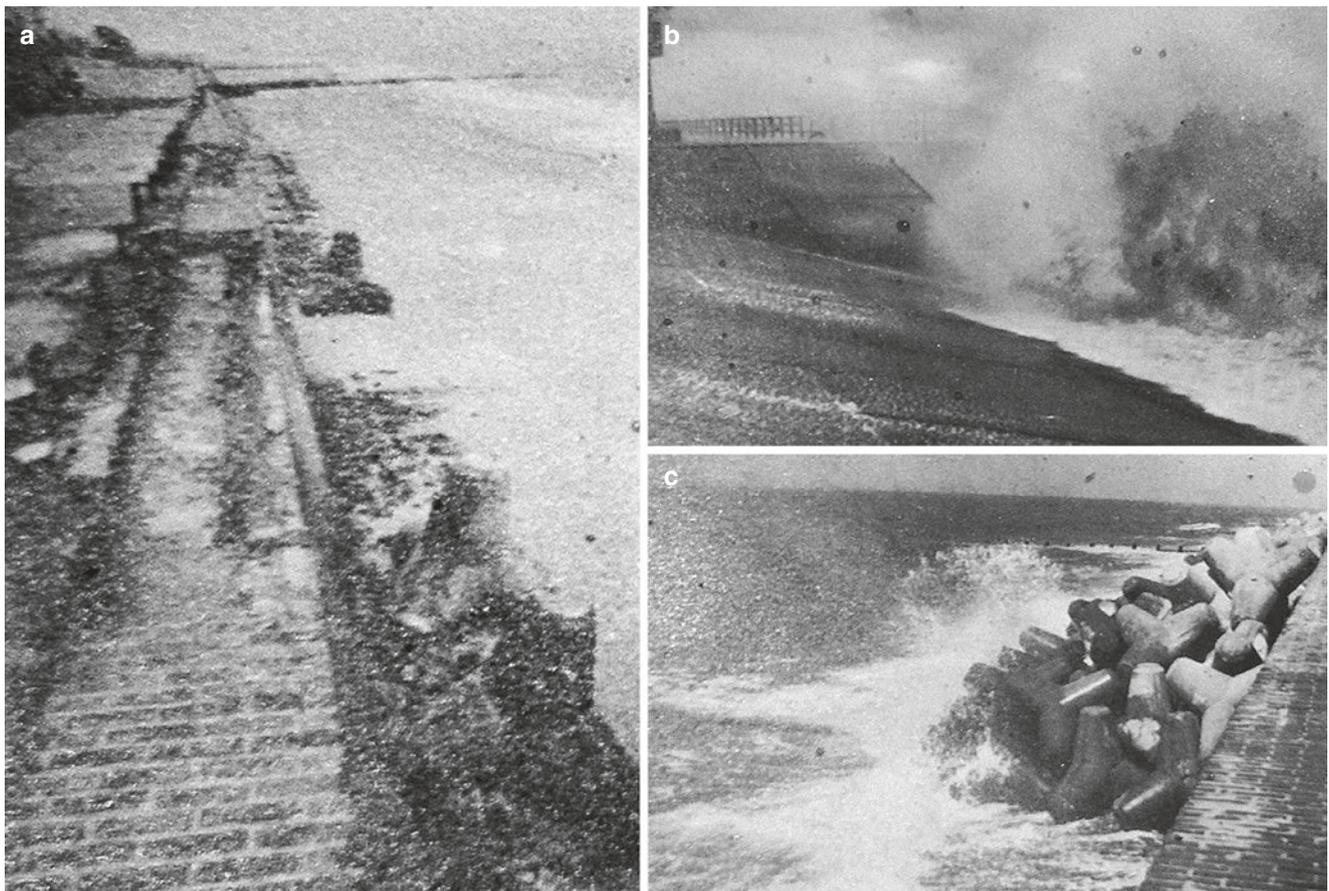
**Fig. 5.10** Defense against violent surf action in Westerland, Island of Sylt, German North Sea. (a) Damaged beach wall and displaced tetrapods; (b) gently sloping wall for breaking the power of storm waves;
