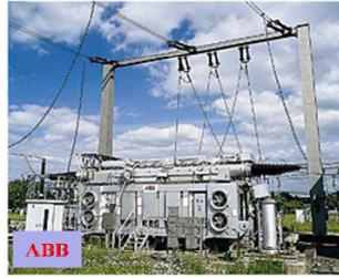
220 kV/115 kV/10kV
