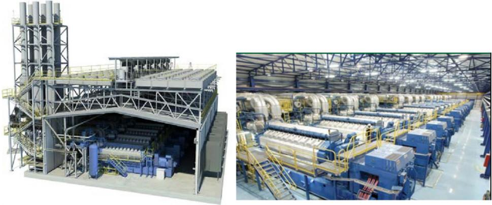
**Figure 3-16:** Engine power plant in multi-unit arrangement, Wärtsilä [20]
