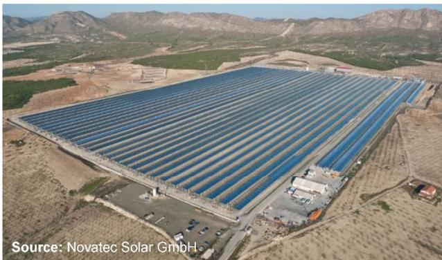
**Figure 5-27:** Solar field of linear Fresnel power plant
