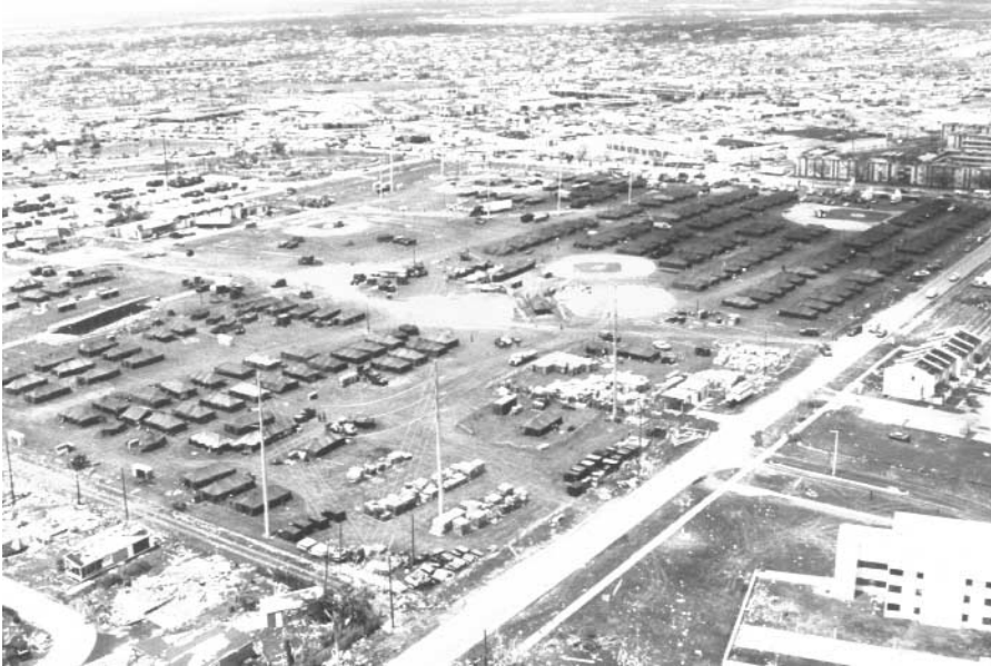
Figure 2-3 Hurricane Andrew, Florida, August 24, 1992. An aerial view showing damage from one of the most destructive hurricanes in America's history. One million people were evacuated and 54 died in this hurricane. FEMA News Photo.
