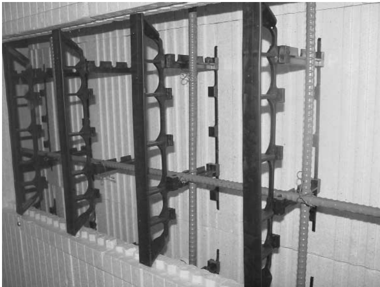
Figure 3-1 November 23, 2001, Tulsa, Oklahoma (Disaster Alley in the Eastland Mall). A safe room wall section is shown here. The insulated concrete form is cut away to show reinforcing steel. The cavity is filled with concrete. Photo by Kent Baxter/FEMA News Photo.
