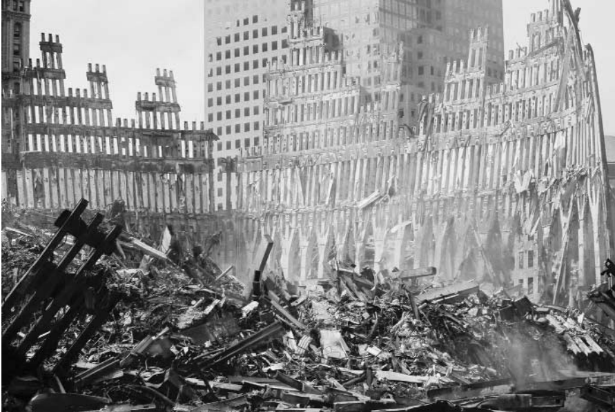
Figure 9-2 New York, NY, September 27, 2001—The remaining section of the World Trade Center is surrounded by a mountain of rubble following the September 11 terrorist attacks. Photo by Bri Rodriguez/FEMA News Photo.
