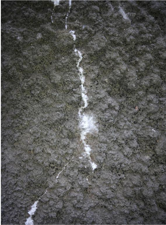
**Figure 3.3** Precipitation of  $\text{CaCO}_3$  from solution of  $\text{Ca}(\text{HCO}_3)_2$  that seeps through the concrete cracks and dries on the concrete surface.
