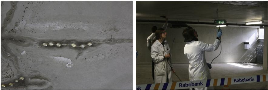
**Figure 12.7** In situ application of the bacteria-based liquid repair system. Manual application using handheld spray units (right image) and counting of water drops permeating per minute through the cracked parking deck (left image).
