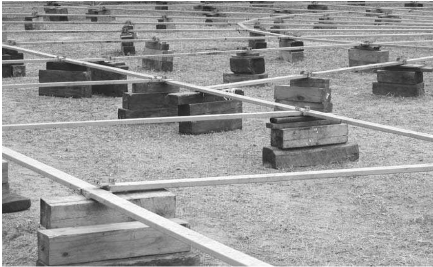
Fig. 5.5 Matrix ground support for roller coaster during setup of the Florida State Fair Midway (Photograph by the author, 2003)
