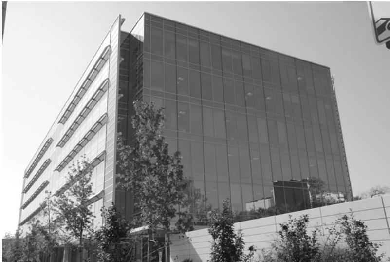
FIGURE 4.1.4 Shell Woodcreek office and multipurpose building complex in Houston, TX as featured on the cover: Western exposure envelope treatments. (Photo taken November 11, 2009 by Heidi Brakewood.)
