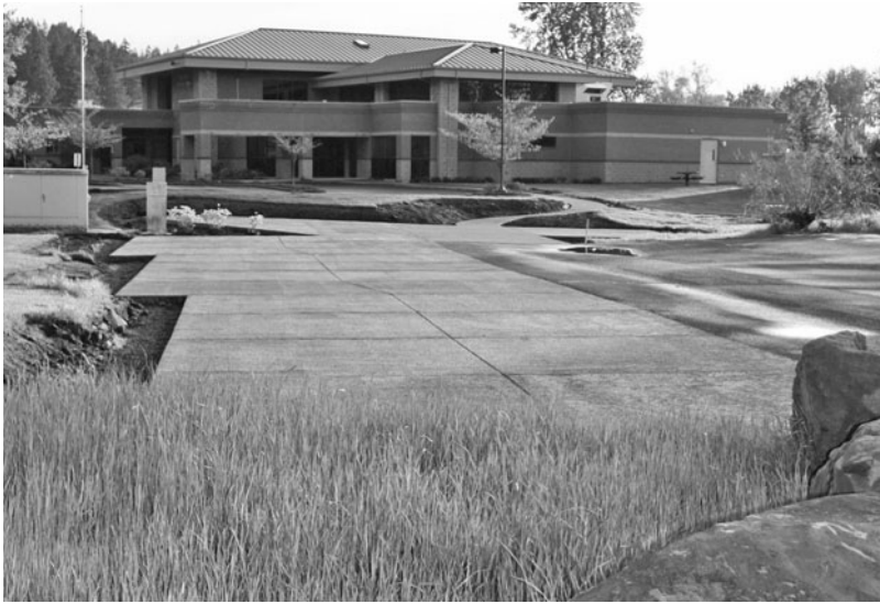
FIGURE 10.1.14 Pervious concrete parking lot in Salem, OR. (Photograph courtesy Scott Erickson of Evolution Paving taken November 2009.)
