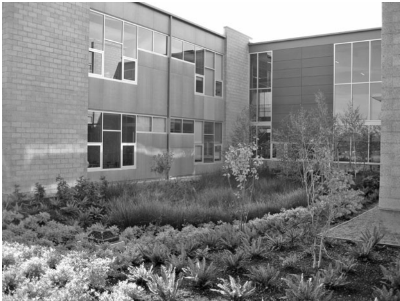
FIGURE 10.1.9 A Gray Middle School rain garden. (Photograph courtesy Coughlin Porter Lundeen taken November 2009.)
