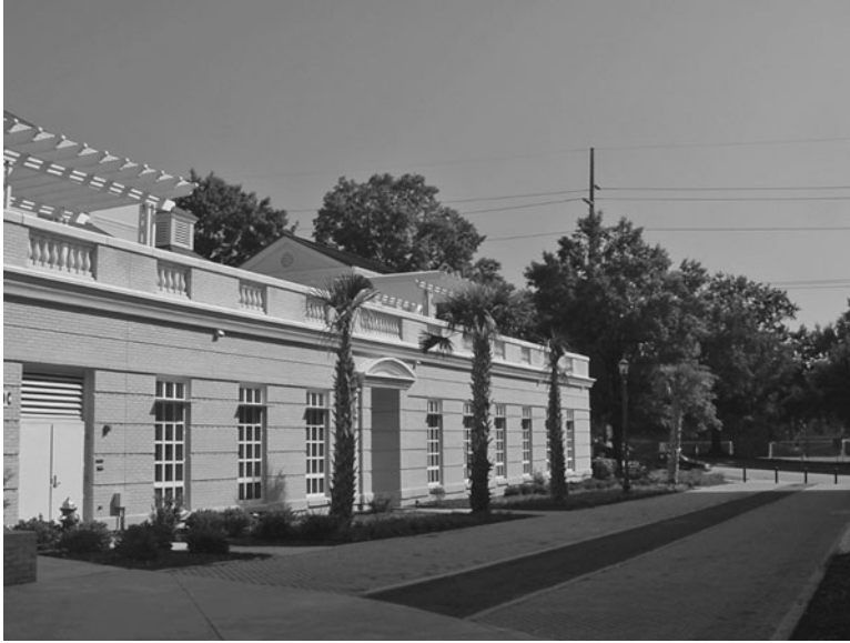
FIGURE 2.7.3 Front of the Learning Center at the West Quad at the University of South Carolina. The roof is partially vegetated and has walkways and architectural shading structures for pedestrian access and use.
