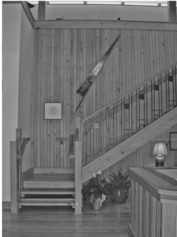
FIGURE 5.3.1 Salvaged wood staircase at Cox and Dinkins, Engineers and Surveyors, Columbia, S.C. (Photograph taken June 2007.)
