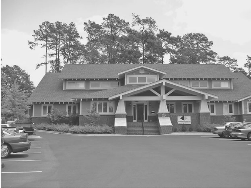
FIGURE 1.2.1 Cox and Dinkins Engineers and Surveyors in Columbia, S.C.: First private building to receive certification under the USGBC LEED-NC rating system in South Carolina. (Photograph taken in June 2007.)
