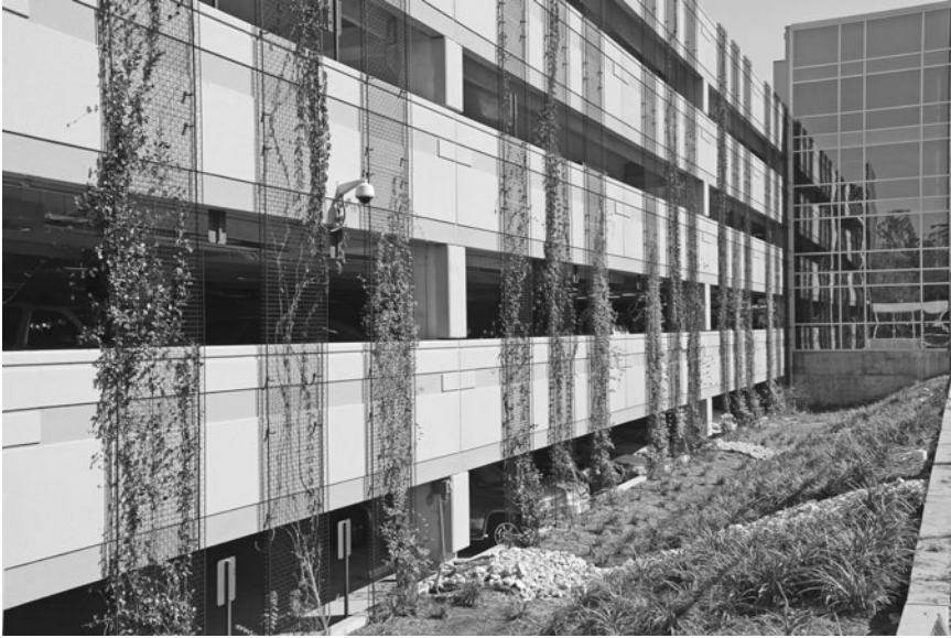
FIGURE 2.7.6 Shell Woodcreek office and multipurpose building complex in Houston, TX. Exterior view of southern wall of new parking garage showing innovative “green wall.” (Photo taken November 11, 2009 by Heidi Brakewood.)
