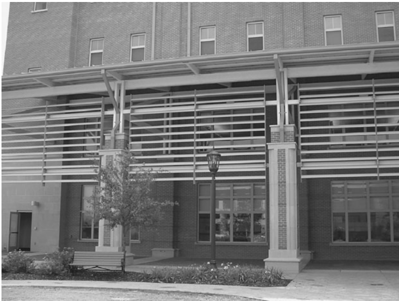
FIGURE 4.1.1 Architectural shading features on the LEED certified Public Health Building at the University of South Carolina, Columbia, S.C. (Photograph taken July 25, 2007.)
