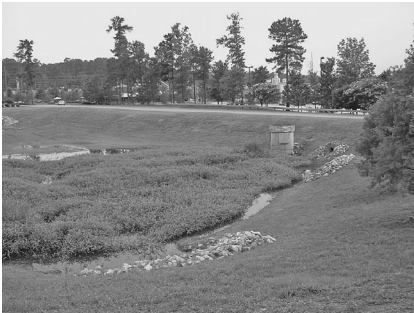
FIGURE 10.1.5 Detention pond with some retention for additional quality control in Irmo, S.C. (Photograph taken July 2007.)
