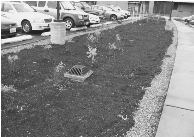
FIGURE 10.1.12 Recently planted rain garden at Ben Franklin Elementary school in Kirkland, WA. (Photograph courtesy Coughlin Porter Lundeen taken October 2007.)
