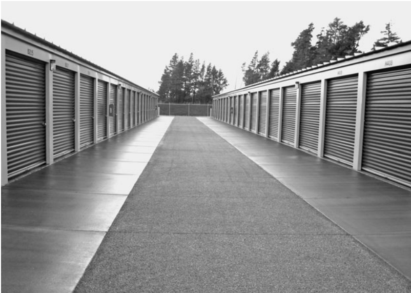
FIGURE 10.2.5 Self storage facility in Florence, OR, with pervious concrete hardscape. (Photograph courtesy Dan Clem of Evolution Paving taken February 2010.)
