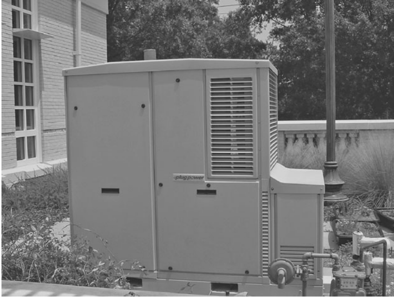
FIGURE 4.7.1 Fuel Cell at West Quad on the University of South Carolina Campus in Columbia, S.C.
