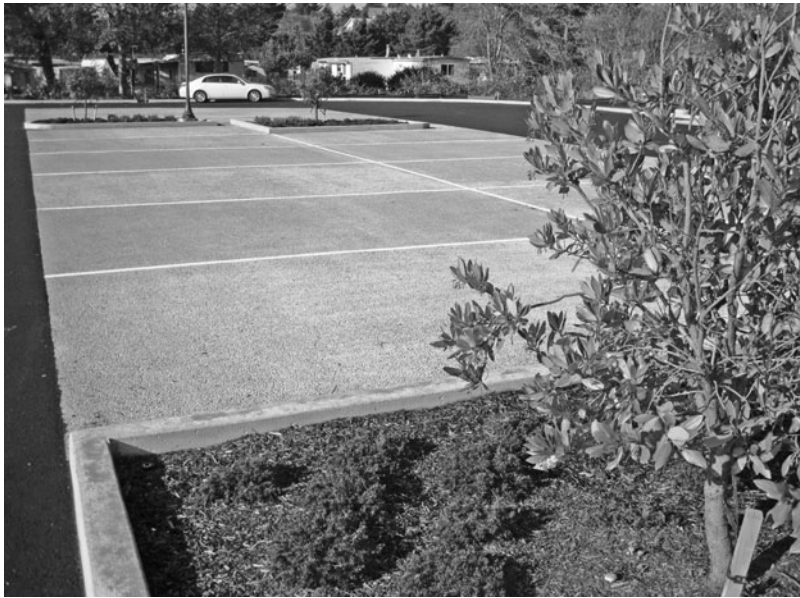
FIGURE 10.1.8 Lincoln City Oregon pervious concrete parking lot. (Photograph courtesy Scott Erickson of Evolution Paving taken November 2009.)
