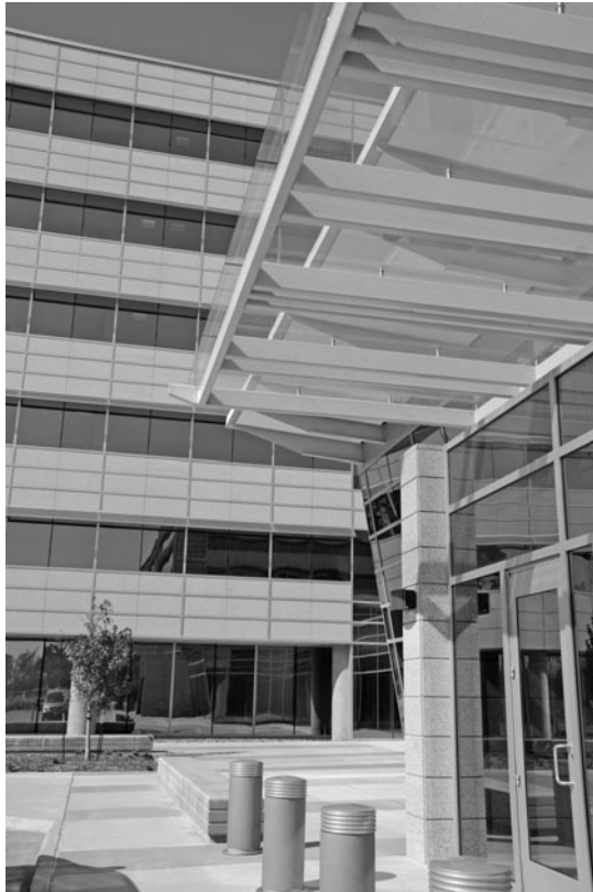
FIGURE 4.1.6 Shell Woodcreek office and multipurpose building complex in Houston, TX: Southern exposure shading features. (Photo taken November 11, 2009 by Heidi Brakewood.)
