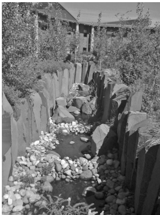
FIGURE 10.1.11 Decorative open conveyance landscape feature at Central Washington University. (Photograph courtesy Coughlin Porter Lundeen taken August 2008.)
