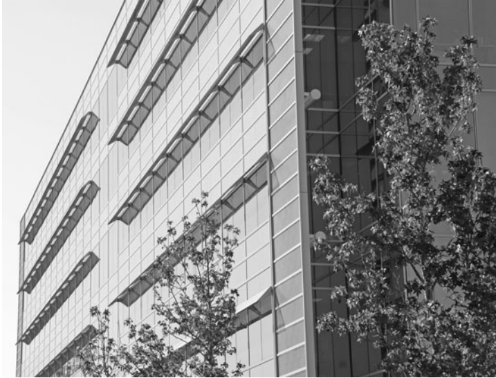
FIGURE 4.1.5 Shell Woodcreek office and multipurpose building complex in Houston, TX: Western exposure envelope treatments close-up view. (Photo taken November 11, 2009 by Heidi Brakewood.)
