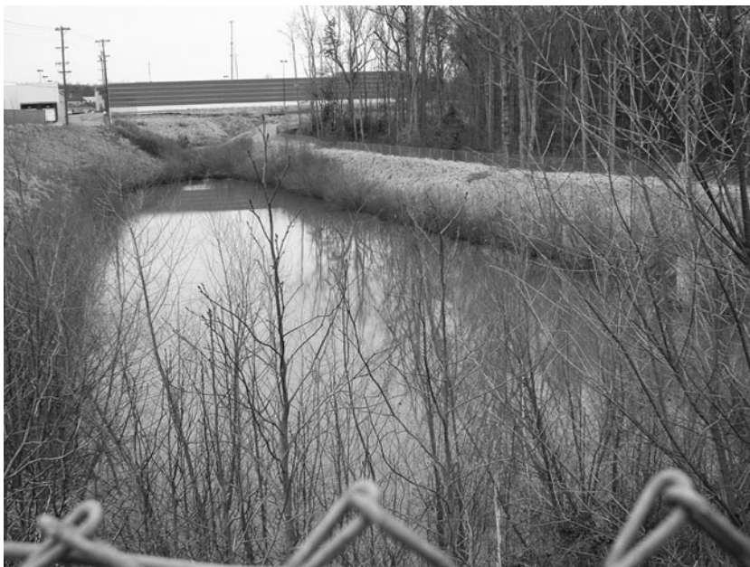
FIGURE 10.1.6 Retention pond in Greenville, S.C. (Photograph taken February 2003.)
