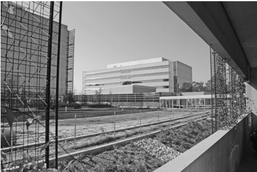
FIGURE 2.7.7 Shell Woodcreek office and multipurpose building complex in Houston, TX. Interior view of southern wall of new parking garage showing innovative “green wall.” (Photo taken November 11, 2009 by Heidi Brakewood.)
