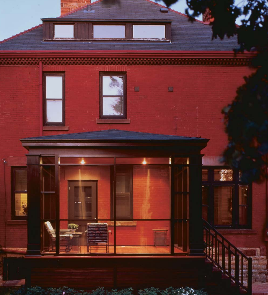
A porch doesn't have to be big. This three-sided porch, with elegant and minimalist detailing, transforms the house for summer living.
