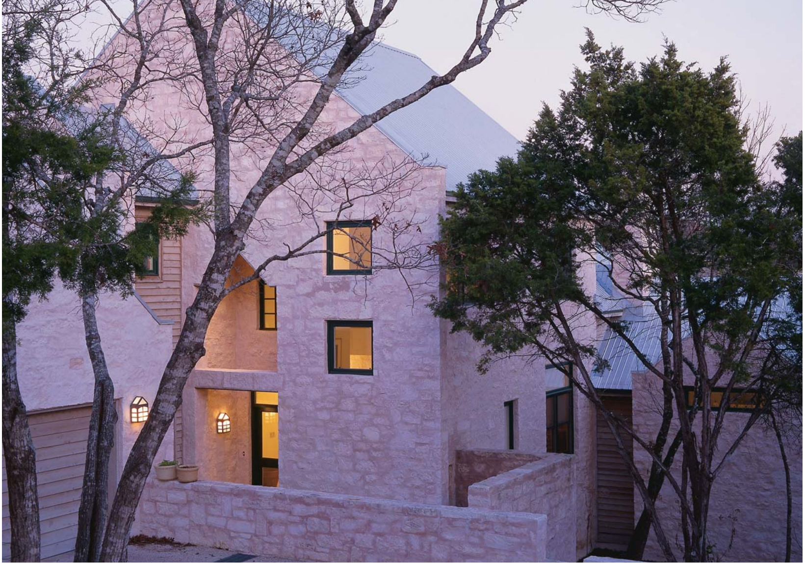
This house, built in a hot climate, was designed to minimize its use of energy and nonrenewable resources. Thick masonry walls and small windows protect the house against summer sun and associated heat gain.
