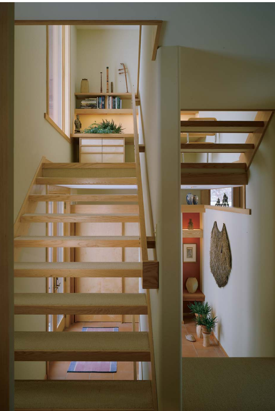
Open stair risers offer filtered views both up and down. A small house like this one benefits from views connecting one level to another, which makes it seem significantly bigger.
