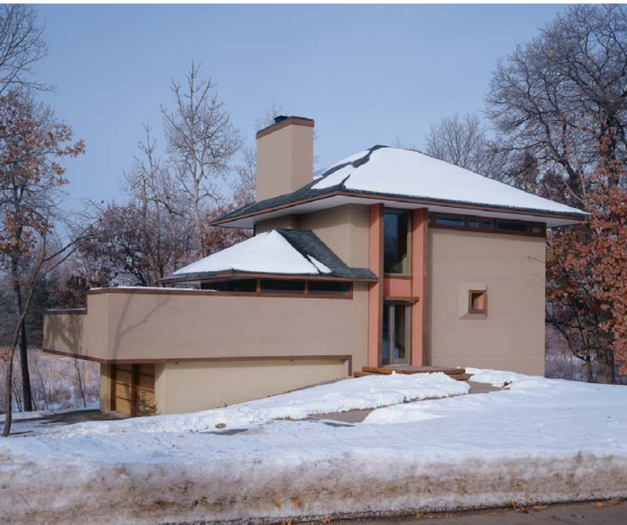
The form of the house is a cube, a very simple and economical shape to build. A screened porch located above the garage extends the cube to the left. There are few windows on the front of the house because it faces a busy street.
