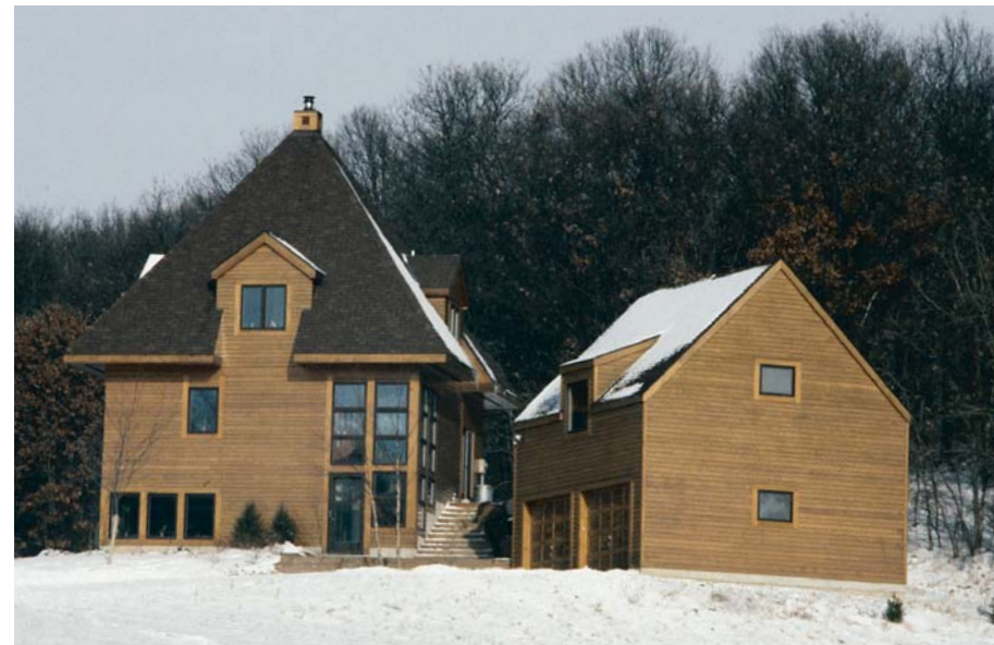
In this energy-efficient house, a two-story window wall on the south side lines the stairway and acts as a passive solar sunspace. Doors at the top and bottom of the stairs can be opened when the temperature within the sunspace rises above 70°F in the winter, bringing heat into the main living areas of the house.
