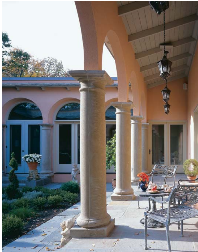
The inspiration for this Minnesota house was an Italian cloister. With broad overhangs and precast concrete columns, a covered walkway connects the house with the outdoors.
