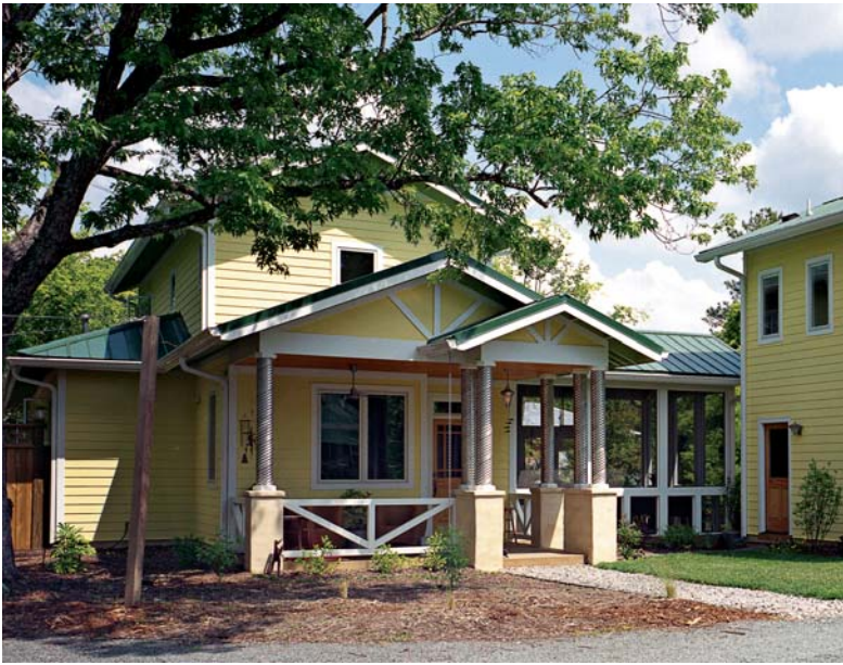
This house in North Carolina, designed by architect Sophie Piesse, uses traditional roof forms but adds a playful touch with galvanized tubing in place of columns, reflecting the owners' love of both natural and industrial materials.
