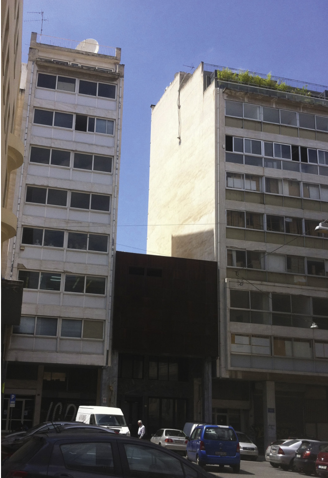
Figure 2.4 A new three-floor building between two nine-story buildings. A.F., Evripidou central Athens area, 2014.
