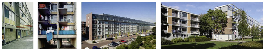
Figure 3.5 Van Shagen in Amsterdam and Kolpa Architecten in Rotterdam (on the right): examples of volumetric compensation (roof-top extension) and creation of new units in the energy retrofitting of existing buildings.
