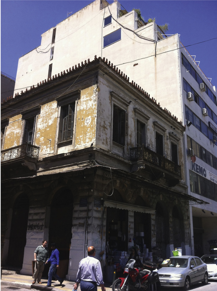
Figure 2.2 A nine-story massive building of the 1980s (on right and in the background) coexists with a two-floor historical building. A.F., Evripidou central Athens area, 2014.
