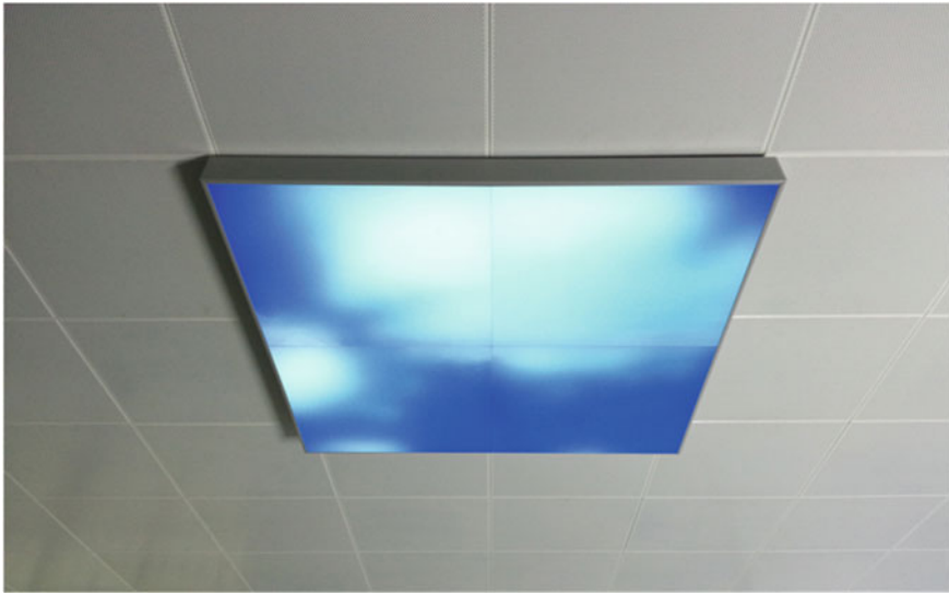
Fig. 17.3 Moving Sky Panel using dynamically controlled RGB LEDs to simulate a skylight (courtesy of SHENZHEN NEONNY TECHNOLOGIES CO., LTD.). Continued improvements in LED efficiency and packaging technology will enable the creation of energy efficient, high resolution video—illumination dual function systems
