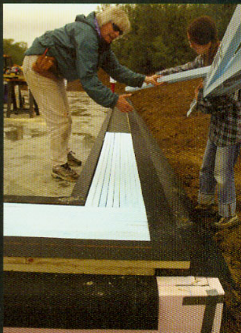
Detail of base plates with insulation
