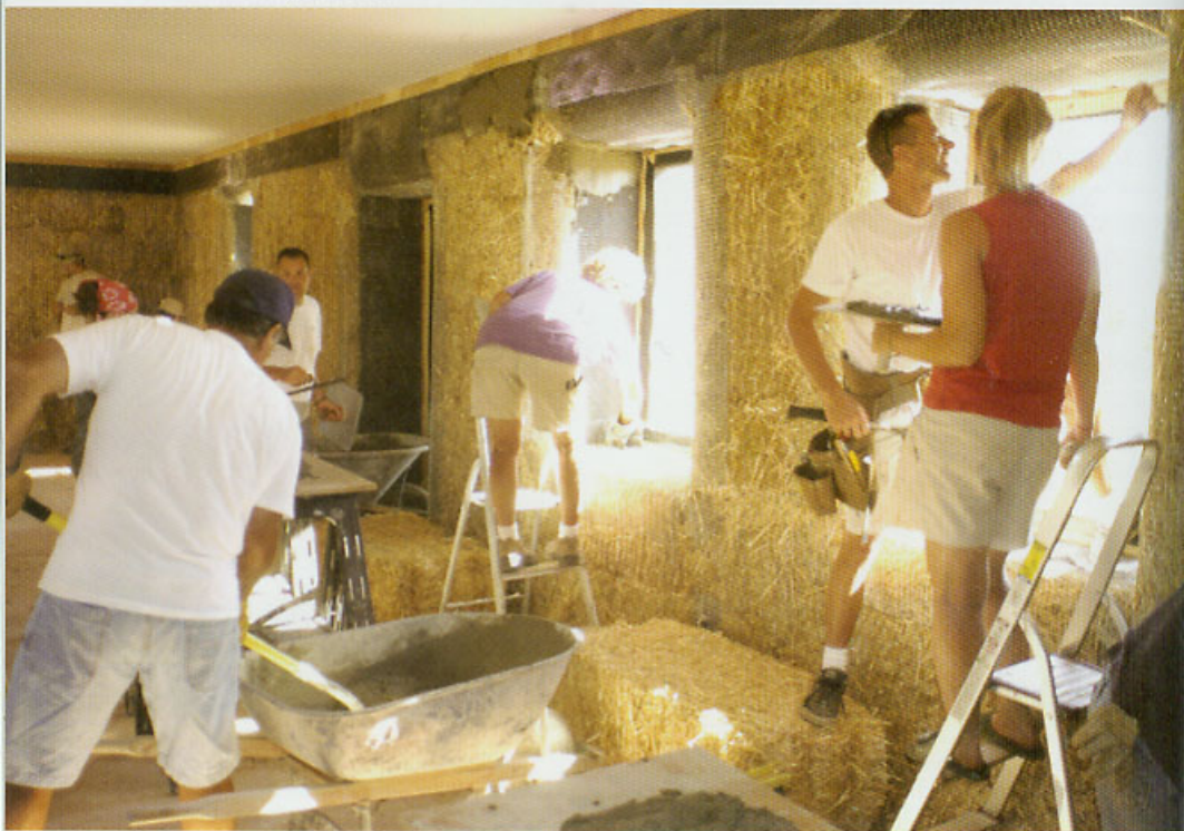
Groups make stuccowork go quickly. Note screed board at the top of the wall.
