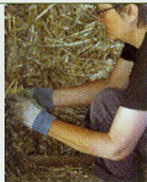
Use loose straw to fill the gaps.
