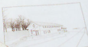
30' EXTERIOR VIEW - FRONT
