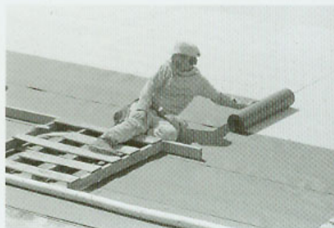
Covering a new roof with waterproof membrane
