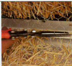
Trimming lath within the weep screed
