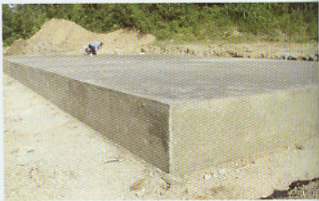
The completed slab awaits straw bales.
