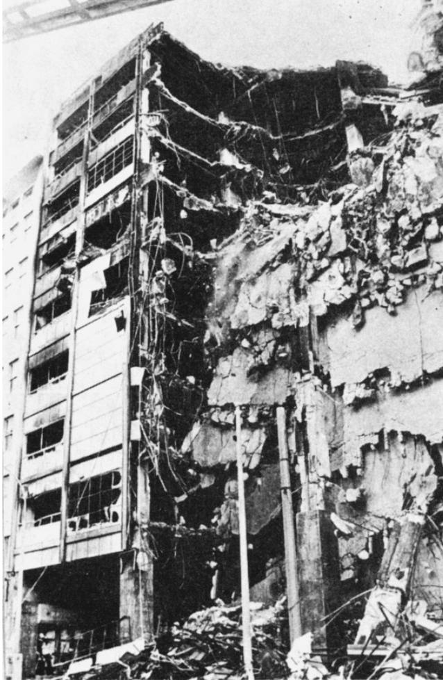
**Figure 7.3** Major structural damage to a multi-storey reinforced concrete department store (Athens, Greece, 1980). Reproduced from Papaioannou (1986) by permission of John Wiley & Sons, Ltd
