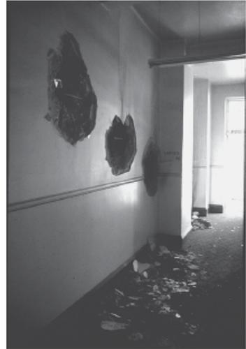
**Figure 6.2** (a) Severe fire in a theatre, showing collapsed steel roof trusses in the foreground; the gallery seating which did not collapse is visible in the upper background. (b) Buckling of a compression member in the heavy steel truss supporting the gallery seating; this truss is close to failure, but did not collapse. (c) Holes punched through a reinforced concrete wall by thermal expansion of the heavy steel truss supporting the gallery seating
