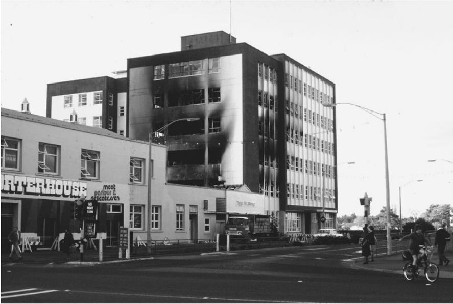
**Figure 7.1** Non-structural fire damage to a typical reinforced concrete office building
