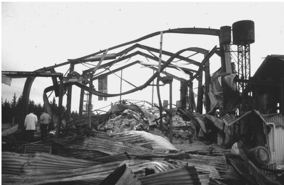
**Figure 6.1** Typical fire damage to unprotected steel frames in an industrial building
