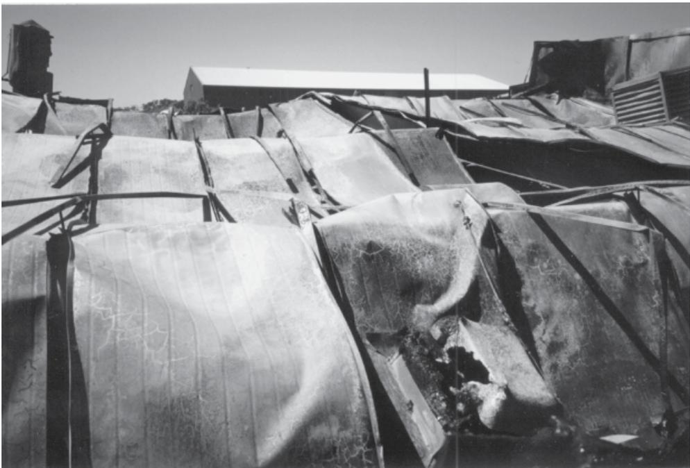
**Figure 10.28** (a) Fire damage to foamed plastic sandwich panels in a factory fire. The building to the right of the photo was completely destroyed by the fire. (b) Steel skins of sandwich panel roofing, draped over the supporting structure after the fire
