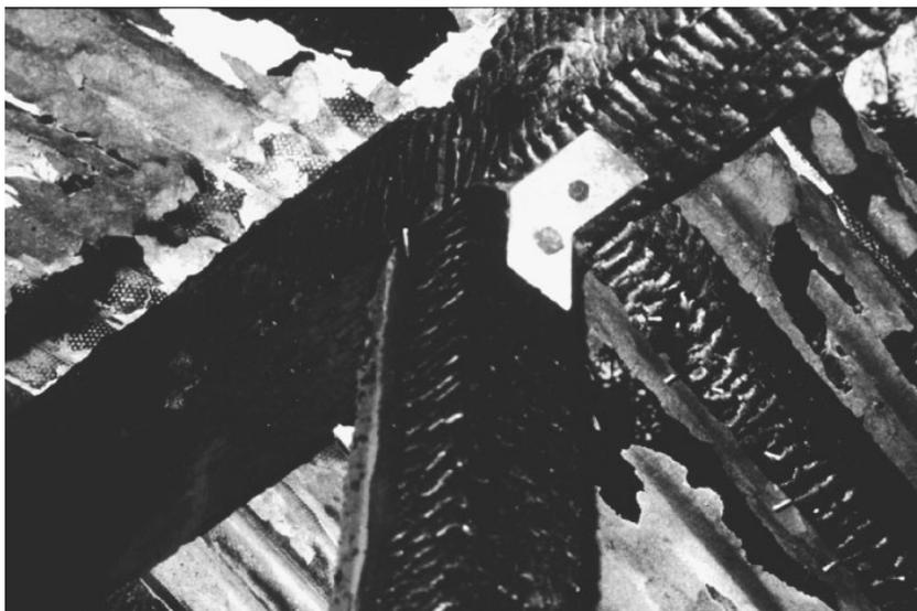
**Figure 9.27** Bolted connection between timber members, after fire exposure
