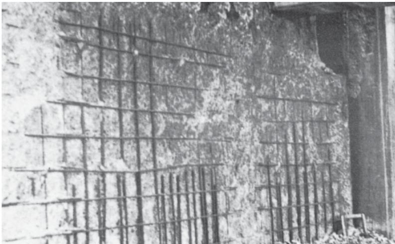
**Figure 7.2** (a) A multi-storey office building engulfed in flames. The reinforced concrete structure did not collapse in the fire (Sao Paolo, Brazil, 1972). (b) Severe spalling of a reinforced concrete wall in the fire
