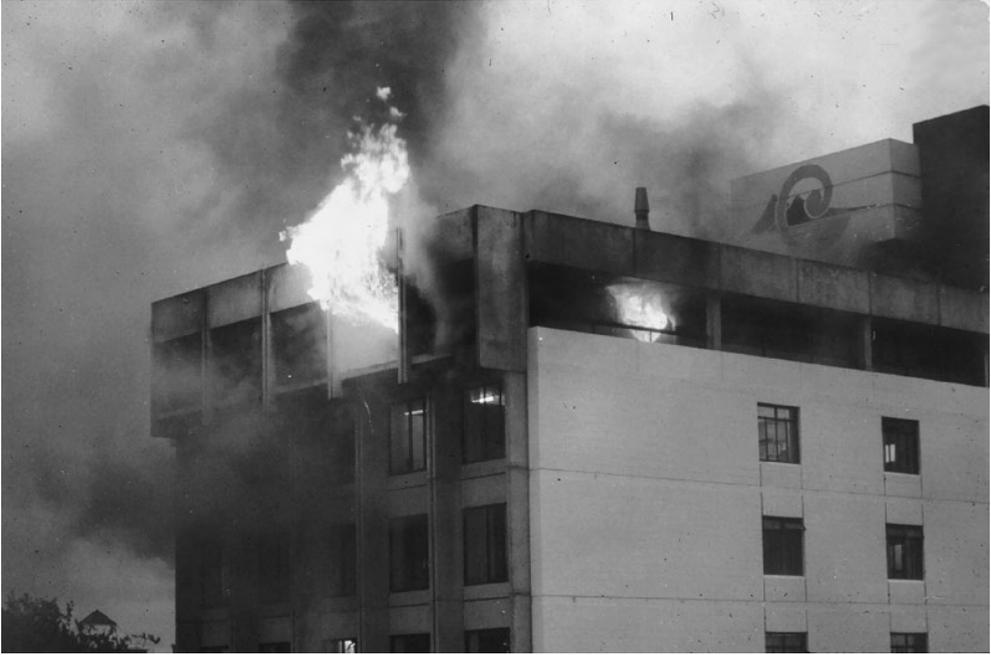
**Figure 3.8** Post-flashover fire on the top floor of a multi-storey office building. The flames coming out of the windows indicate that this fire is ventilation controlled
