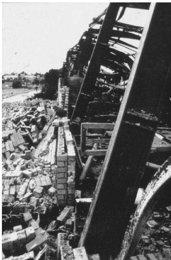
**Figure 8.16** Failure of an unreinforced brick masonry wall of an industrial building; the wall was pushed outwards by thermal expansion of the steel portal frames, which later collapsed inwards. Reproduced by permission of the Cement and Concrete Association of Australia
