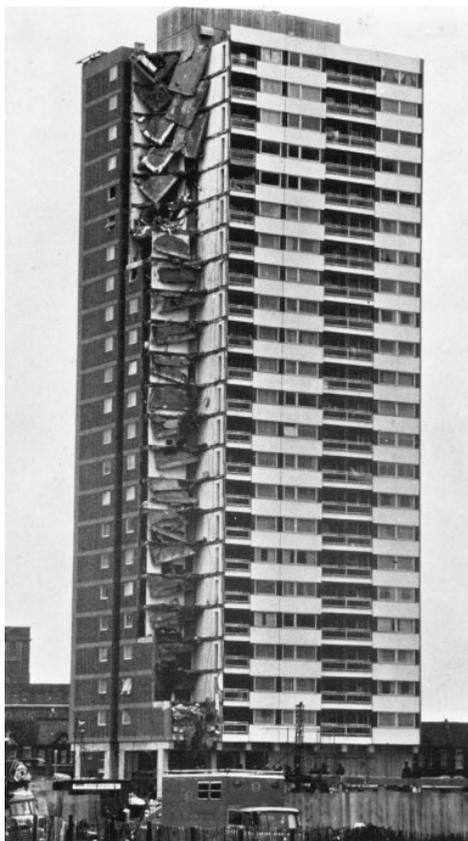
**Figure 5.10** Multi-storey apartment building after a gas explosion caused disproportionate collapse to upper floors. Reproduced from HMSO (1968) by permission of Building Research Establishment, UK
