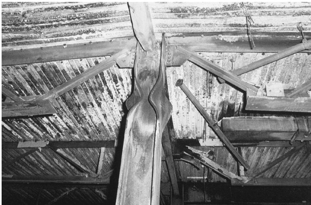
**Figure 8.11** Local buckling of an unprotected steel column during a fire in a building under construction (Broadgate, London, 1990) (SCI, 1991)
