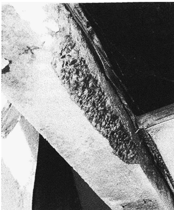
**Figure 7.4** Local spalling at the corner of a concrete beam
