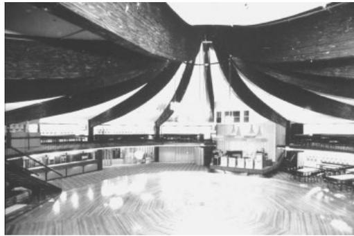
**Figure 9.3** Curved glulam roof beams after repair following a severe fire. Reproduced by permission of Timberlab
