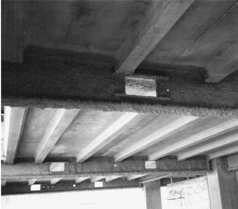
**Figure 6.12** Sprayed-on fire protection to steel beams supporting precast concrete floor slabs
