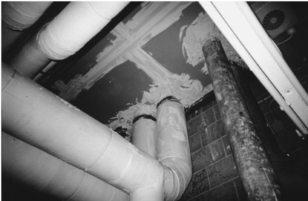
**Figure 2.9** Fire protection to service penetrations through a fire resisting floor
