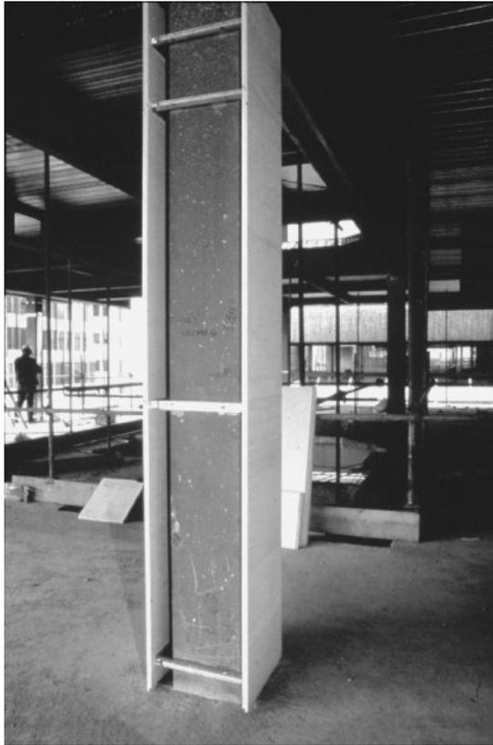
**Figure 6.11** Box protection being placed on a steel column using sheet material
