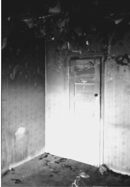
**Figure 3.4** Smoke damage following a pre-flashover fire in a room, indicating the thickness of the hot upper layer during the fire
