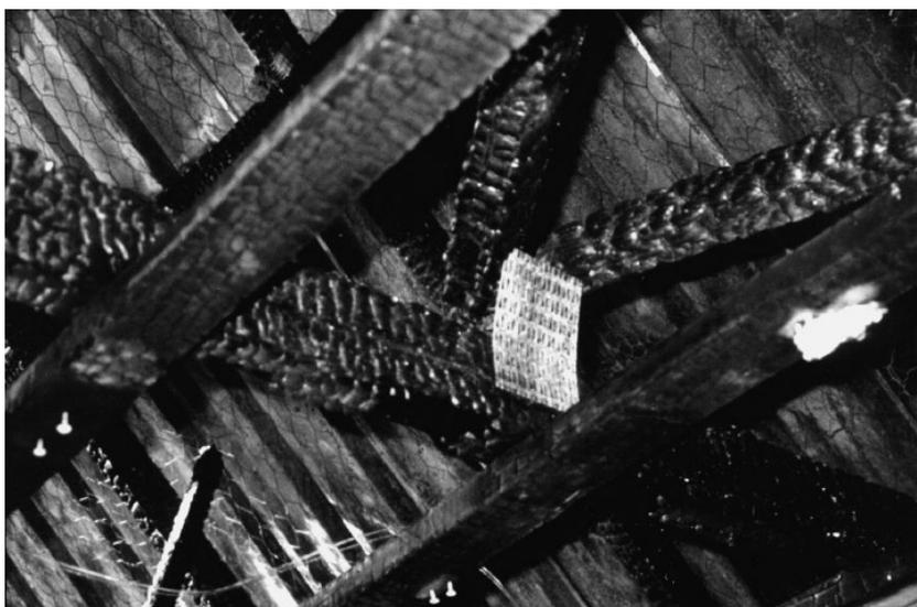
**Figure 9.28** Truss plate connection between timber members, after fire exposure
