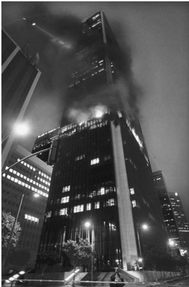
**Figure 2.6** Fire on the 12th floor of a 62 storey building, illustrating the importance of providing both containment and structural stability. Reproduced by permission of Boris Yaro
