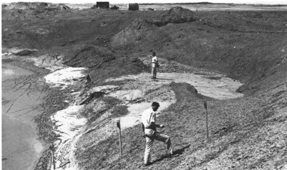
Figure 5.10 Internal shot of portion of crater taken soon after the explosion when ground water was beginning to seep into the base of the structure (after G.H.S.Jones).
