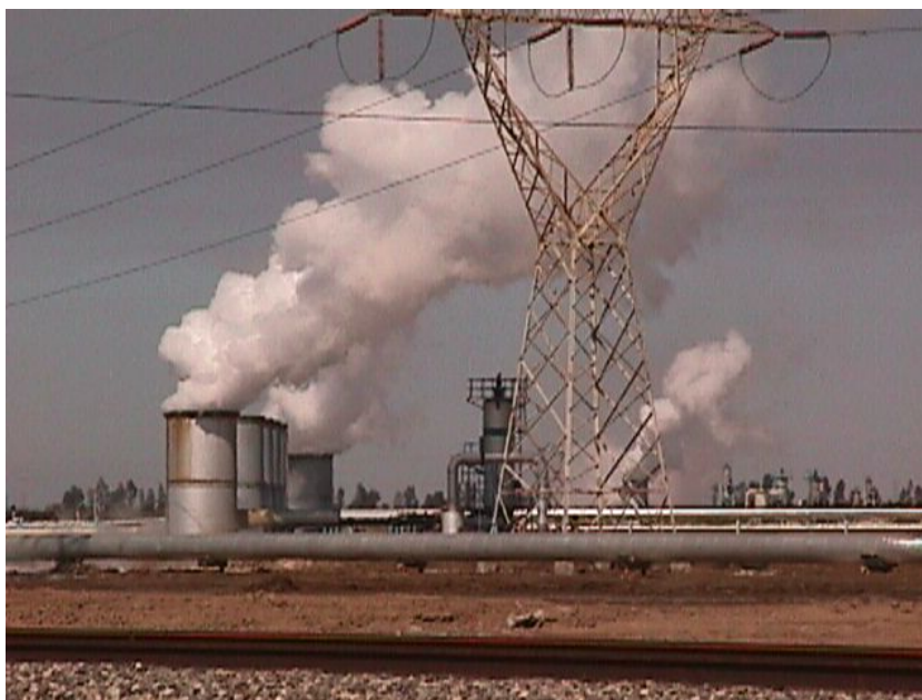
Figure 16. A humid corrosive environment in a geothermal field caused by steam and gases emission.
