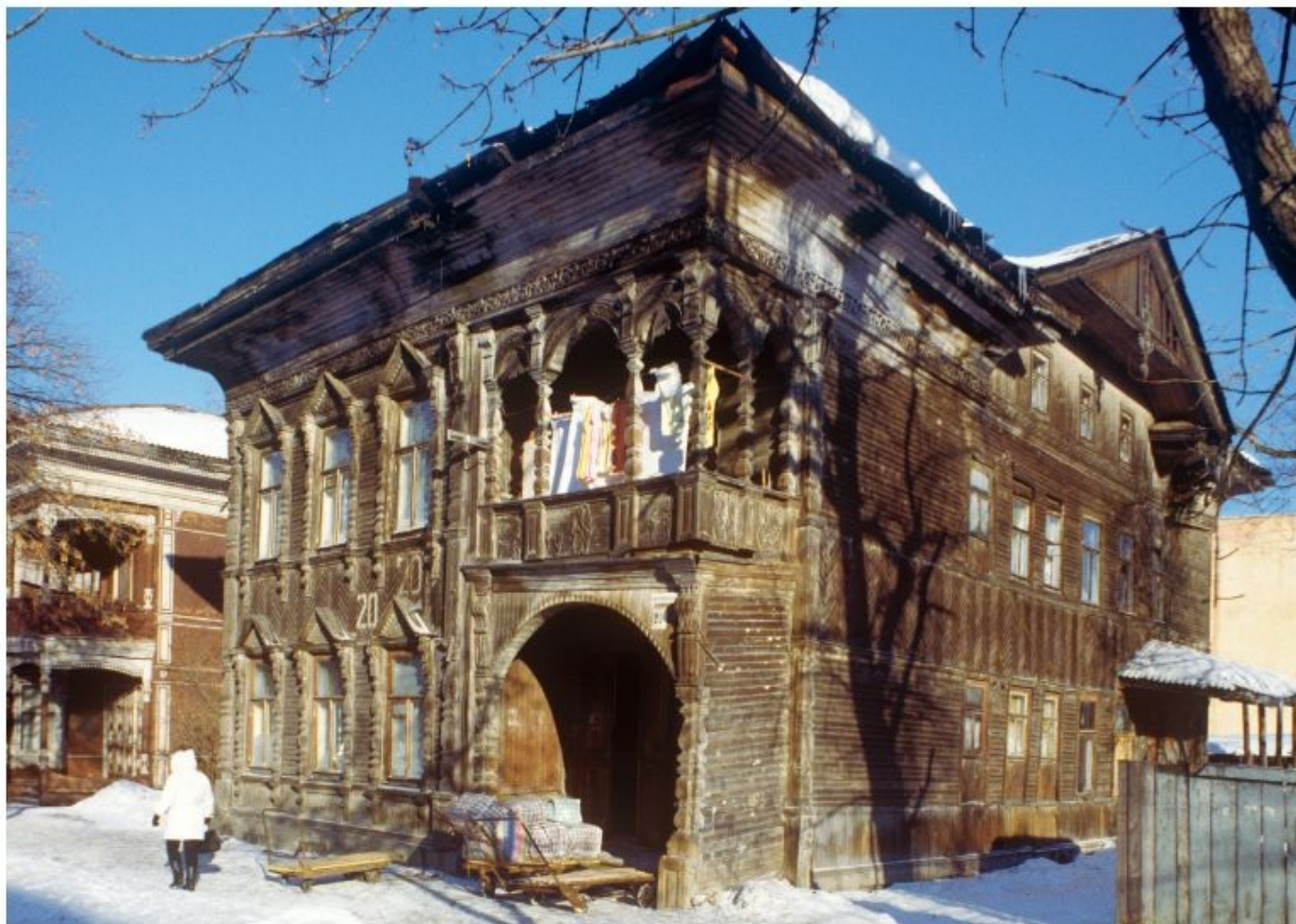
VOLOGDA. Kirkhoglanin house, Annunciation Street 20. Built at the turn of the twentieth century, this house displays the exuberant decoration typical of merchant houses. Photograph: February 26, 1998.
