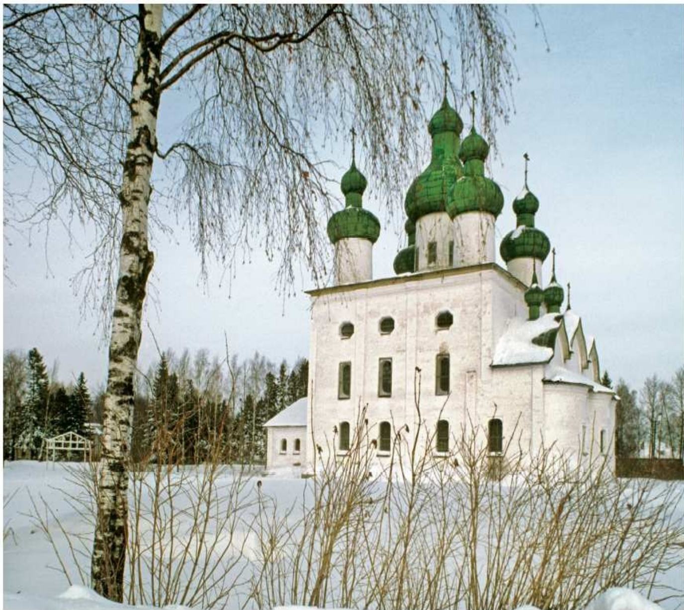
KARGOPOL. Church of the Nativity of John the Baptist, southeast view. Church built in 1751. Photograph: February 27, 1998.
