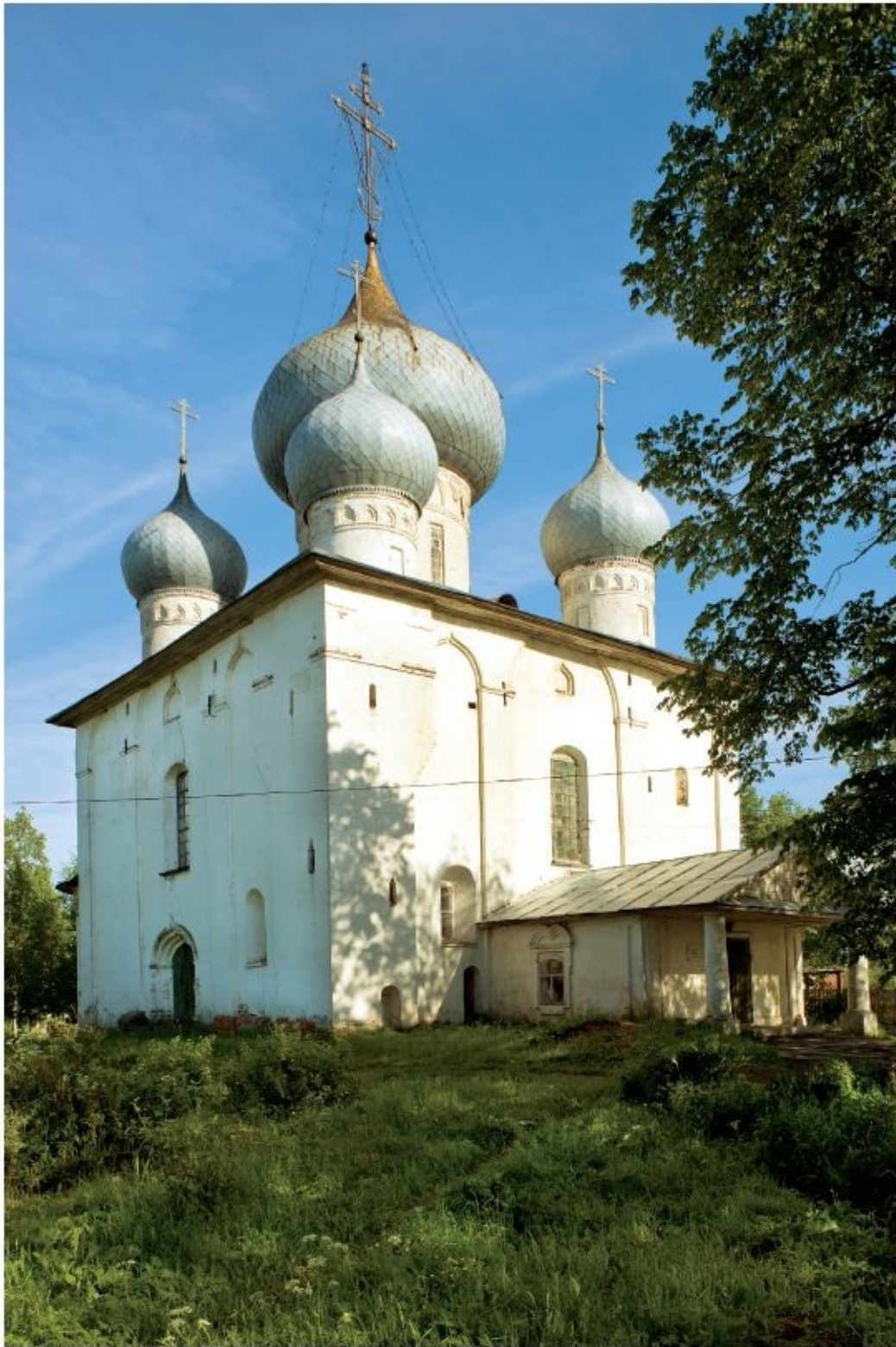
BELOZERSK. Church of the Dormition, northwest view. Also referred to as a cathedral, the structure was built between 1552 and 1563. Photograph: June 9, 2010.
