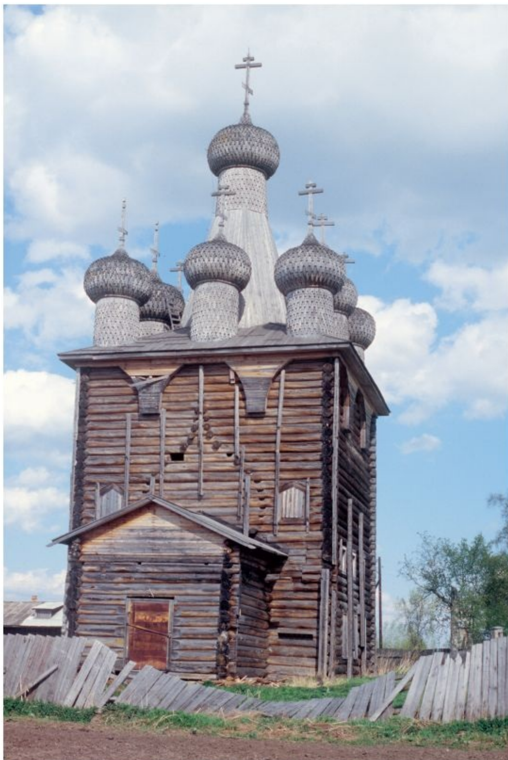
ZAOSTROVYE. Wooden Church of the Purification (also known as Intercession). Built between 1683 and 1688. West view. Photograph: June 10, 1998.
