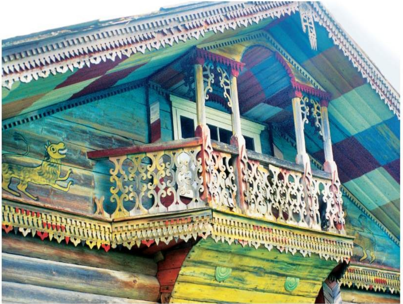
OSTROVSKOE. "House of Lions." Facade with painted eaves, balcony, and ornamental gable. Built in late nineteenth century. Note decorative use of tops from large cans of sardines under the balcony. Photograph: June 13, 2000.
