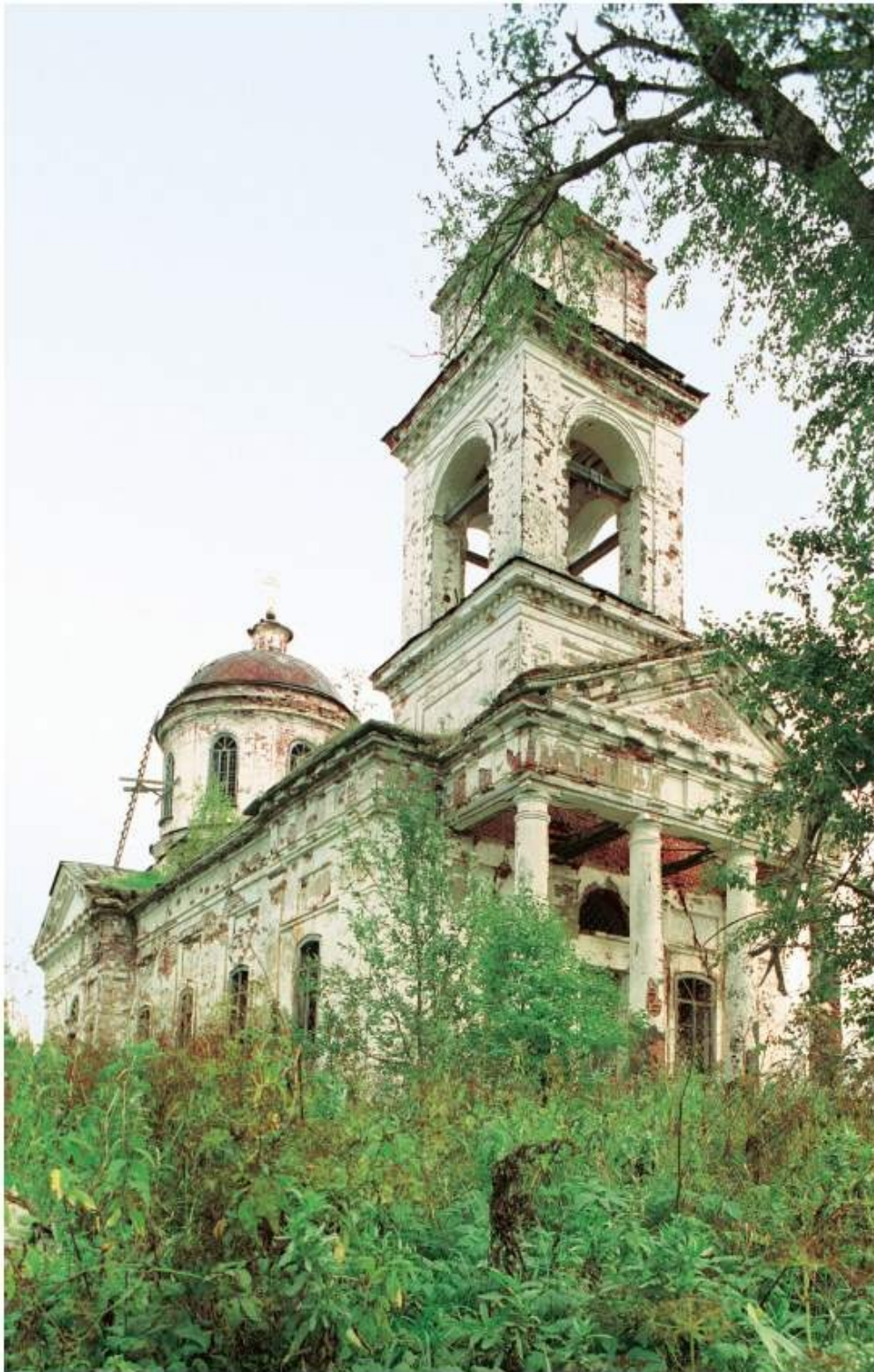
PALTOGA (Paltozhsky Pogost). Church of the Icon of the Sign, northwest view. Church built in 1810. Photograph: August 28, 2006.
