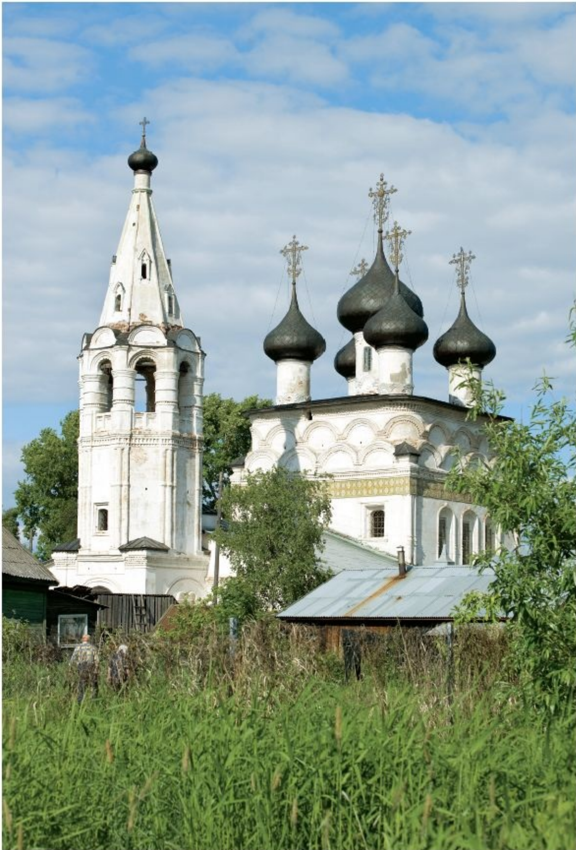
BELOZERSK. Church of the Merciful Savior, southwest view. Church built in 1723. Photograph: June 9, 2010.
