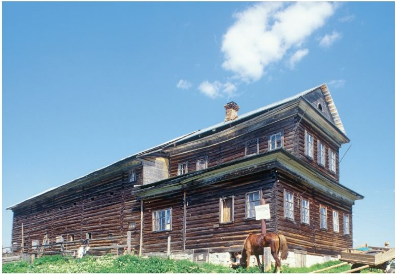
MONASTYR. Log house with attached barn. Photograph: June 23, 1999.
