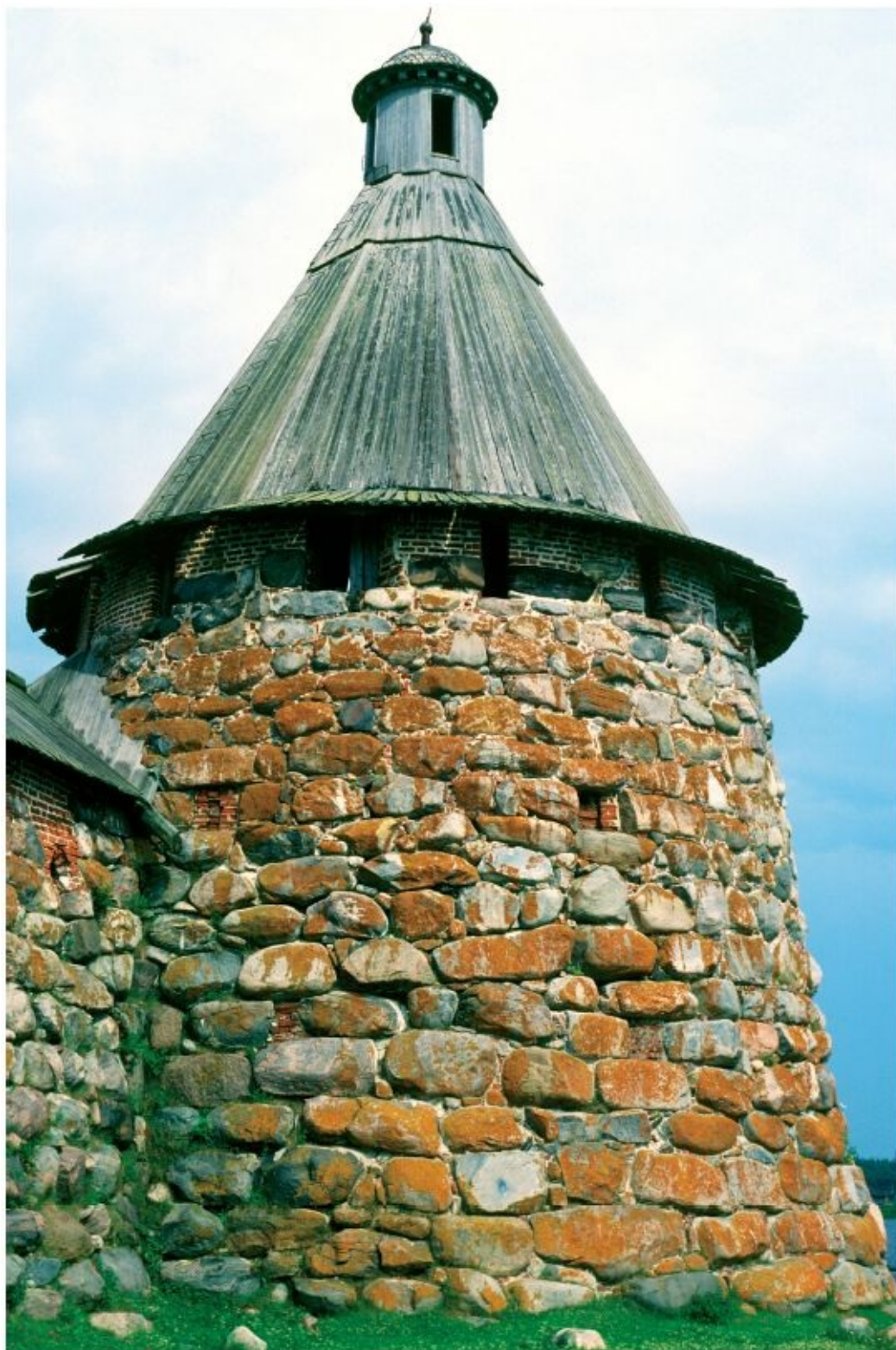
GREAT SOLOVETSKY ISLAND. Archangel Tower, southeast range of monastery walls, built in late sixteenth century from granite boulders. Photograph: July 26, 1998.
