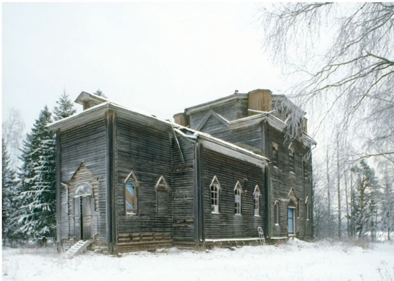
LOVZANGA. Wooden Church of St. Nicholas, southwest view. Church built in 1661. Photograph: November 26, 1999.
