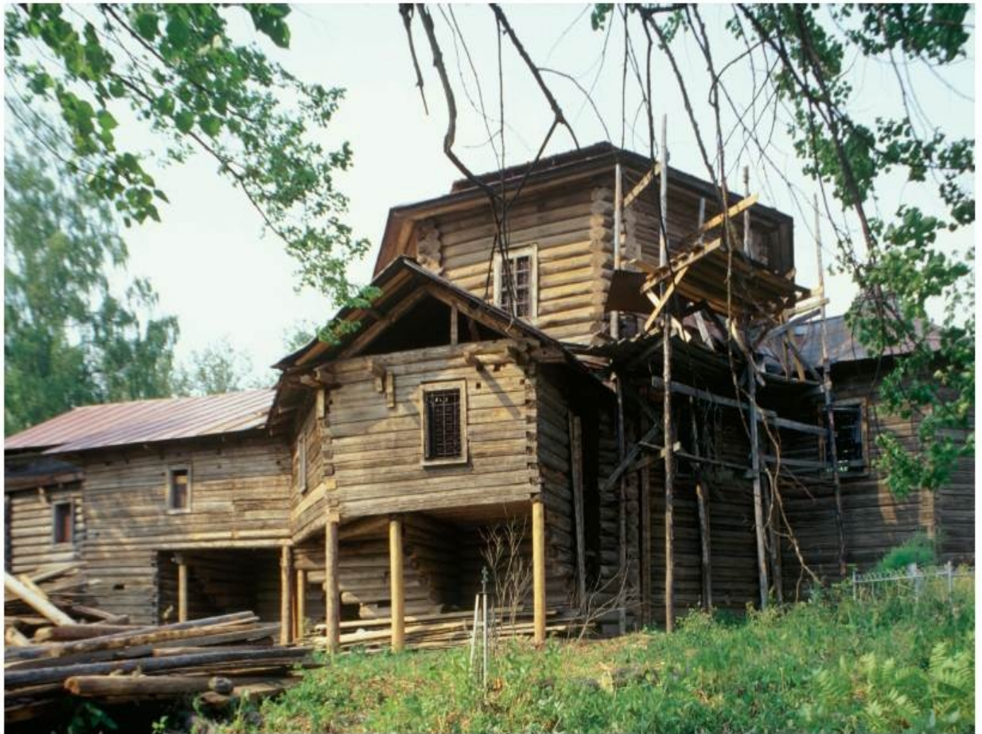
TSYPINO. Wooden Church of Elijah the Prophet. Built in mid-eighteenth century, the upper part of the abandoned church collapsed in the 1960s. This south view shows the structure as the plot was being cleared for a possible restoration, which began in 2003. Photograph: July 15, 1999.
