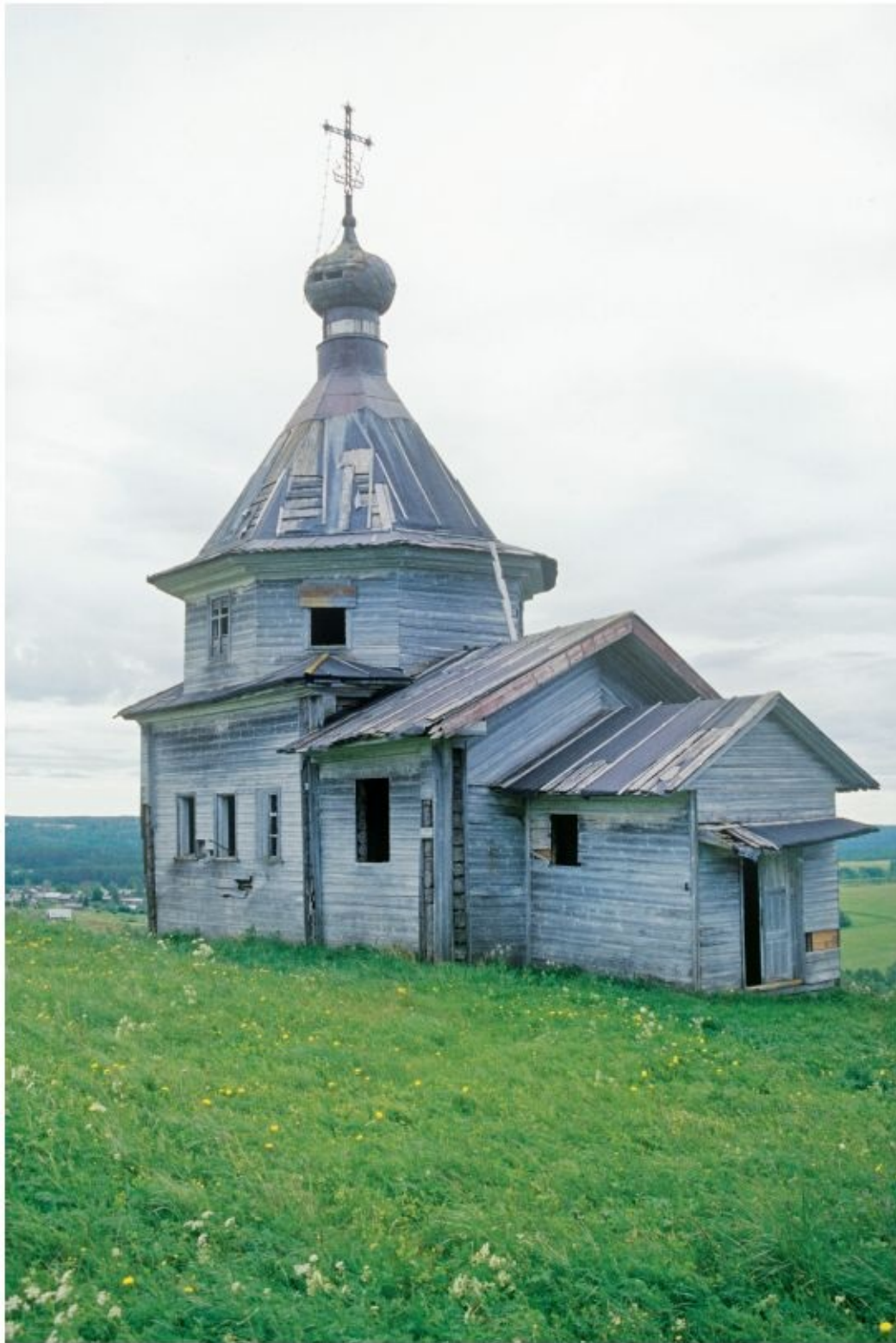
SEREDNIAIA (Yakovlevskaia). Chapel of Saints Zosima and Savvaty, northwest view. Chapel built in late eighteenth or early nineteenth century. Photograph: June 14, 2000.
