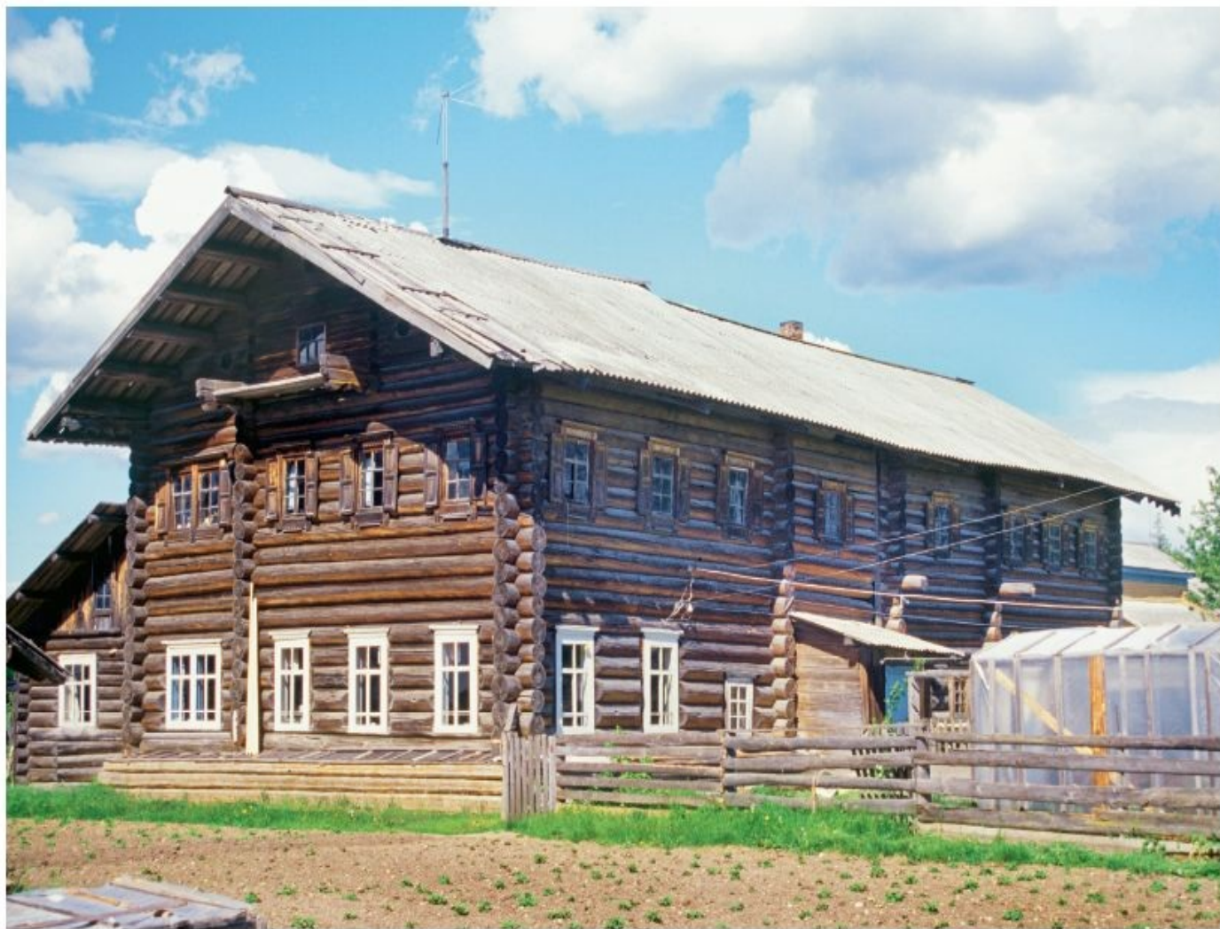
BEREZNYK. Log house (kurnaya izba), river facade. Photograph: June 17, 2000.
