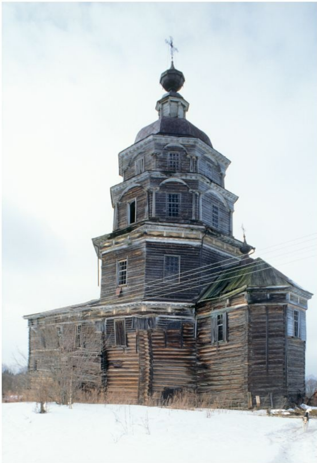
ПОПОВКА-КАЛИКИНСКАЯ. Church of the Nativity of the Virgin, southeast view. Built in 1783. Already with a visible lean, the church collapsed in 2002. Photograph: April 2, 2001.
