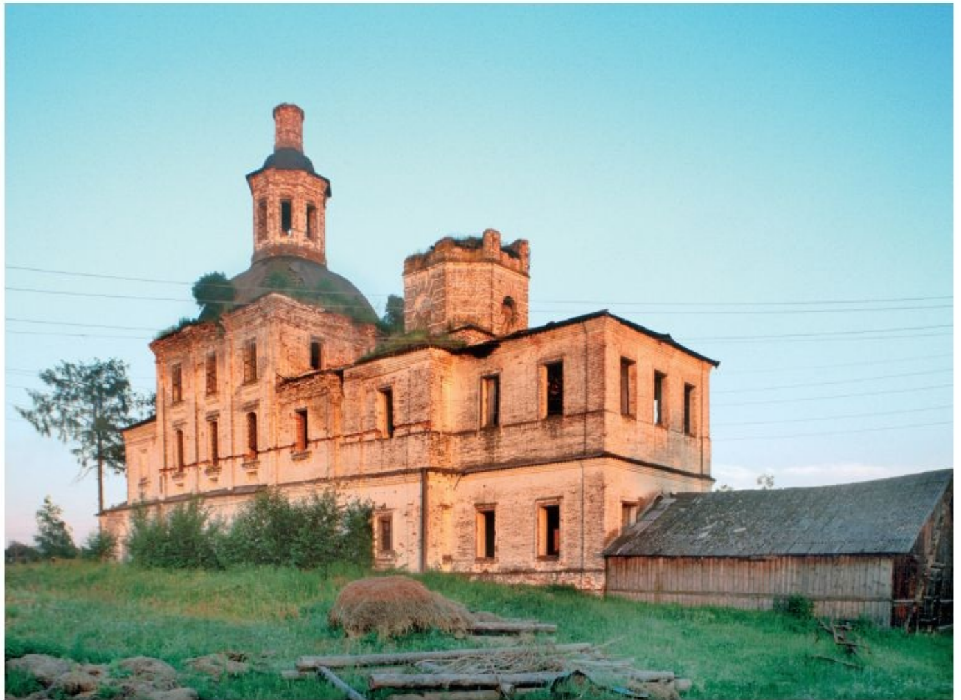
PESCHANITSA (Grigorovo). Church of the Trinity, northwest view at sunset. Built in 1789; upper part of the church collapsed around 2010. Photograph: June 25, 2000.
