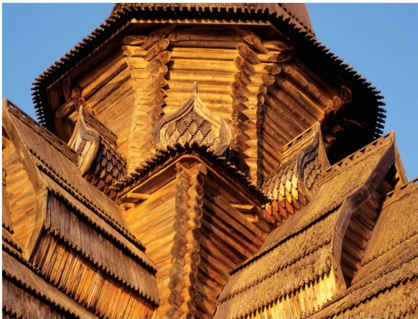
VARZUGA. Church of the Dormition, northwest view, upper structure. Construction details no longer visible because of new plank siding. Photograph: July 20, 2001.
