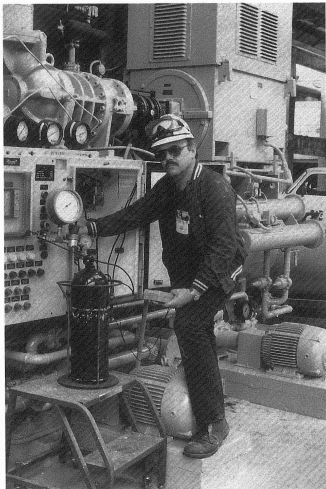
Figure 20 Proof testing a high-pressure switch on a refrigeration unit.
