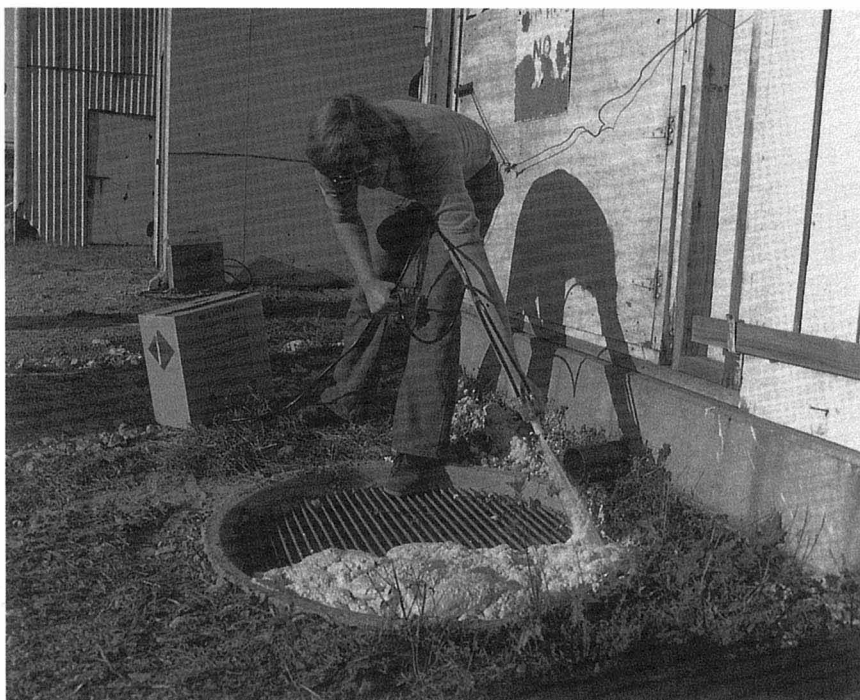
Figure 2 Sealing a sewer grate with a urethane foam unit.
