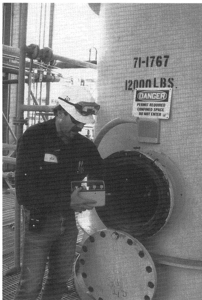
Figure 5 An operations foreman checks for blinding and samples the vessel's atmosphere before tank entry.
