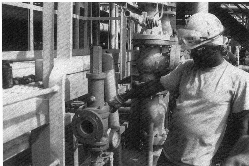
Figure 17 A mechanic is tightening down the bolts as he reinstalls a safety relief valve (SRV) after it was tested in the shop.
