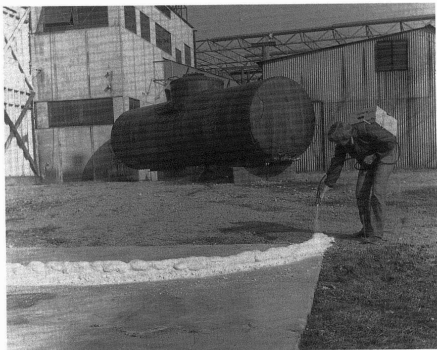
Figure 1 Formation of a dike with a urethane foam unit.
