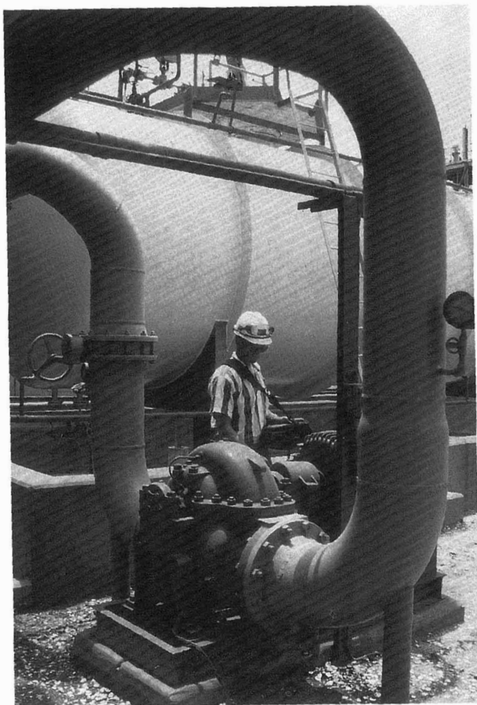
Figure 1 A vibration technician taking readings on a cooling water pump.
