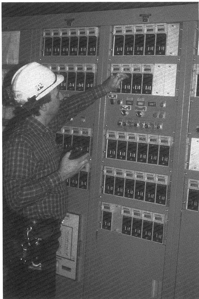
Figure 23 An instrument repairman proof tests a critical instrument panel.
