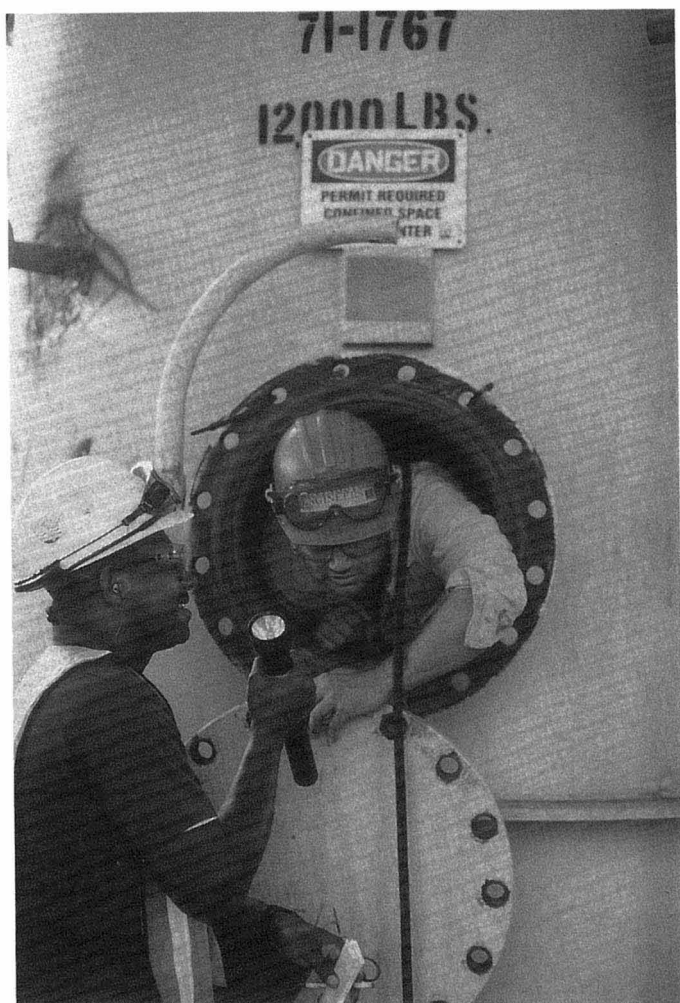
Figure 7 A pressure vessel inspector enters a confined space after the vessel is blinded, tested, and cleared, but he still relies on a manway watchman.
