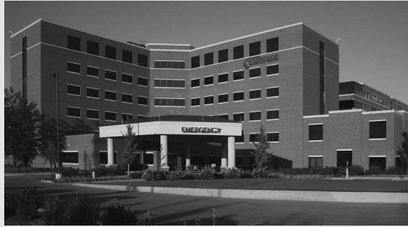
FIGURE 21.8 A new canopy introduces WMC's Emergency Department, which moved into vacated spaces to protect land usage and allow further expansion. (Photo courtesy of Chad Alan. With permission.)
