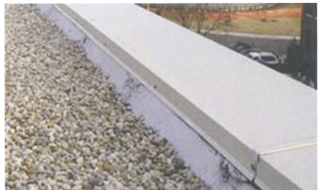
Timber roof with low parapet and layer of shingle
