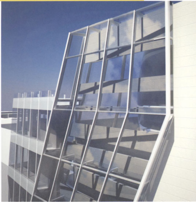
Double skin facade creating a thermal chimney
