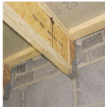
Typical joist hanger in masonry wall with engineered timber joist
