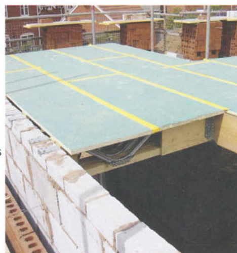
Typical timber floor construction with masonry structure. Timber boarding used for stiffness
