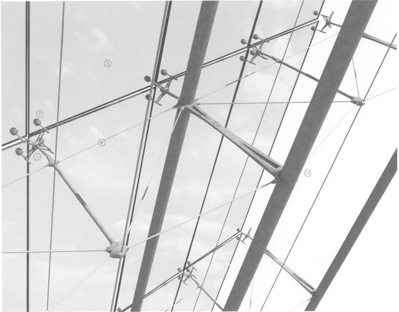
3-D view of bolt fixed wall system
