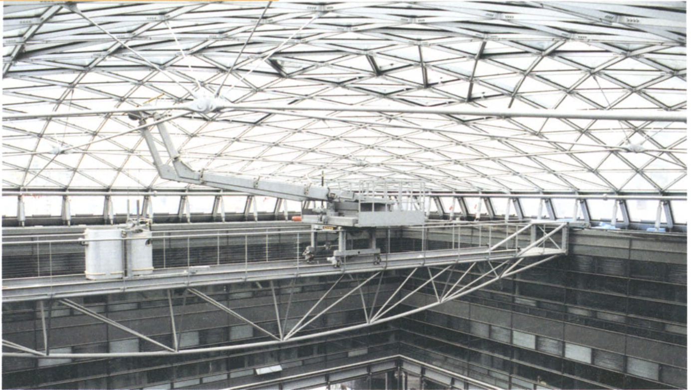
Cleaning gantry allowing underside of roof to be cleaned and maintained without cleaning platform from below. B8 offices , Daimler Chrysler Projekt, Potsdamer Platz, Berlin. Architect: Richard Rogers Partnership.
