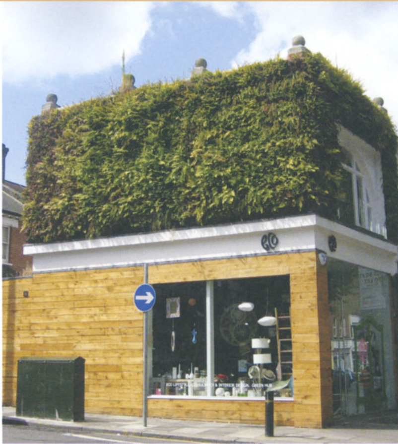
Modular system with soil substrate: Eco Store, London.
