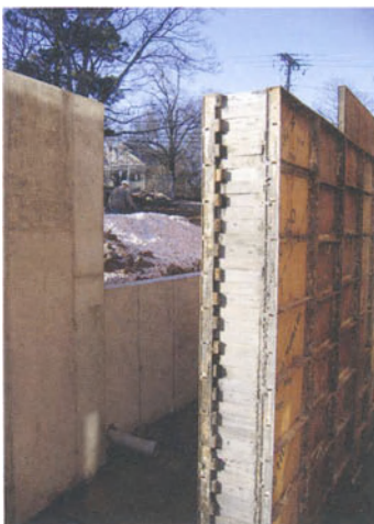
Timber formwork used to achieve decorative texture
