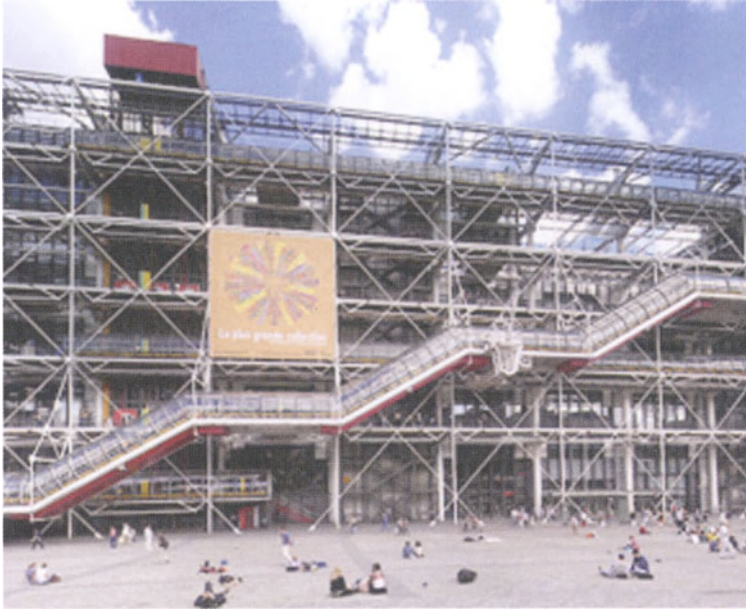
Braced steel frame . Pompidou Centre, Paris, Architects: Richard Rogers
