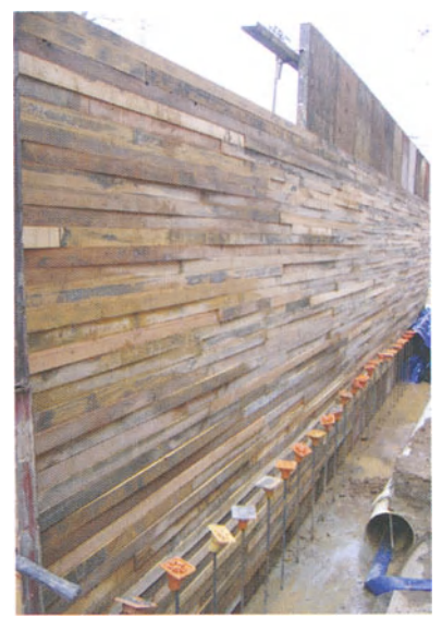
Timber formwork used to achieve texture
