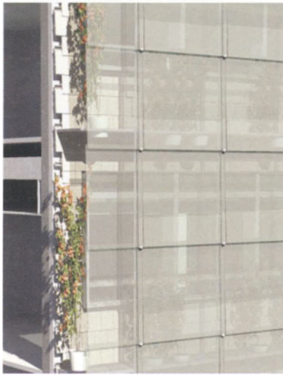
Vertical Section 1:20 and 3-D view through double skinned facade with plant in cavity
