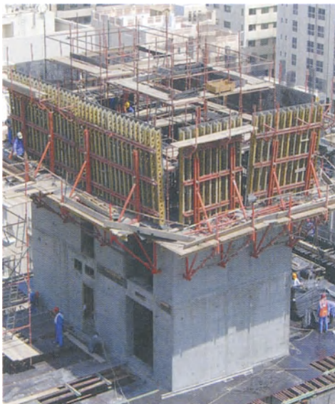
Timber/Aluminium formwork on upper floors of building construction
