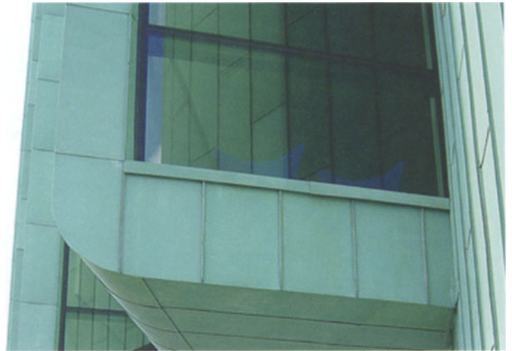
Copper cladding in use
