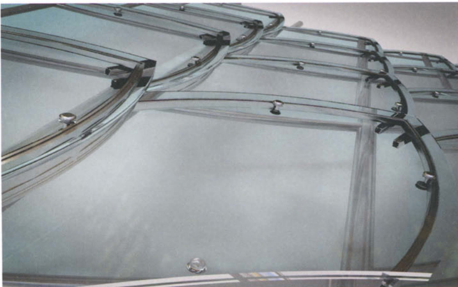
Above. Section showing sealed connection between panels
