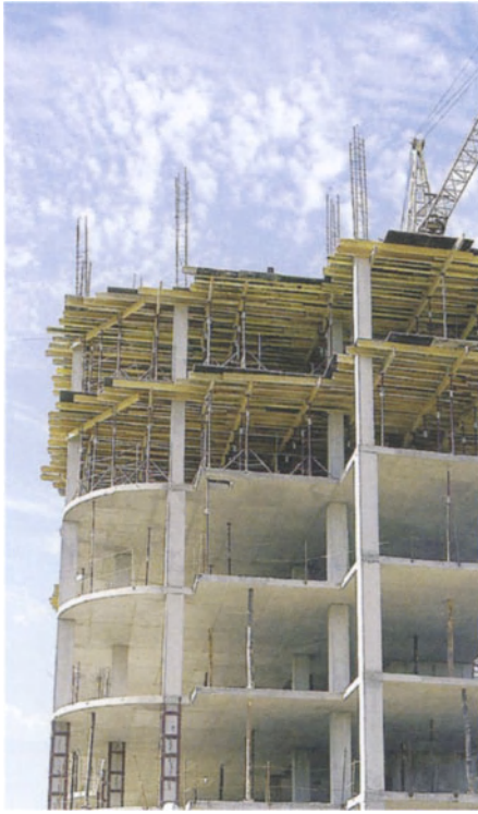
Typical in-situ concrete tower construction showing form work on top two floors
