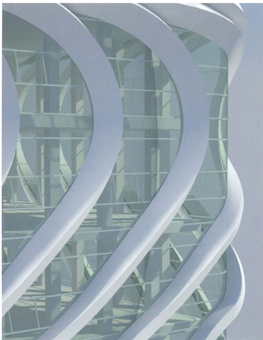
Close-up views of twisting louvres
