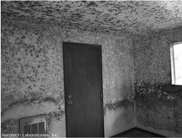
13.1 Bedroom mixture of Cladosporium , Aspergillus , and Penicillium on painted drywall surface.
