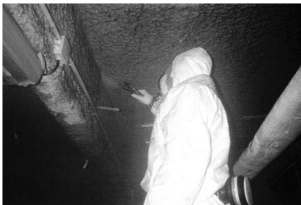
7.7 Worker removing indoor friable asbestos.
