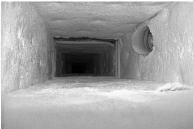
13.7 HVAC duct encapsulant lining.
