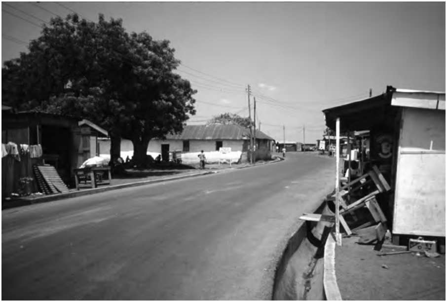
Figure 14.4 The improved road in Agbogba, 2003
