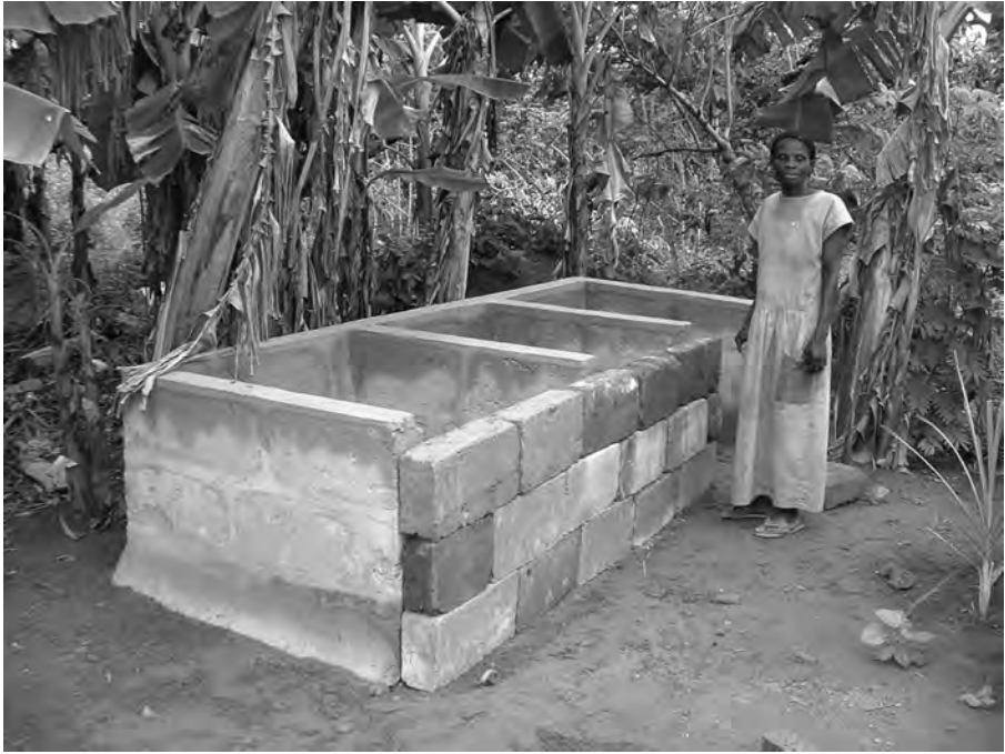
Figure 16.3 High-capacity block-built compost bin
