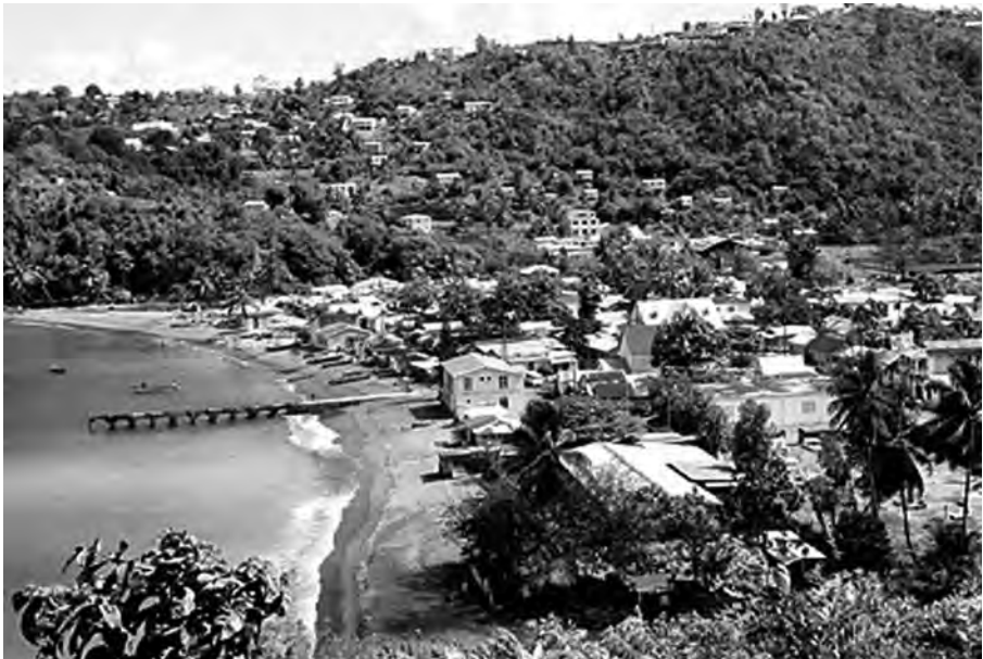
Figure 10.3 Anse La Raye's dilapidated waterfront zone
