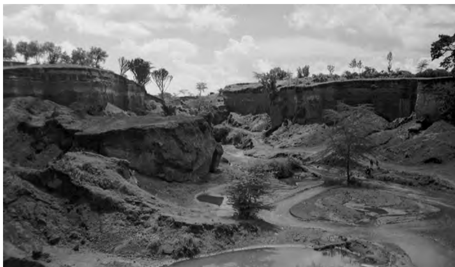
Figure 18.5 Soil erosion and sedimentation in the Njoro River caused by sand extraction
