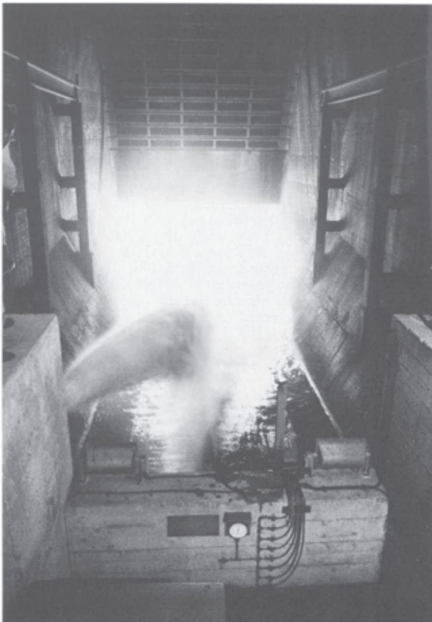
*Plate 6.2* The control of river flows by valves: inside Clywedog Dam, mid-Wales, regulating the flow of the River Severn (photo M.D.Newson)
