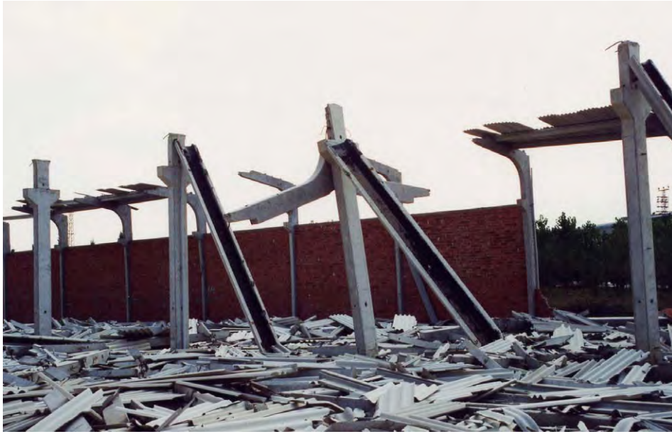
Fig. 2-14: Failure of cantilever head connection on top of columns (1999 Kocaeli earthquake)
