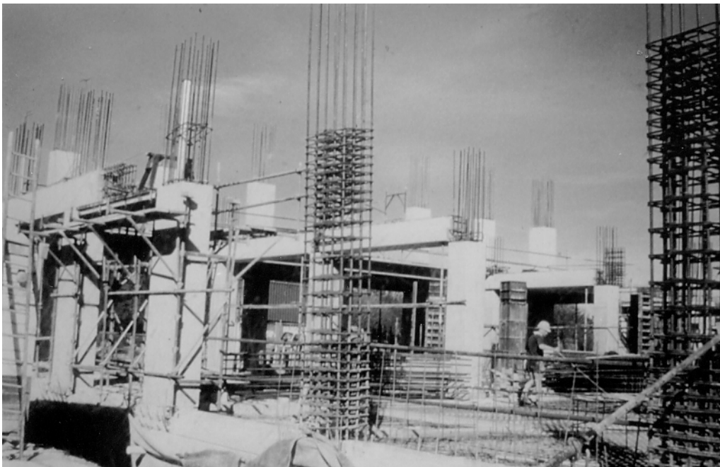
Fig. 4-14 Construction in New Zealand of an equivalent-monolithic moment frame using precast beams and cast-in-place columns, showing column tie reinforcement
