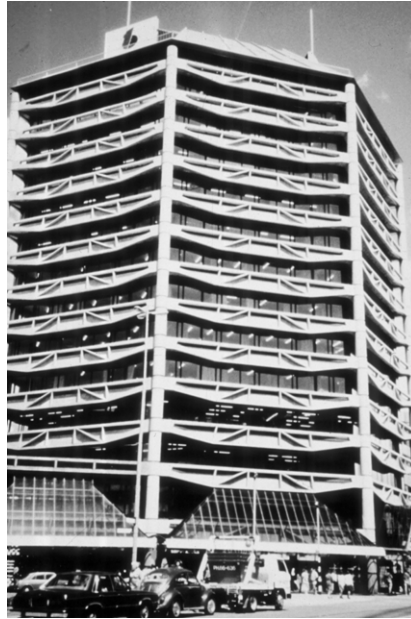
Fig 5-69 Precast concrete perimeter frame in a building in New Zealand with seismic forces resisted mainly by an interior core of cast-in-place concrete structural walls (Courtesy of R. Park)
