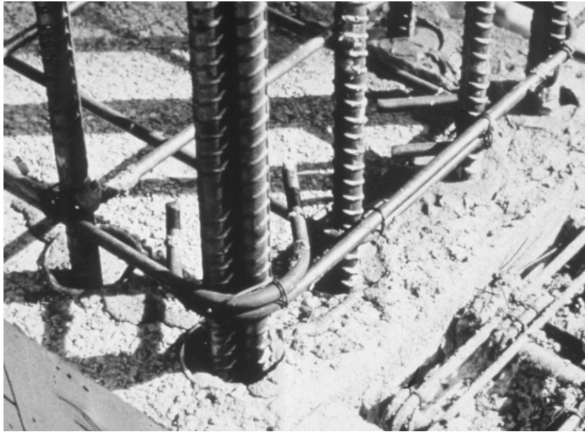
Fig. 5-12: Column bars after being grouted in the joint core (Courtesy of J. Restrepo)
