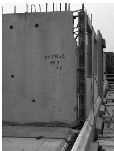
Fig. 5-48: Wall panel connection detail in large panel construction (Courtesy of M. Fischinger)
