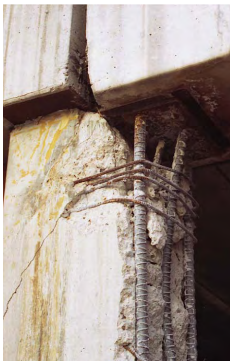
Fig 2-18: Failure of beam-column pin connection at top of poorly detailed column (1994 Northridge earthquake)
