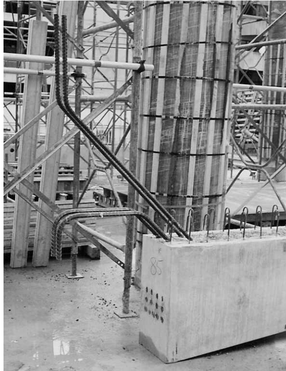
Fig. 5-37: Example of the end reinforcement of a precast prestressed secondary beam with a pinned joint in a construction site in New Zealand (Courtesy of J. Restrepo)
