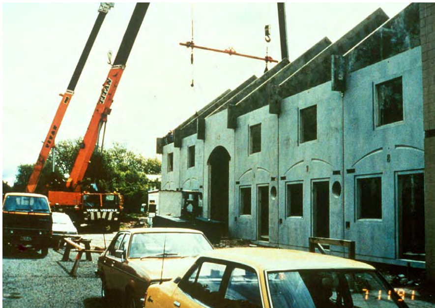
Fig. 3-6: Wall panels with discrete joints and ductile connectors
