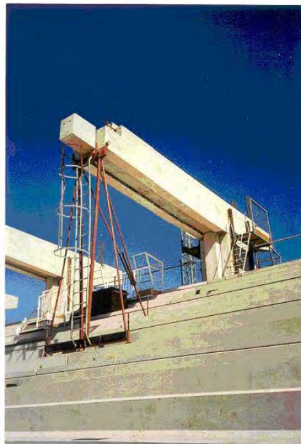
Fig. 3-7: Temporary support with access ladders and work platforms for grouted post-tensioned joints
