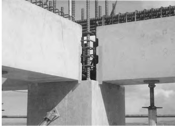
(a) Example from Japan: View of beams before the placement of the floor slab (Courtesy of F. Watanabe)
