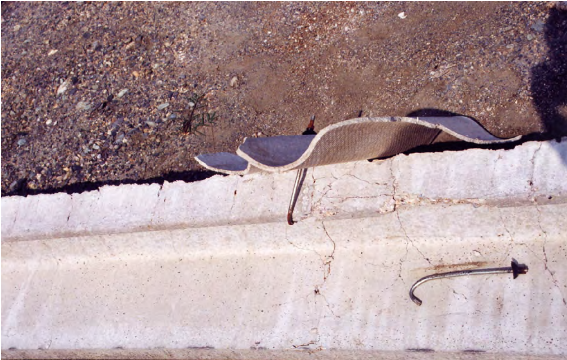
Fig. 2-10: Flexible connections connecting diaphragm to precast concrete beam (1999 Kocaeli earthquake)
