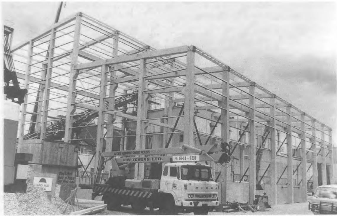
Fig 3-3: Precast, pre-tensioned columns and rafter (Caxton Paper Mill, Kawerau)
