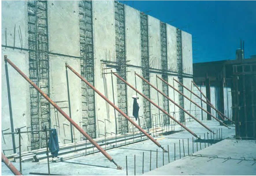
Fig. 3-5: Lapped reinforcing bars in wall joints, emulating cast-in-place construction.
