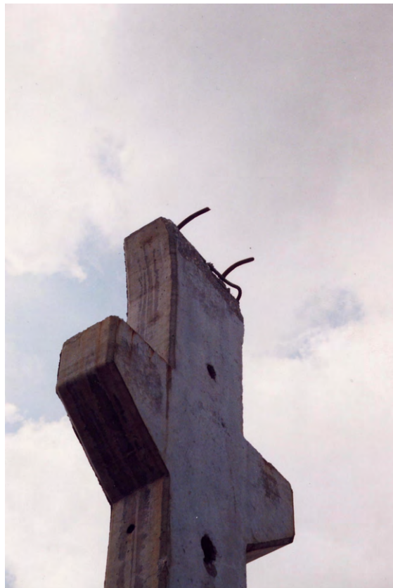
Fig. 2-15: Failure of column to cantilever head connection due to failure of bolts (1999 Kocaeli earthquake)
