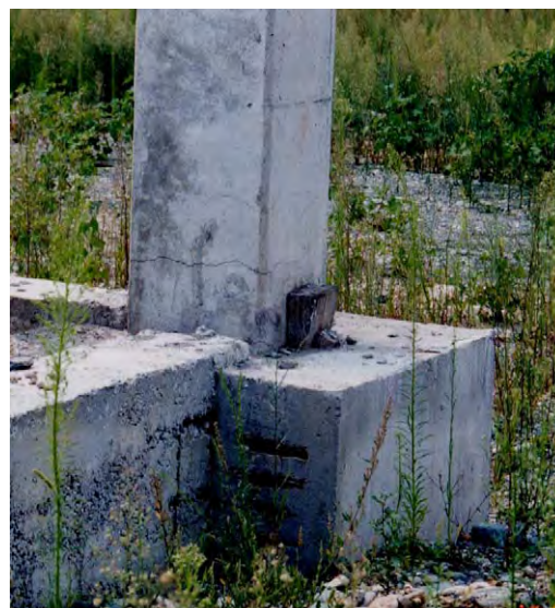
Fig. 8-4: Undamaged socket foundation (Kocaeli earthquake, Turkey 1999)
