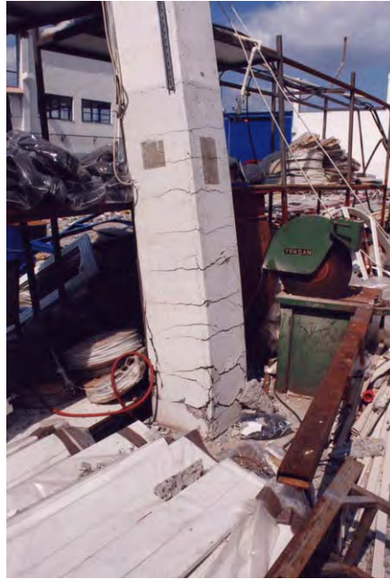
Fig. 2-6: Flexural hinging at base of precast concrete column (1999 Kocaeli earthquake)
