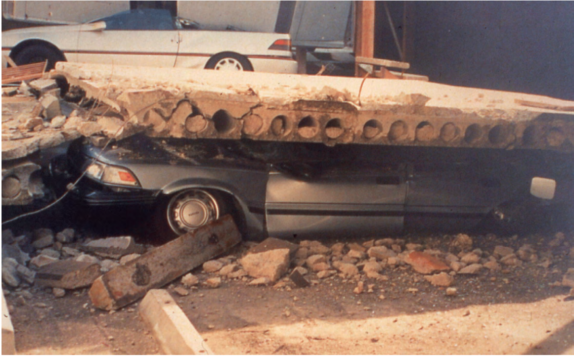
Fig. 2-9: Collapse of precast concrete hollow core floor (1994 Northridge earthquake)
