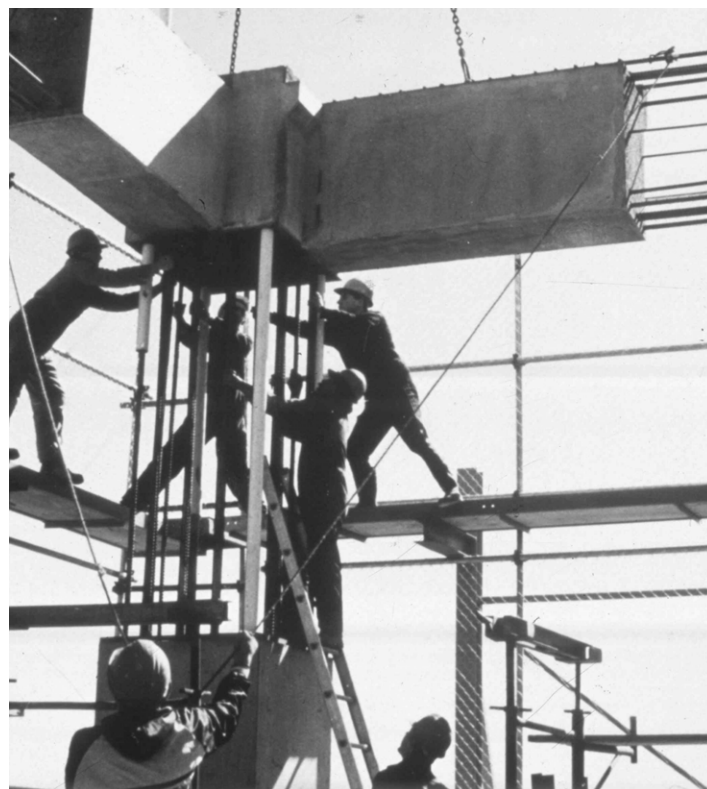
Fig. 5-11: Beam corner unit being lowered into place using temporary plastic tubes as guides (Courtesy of J. Restrepo)
