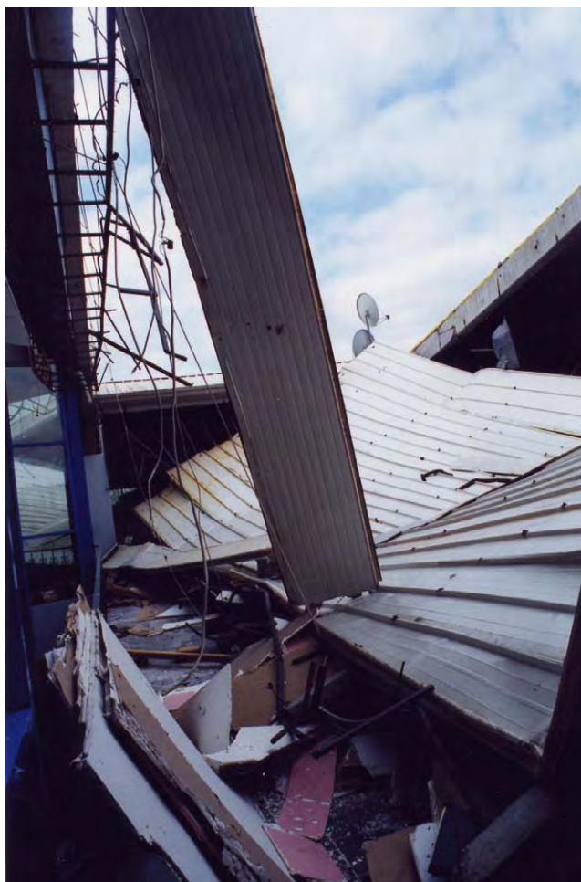
Fig. 2-11: Failure of flexible light-gauge metal diaphragm (1999 Kocaeli earthquake)
