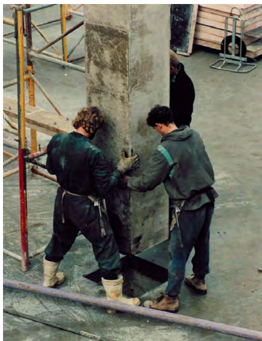
Fig. 8-1: Application of the socket base connection in New Zealand (Courtesy of J Restrepo)
