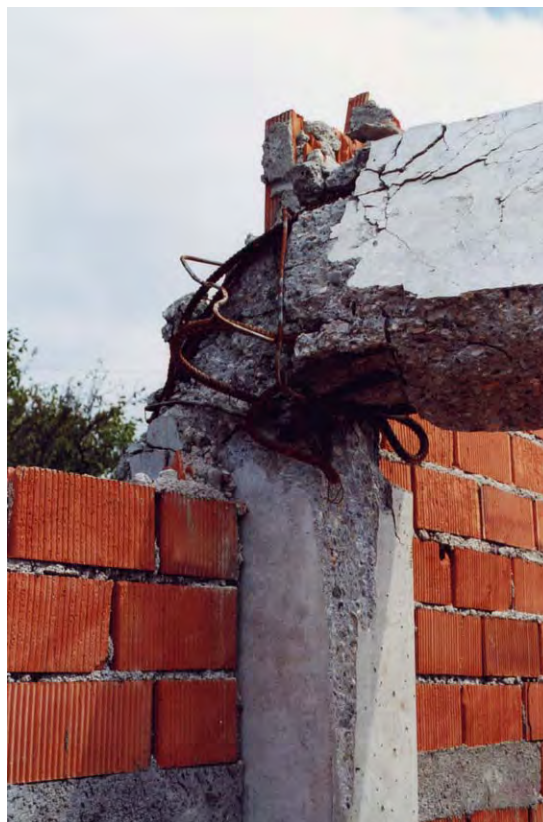
Fig. 2-20: Failure of column at lap splice connection and at top of infill wall (1999 Kocaeli earthquake)
