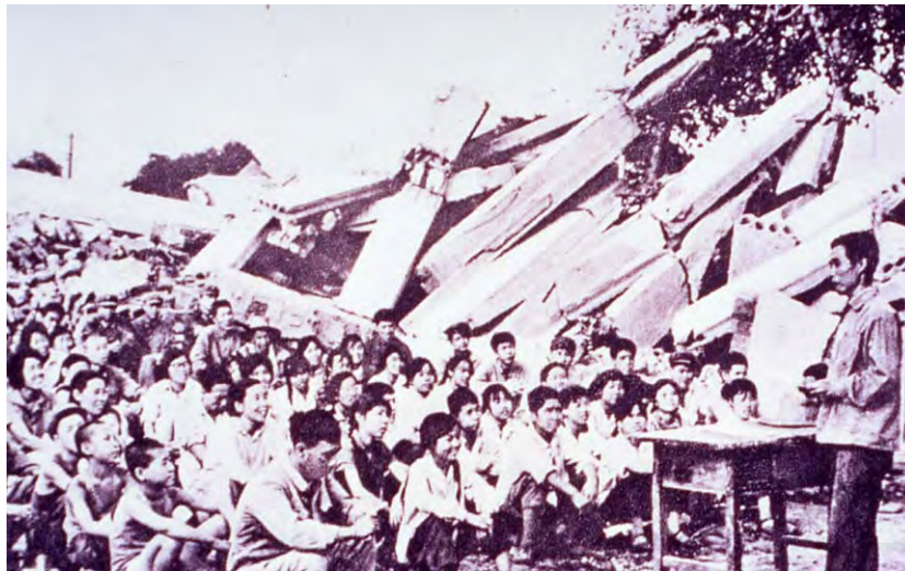
Fig. 2-1: Collapse of precast buildings in Tangshan, China in 1976
