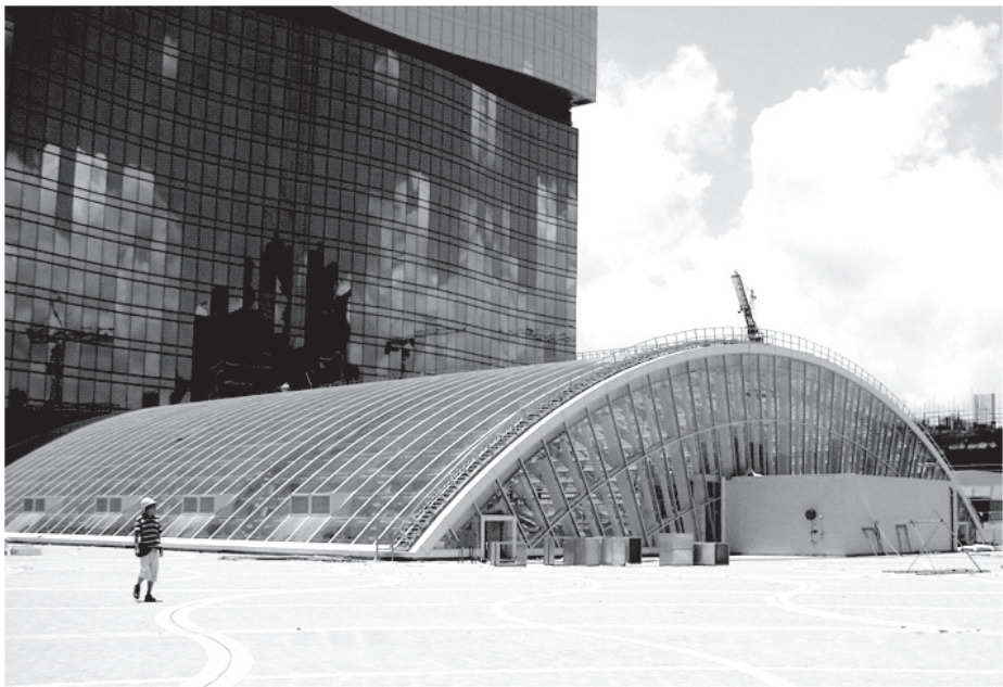
FIGURE 7.5 The single-layered shallow roof of a building (as built).
