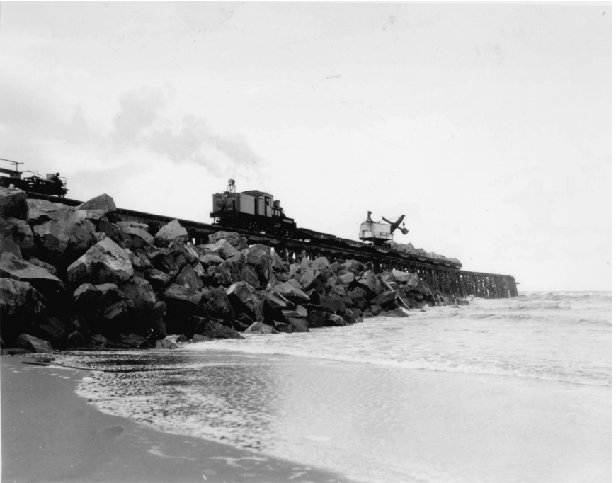
FIGURE 18-2. Trestle Construction Method (COE, Portland District).
