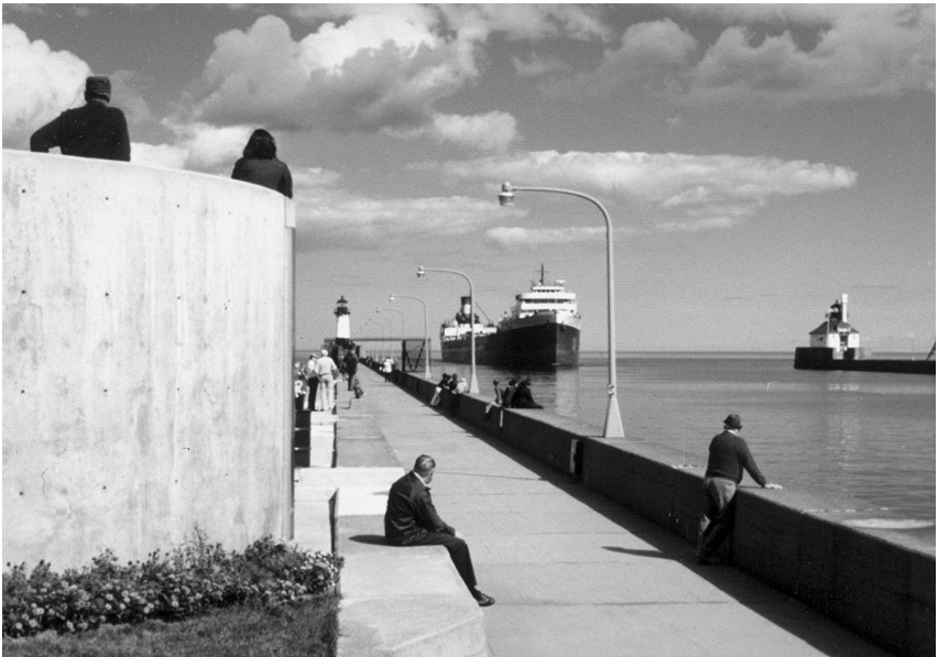
FIGURE 11-7. Concrete Composite Jetty at Duluth Harbor (COE, Digital Visual Library).
