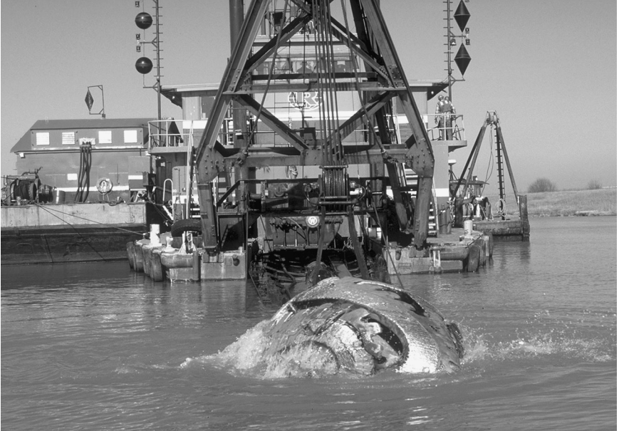
FIGURE 10-5. Dredging Sacramento Ship Channel (COE, Digital Visual Library).
