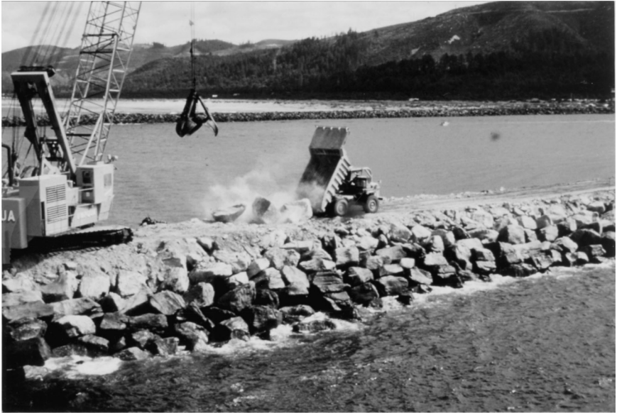
FIGURE 11-3. Armor Rock for Yaquina Jetty Repair Work (COE, Portland District).
