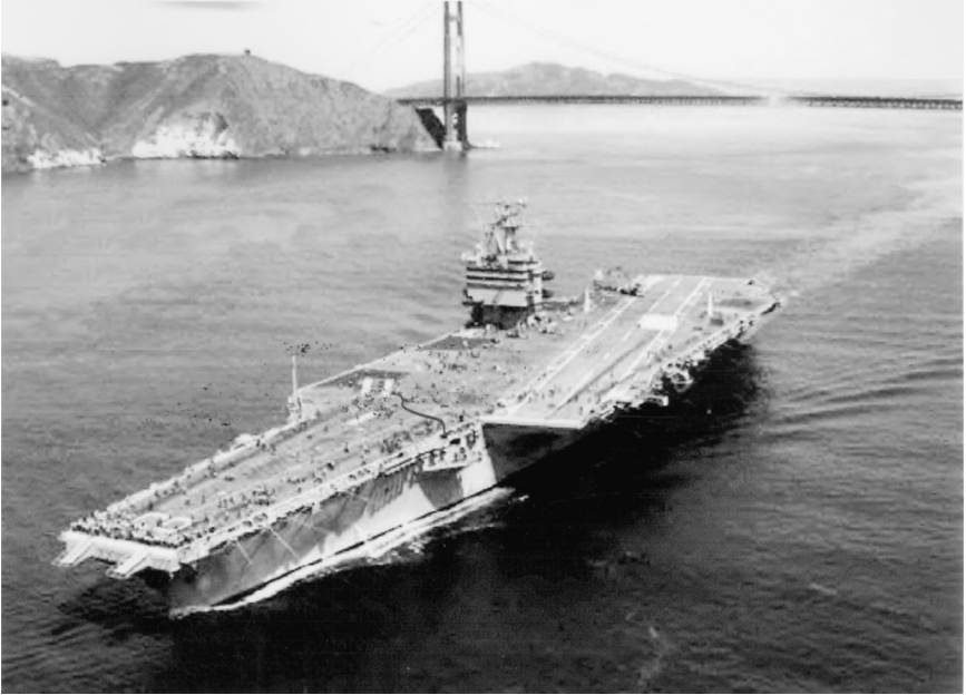
FIGURE 13-4. Golden Gate Bridge Provides Generous Clearance For Ships [USS Enterprise (Navy Web, chinfo.navy.mil )].
