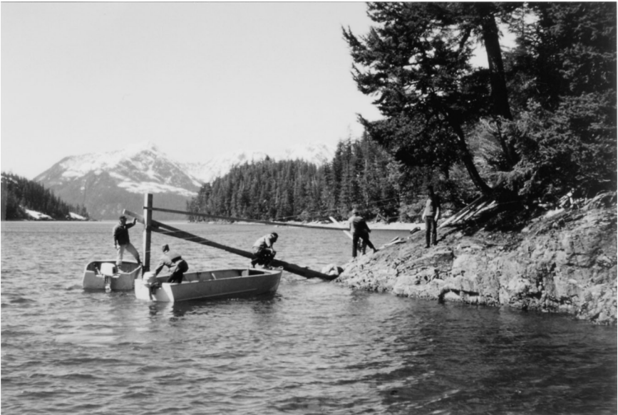
FIGURE 21-3. Temporary Tide Gauge, Prince William Sound, Alaska (from Lieutenant (jg) B. McCartney).
