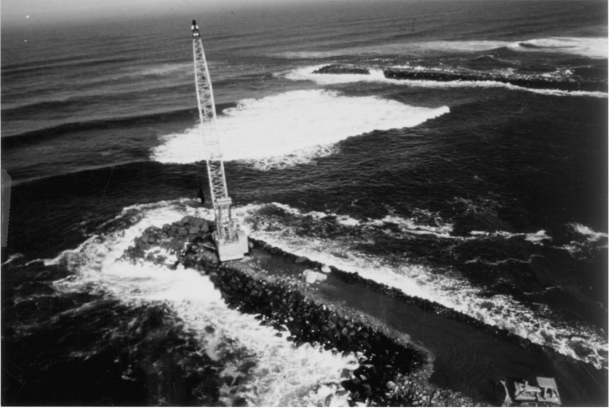
FIGURE 18-1. Yaquina Bay Jetty Rehab (COE, Portland District).
