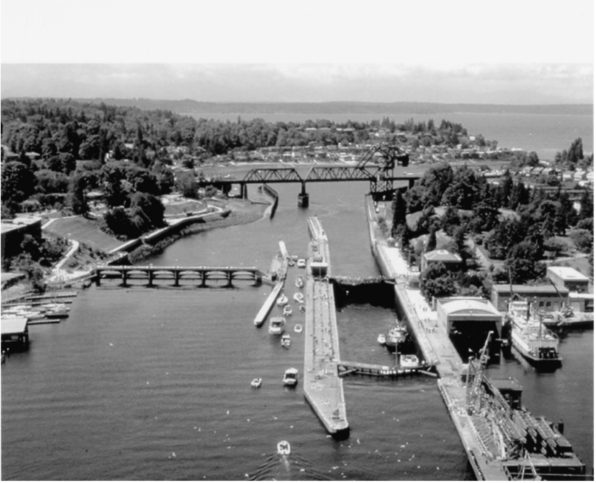
FIGURE 12-3. Hiram M. Chittenden Locks, Seattle, Washington; Large Lock for Ships, Small Lock for Pleasure Craft (COE Seattle District).
