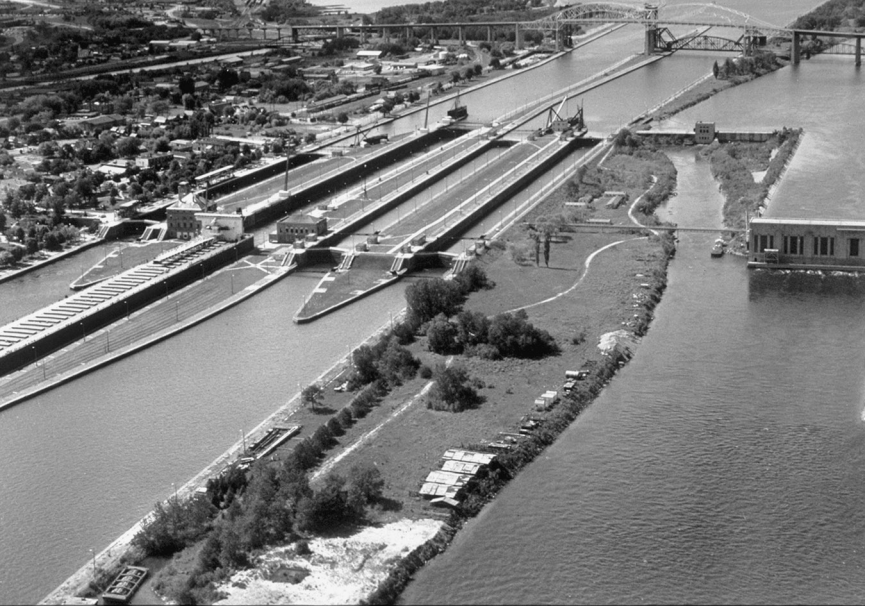
FIGURE 12-1. Soo Locks at Sault St. Marie, Michigan; Ship Departing from Poe Lock (COE, Digital Visual Library).
