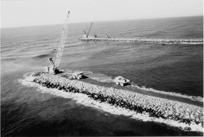
FIGURE 19-1. Yaquina Bay, Oregon Jetty Repair (COE, Portland District).
