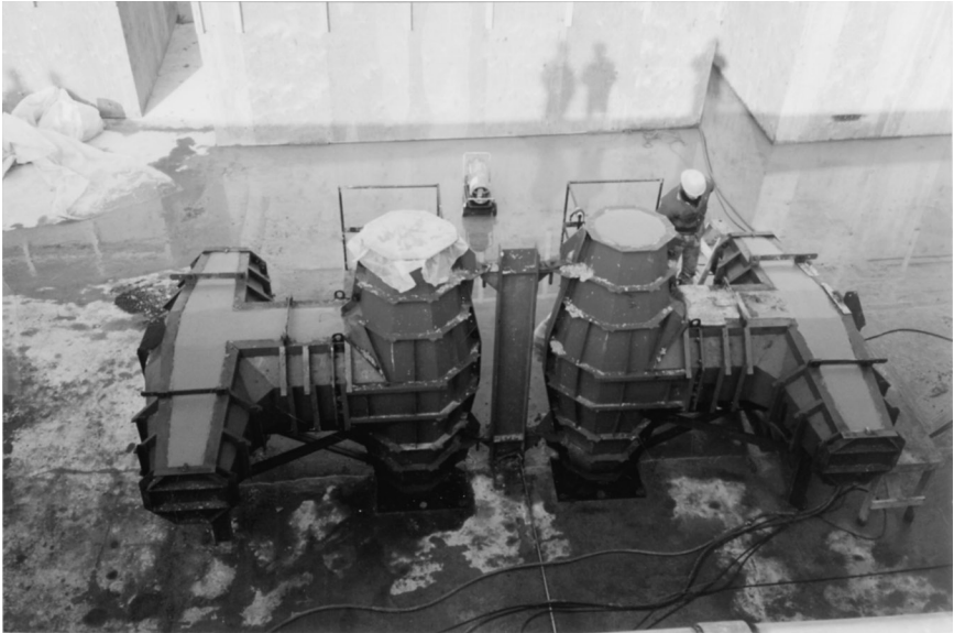
FIGURE 11-5. Dolos Armor Units Cast in Tacoma, Washington (COE, North Pacific Division).
