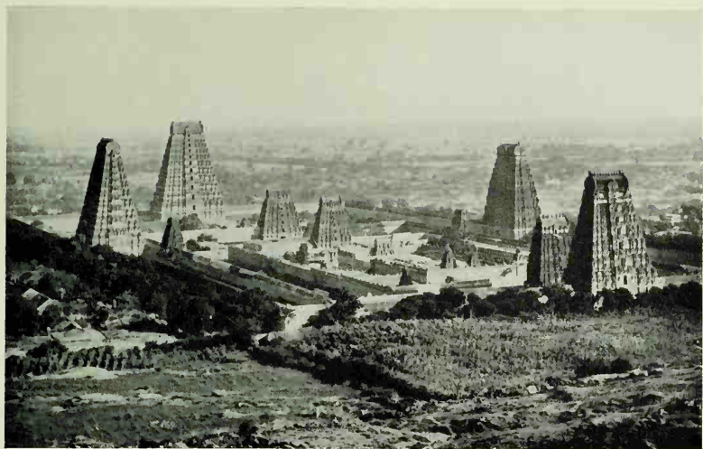
(A) Temple at Tiruvannāmalai
