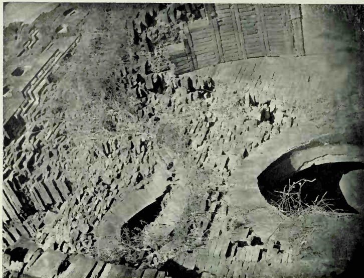
(B) Vaults of Mahābodhi temple before restoration
