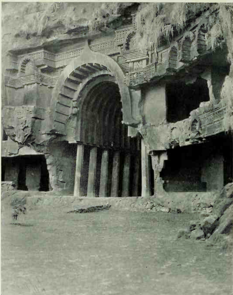
Façade of chaitya-hall. Bhājā
