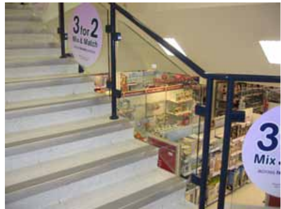
Glazed guarding on this staircase in a shop allows customers to see products on the floor below. Note the visually contrasting nosings, handrails and guarding supports
