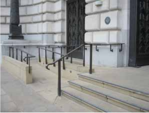
A ramp utilising the space to the side of these steps provides step-free access to the main entrance of this office building without intruding on the pavement
