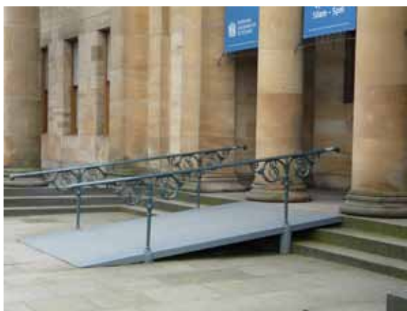
Some temporary ramps, designed in keeping with the building, become permanent
