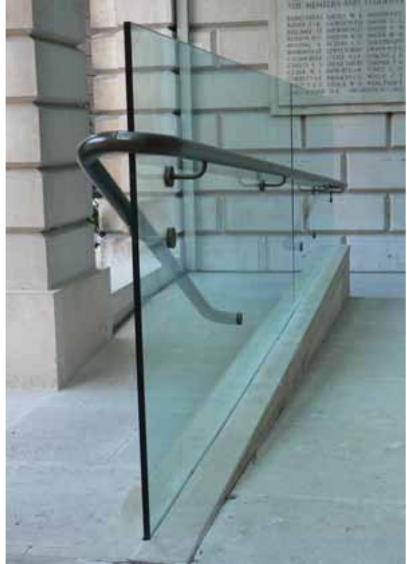
The central glass balustrade to this dogleg ramp provides support for the handrail and has minimum impact on the appearance of the building
