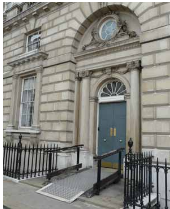
An inelegant temporary ramp to a listed office building that projects out into the pavement, providing a potential trip hazard
