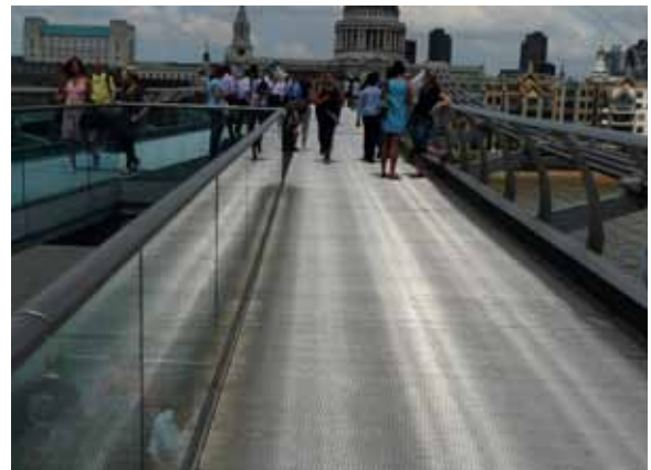
Glare from bright sunlight on this external metal ramp may be difficult or confusing, particularly for people with visual impairments
