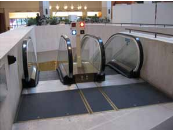
The direction of travel of these escalators in a public building is clearly signed and easily visible
