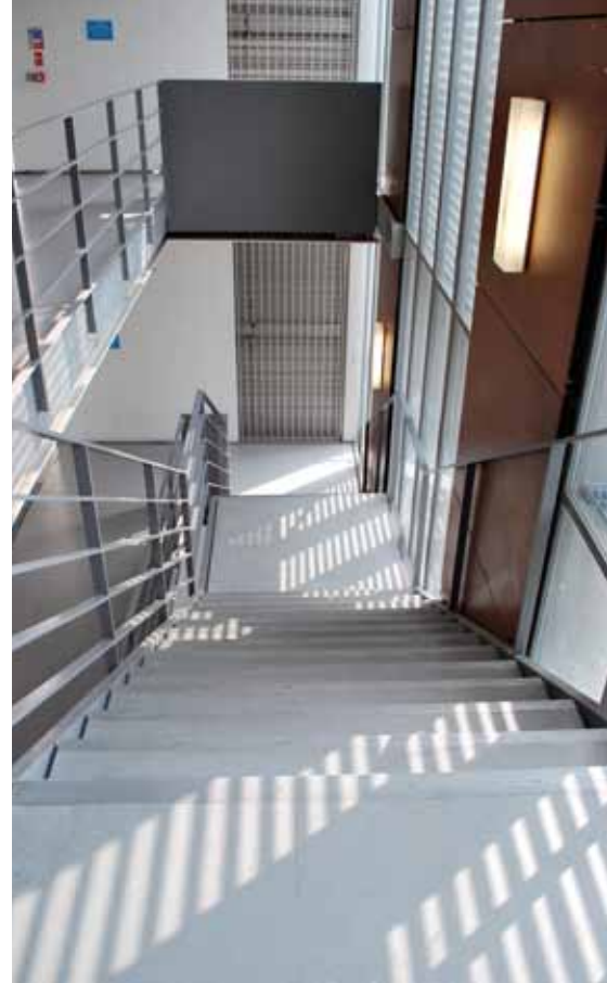
Shadows caused by bright sunlight through the Venetian blinds obscure these stairs, which do not have visually contrasting nosings, and may confuse people with visual impairments
