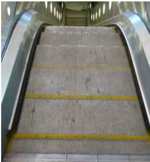
Flat steps at the top of an escalator are required to facilitate people getting on or off a moving surface. Note the yellow line marking the front of the treads and the side lighting set into the balustrades, which helps to highlight the step edges
