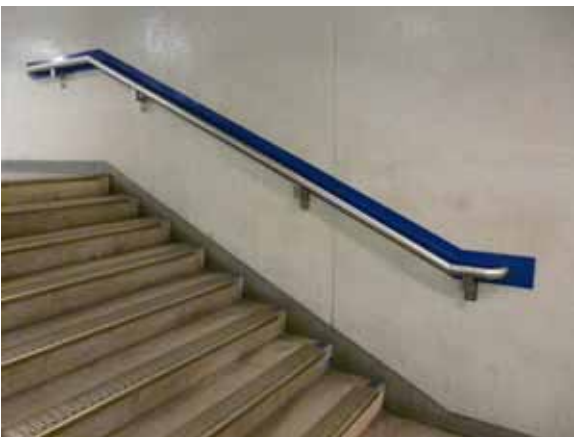
A blue band has been put behind this handrail in a London Underground station to provide greater visual contrast
