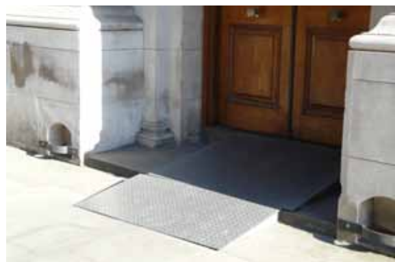
This temporary ramp to an office building is in two parts to accommodate two steps with different height risers. The two parts of the ramp may not stay together or aligned and the projection into the pavement could cause a trip hazard for pedestrians
