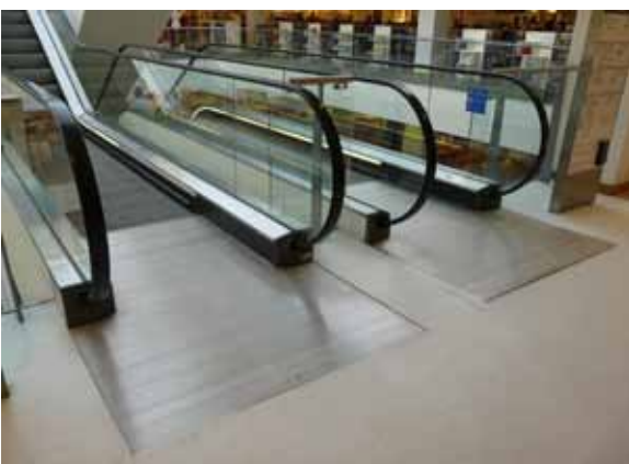
A spacious landing at the top and bottom of escalators minimises the risk of congestion and blocked egress. Note the extended landing plates and moving handrails, which help to mitigate conflict between people moving directly to the next escalator and those wanting to access or leave that floor level
