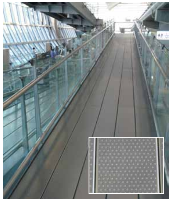
An internal profiled metal ramp in an airport gives a light appearance and is hard wearing and easy to clean. Note that the guarding is higher than the handrails and that the lower rail provides protection to the glass and a tapping rail
