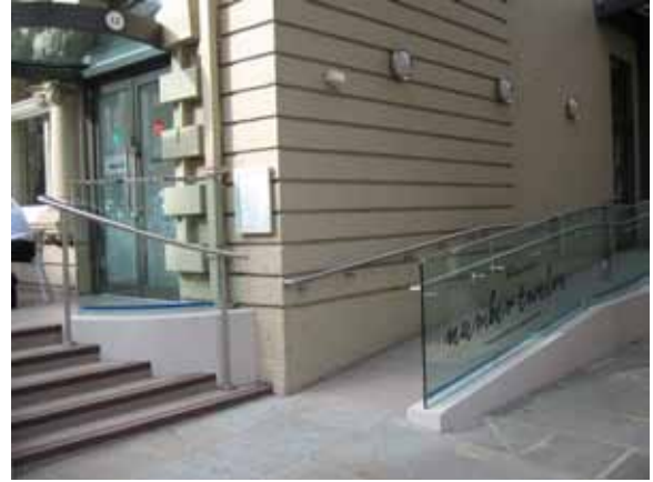
A ramp to an alternative entrance starting from the foot of the steps provides a clear alternative to the steps to the café
