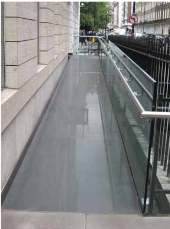
This etched glass ramp has been installed over the area behind the existing railings to provide step-free access to the main entrance of this office building, while still allowing light into the basement area
