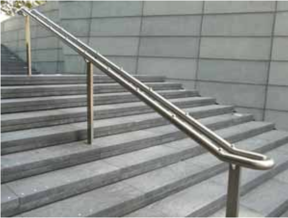
This external stainless-steel handrail to an office building has raised profiles on the top to prevent youngsters using the handrail as a slide: these will prevent people being able to easily move their hand up or down the rail and the stainless steel will be cold to the touch in winter
