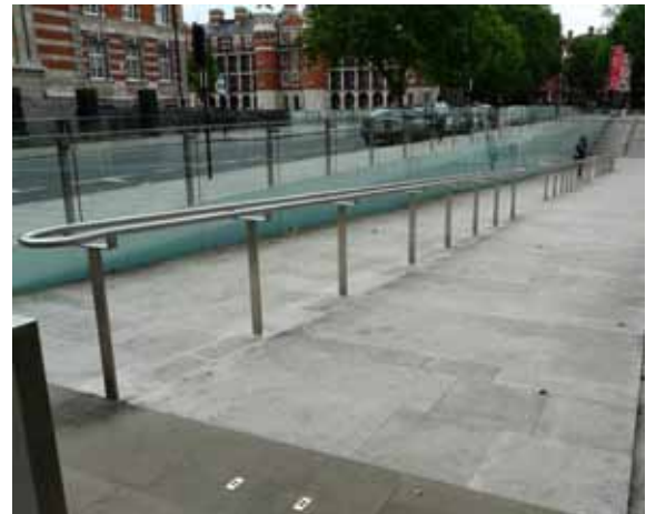
A double central handrail on this wide ramp provides a choice of side for support and helps to avoid a clash of hands
