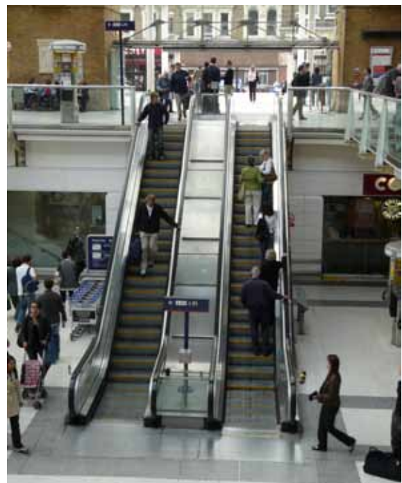
Side-by-side escalators in the concourse of a mainline station provide easy and immediate access to and from the first floor and street level. Note the clear signage to the lifts as an alternative means of access at the top and bottom of these escalators
