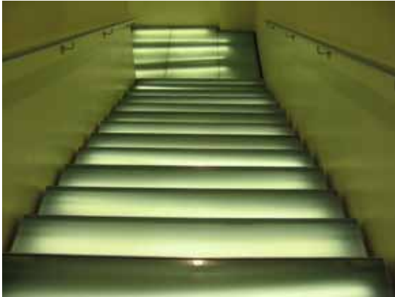
These glass stairs, lit from below, are likely to cause glare and be confusing to visually impaired people
