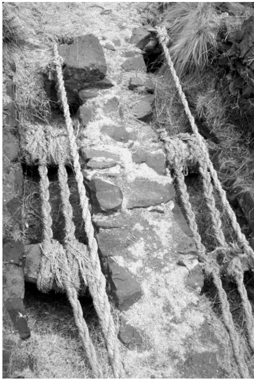
Figure 17.23. The cables of the Quesuachaka Bridge are tied to masonry archers on each side of the river. (Photograph by the author, 1989)
