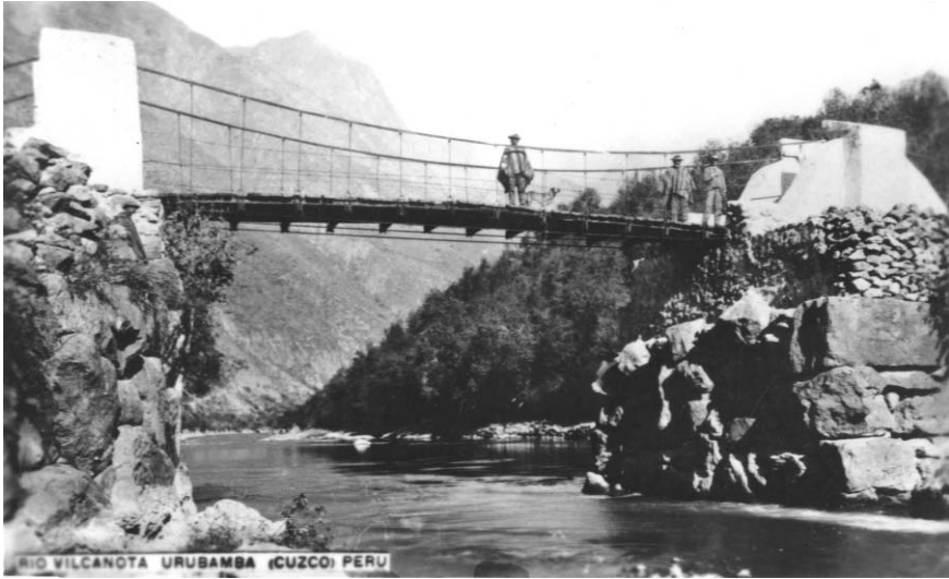
Figure 17.2. The western span and the central support of the Ollantaytambo Bridge. While the Inca platforms for the bridge are well preserved, the bridge towers used to suspend the cables have been rebuilt with stone and mortar. Also note the use of metal cables that allows the suspension of a flat walkway. (Anonymous, ca. 1930)
