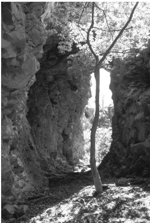
Figure 17.14. Once high enough for mounted horsemen, the tunnel that leads to the Apurimac Bridge site is now filled with debris (Photograph by author, 1987)
