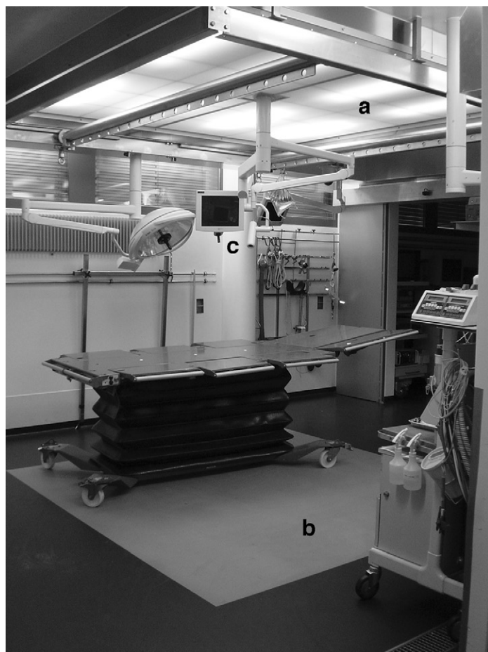
Figure 10-7. View into the aseptic surgery suite of the Equine Hospital, University of Zurich. a , The laminar air filter is illuminated. b , The grey area marked on the floor delineates the extent of the filter field. The surgery site, the surgeons, and the instrument tables need to be located within this field during surgery. (A mobile Haico, surgery table [Loimaa, Finland] is shown in the room). c , A movable video camera (left) is mounted on the ceiling together with a video screen.
