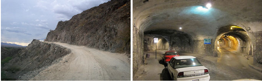
Fig. 2.8 Left : Unpaved road near Salta in Argentina. Right : Roads in tunnels (below the historic centre of Guanajuato) (Courtesy of the authors of [237])
