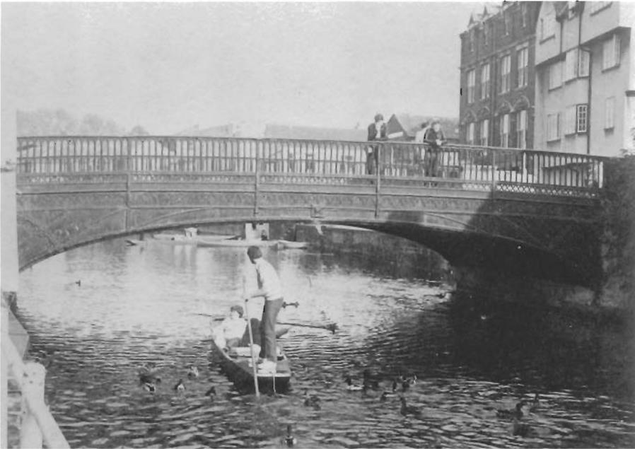
**Fig. 1.4.** Magdalene Bridge built in 1823 on the site of the ancient Saxon bridge over the Cam. The present cast-iron arches carried, until recently, loads far in excess of those envisaged by the designers. Fortunately, the bridge has now undergone a well-earned restoration.
