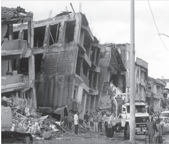
Figure 38.3: Collapsed buildings in the August 1999 Izmit earthquake Source: EERI; at: < http://www.eeri.org/lfe/turkey_kocaeli.html >.
