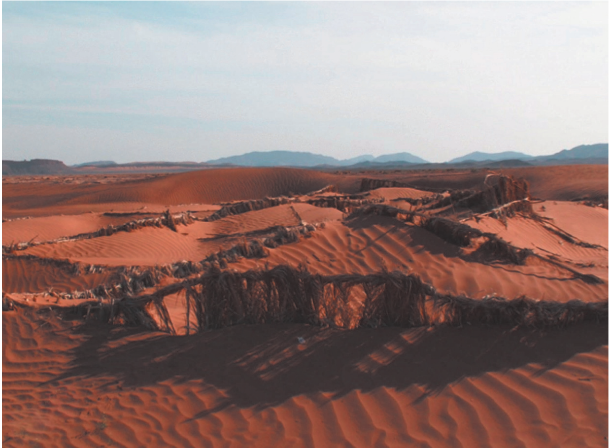
Figure 53.5: The checkerboard of protection of the Rissani-Alnif road is completely filled and in a state of advanced decay. This device, not followed by biological fixation, took part in the accumulation of considerable sandy volumes which are now an immediate danger for the road. Source: © Photo taken by the authors, F. Dumay and M. Mainguet.
