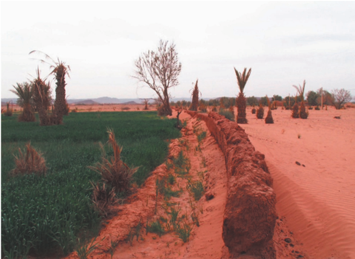
Figure 53.6: Aït Ben Omar. Wall of protection against sand encroachment. The wall plays an effective role in stopping the sand. Source: © Photo taken by the authors, F. Dumay and M. Mainguet.
