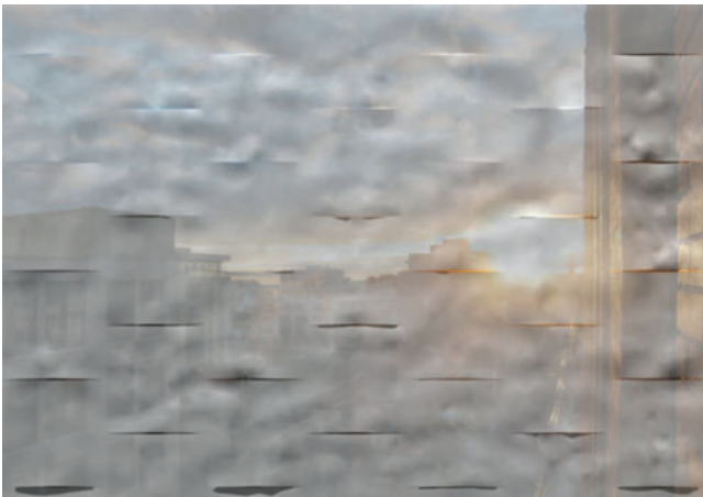
Fig. 4.35 Decker Yeadon LLC, Smart Screen project, version one: a solar shading system opening and closing in response to the changing room temperature
