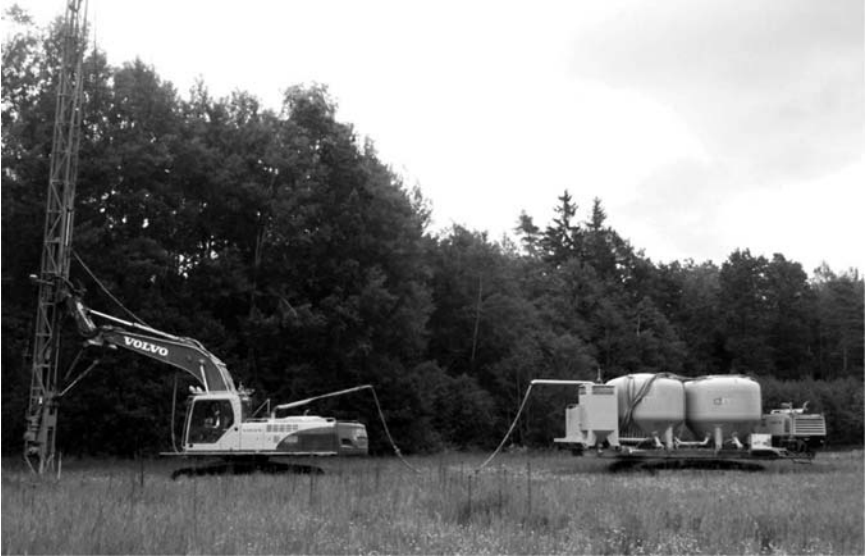
Figure 10.9 DSM machine unit, drilling rig, and shuttle. (Courtesy of dmixab.)
