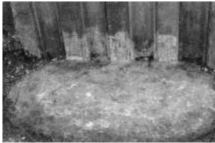
Figure 6.11 JACSMAN column abutting sheet piling.
