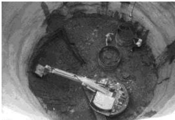
Figure 6.39 Shaft excavation in progress.
