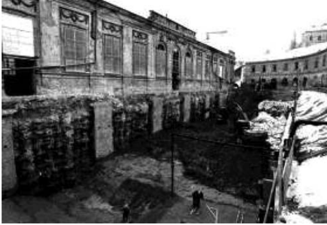
Figure 6.25 Exposed jet grout underpinning adjacent to an excavation in London.
