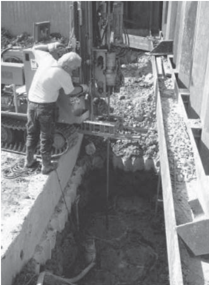
Figure 10.33 (a) Testing of DSM columns. (b) Printout of KPS tests. (Courtesy of dmixab.)
