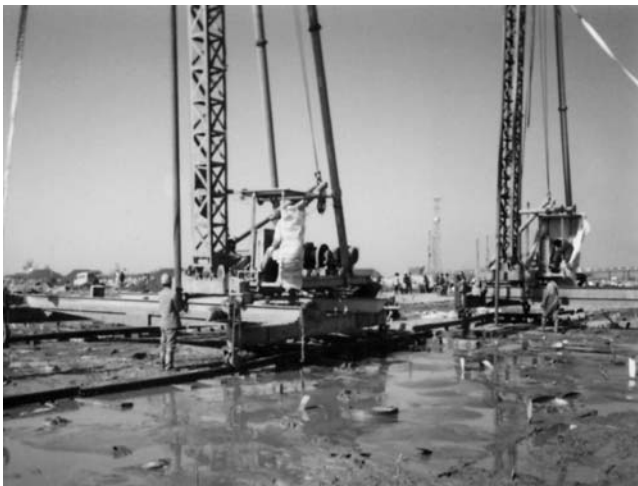
Figure 4.14 A light-weight truck-supported installation rig. (Courtesy of S.W. Yan.)
