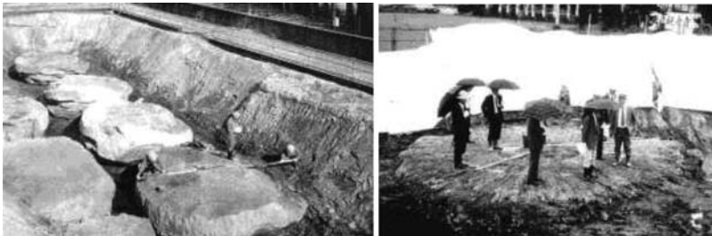
Figure 6.5 Exposed SuperJet columns during technology development.
