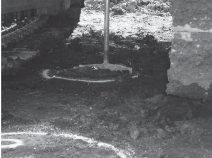
Figure 10.25 Field test with column penetration tests. (Courtesy of Keller Géotechnique.)
