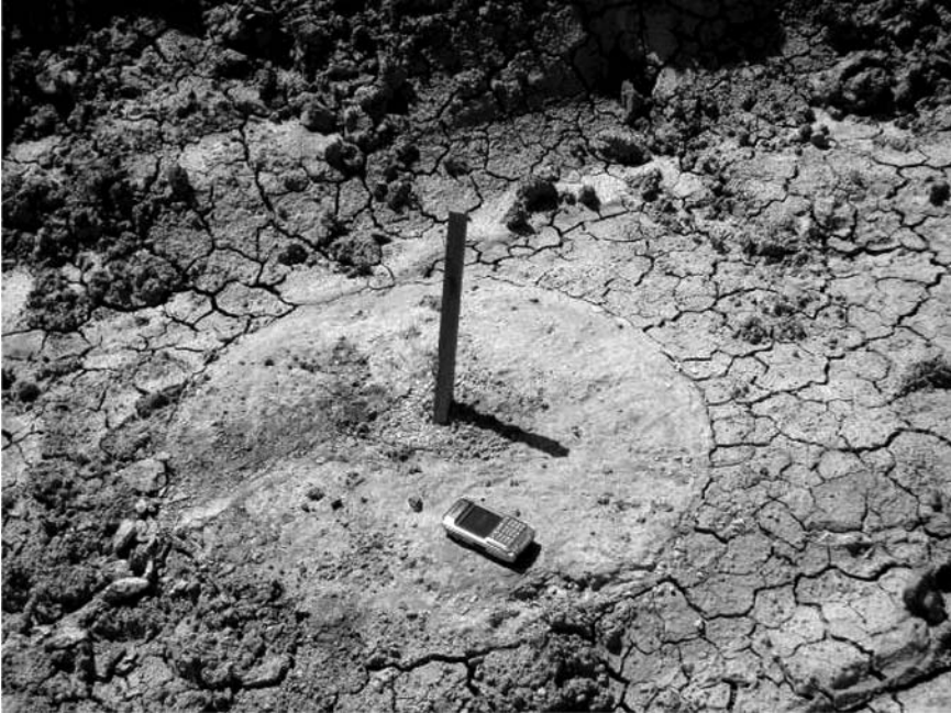
Figure 10.21 Exposed DSM column.
