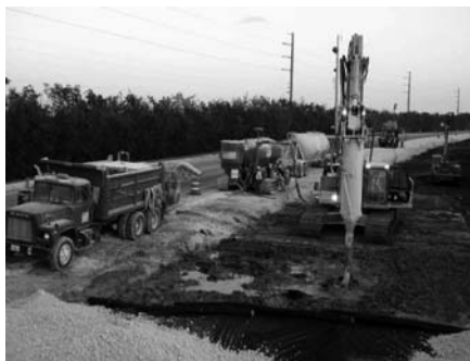
Figure 10.31 Production of mass mixing on site. (Courtesy of Hayward Baker.)
