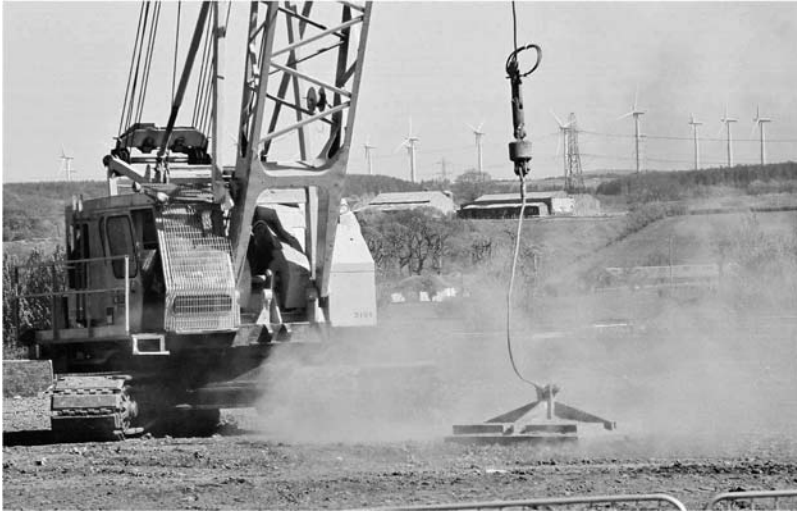
Figure 3.1 Typical crawler crane and equipment.
