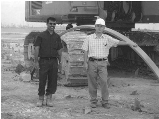
Figure 4.18 A bent mandrel coming out of the ground.
