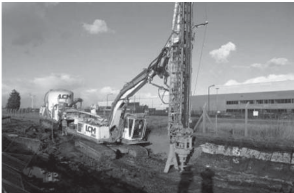
Figure 10.24 Installation of DSM. (Courtesy of Keller Géotechnique.)
