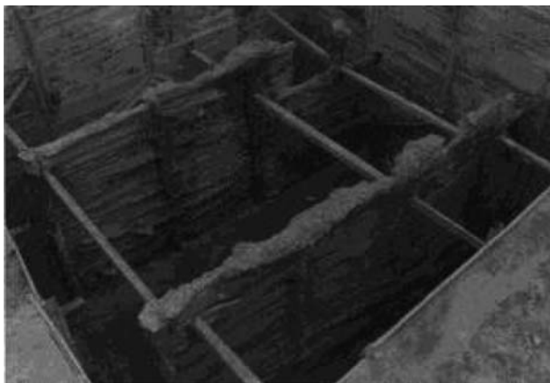
Figure 6.2 Exposed jet grout panels.
