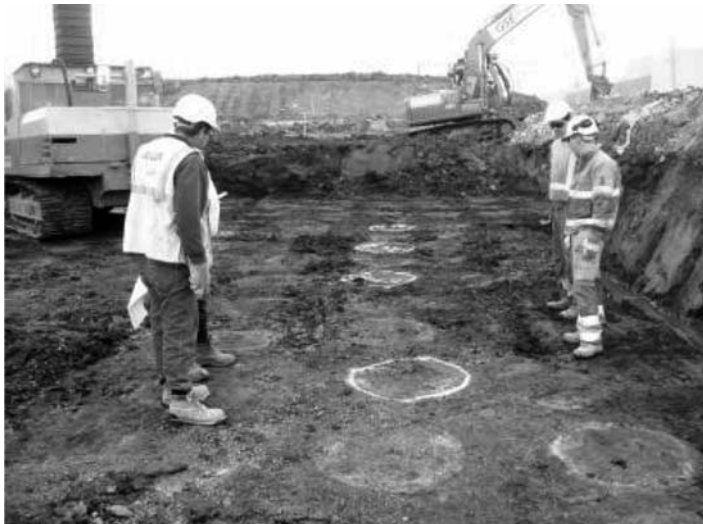
Figure 10.26 Exposed columns for visual examination. (Courtesy of Keller Géotechnique.)
