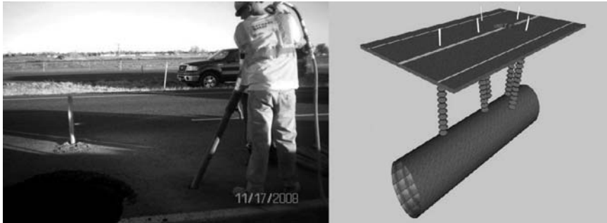
Figure 8.23 Compaction grouting densifies soils loosened during tunneling operations. (Courtesy of Hayward Baker Inc.)
