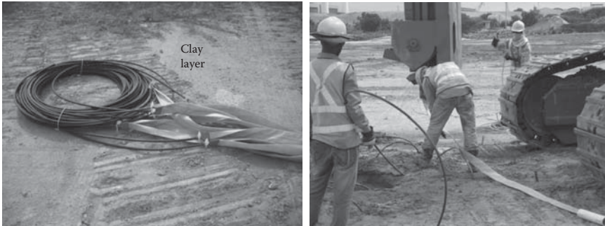
Figure 4.46 Installation of PVDs with plastic pipe connected.
