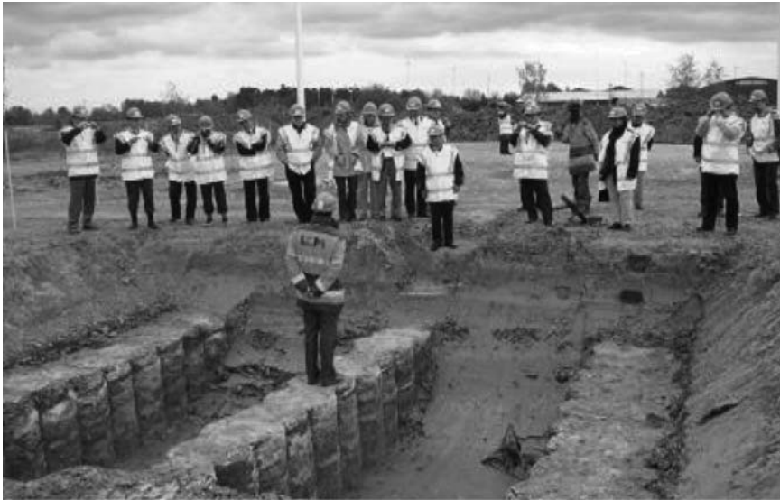
Figure 10.12 Interlocking columns in panels at Bärbyleden, Uppsala, Sweden.
