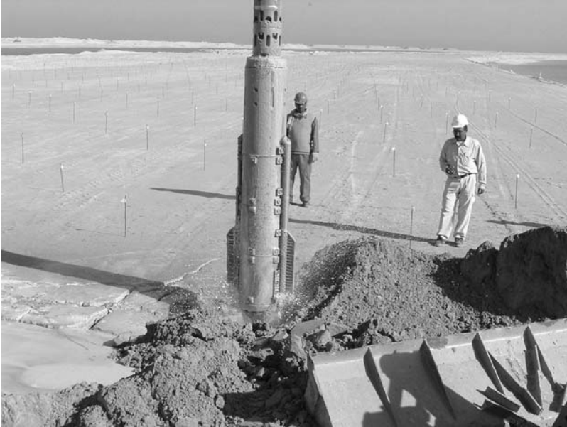
Figure 2.19 Compaction works at Palm Island.
