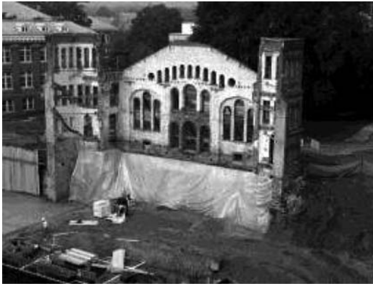
Figure 6.45 Excavated Avery Hall façade underpinned with jet-grouted soilcrete columns.
