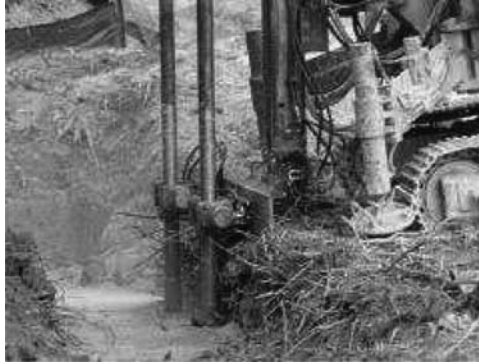
Figure 6.31 Dual axis jet grouting operation for the jet-grouted soilcrete barrier wall.
