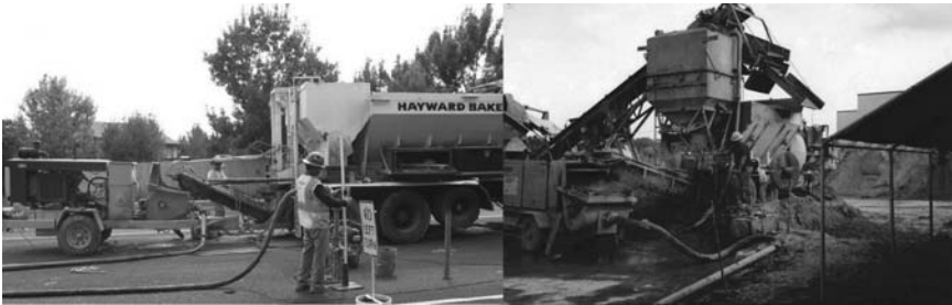
Figure 8.11 Examples of on-site LMG batch plants. (Courtesy of Hayward Baker Inc.)
