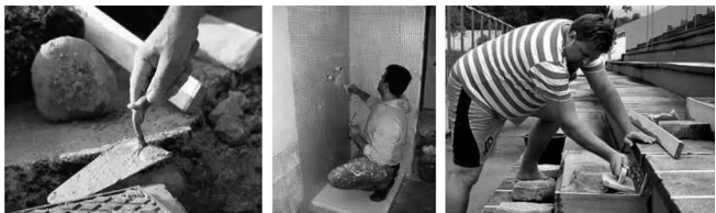
FIGURE 8.69 Principal building tasks.
