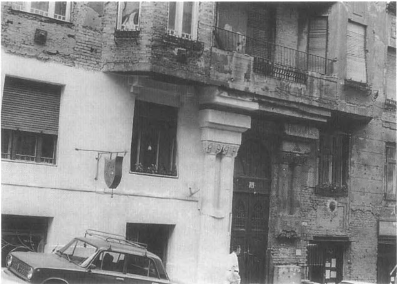
Figure 4.7. Partial gentrification: one-half of ground floor exterior finished. Photograph by author.
