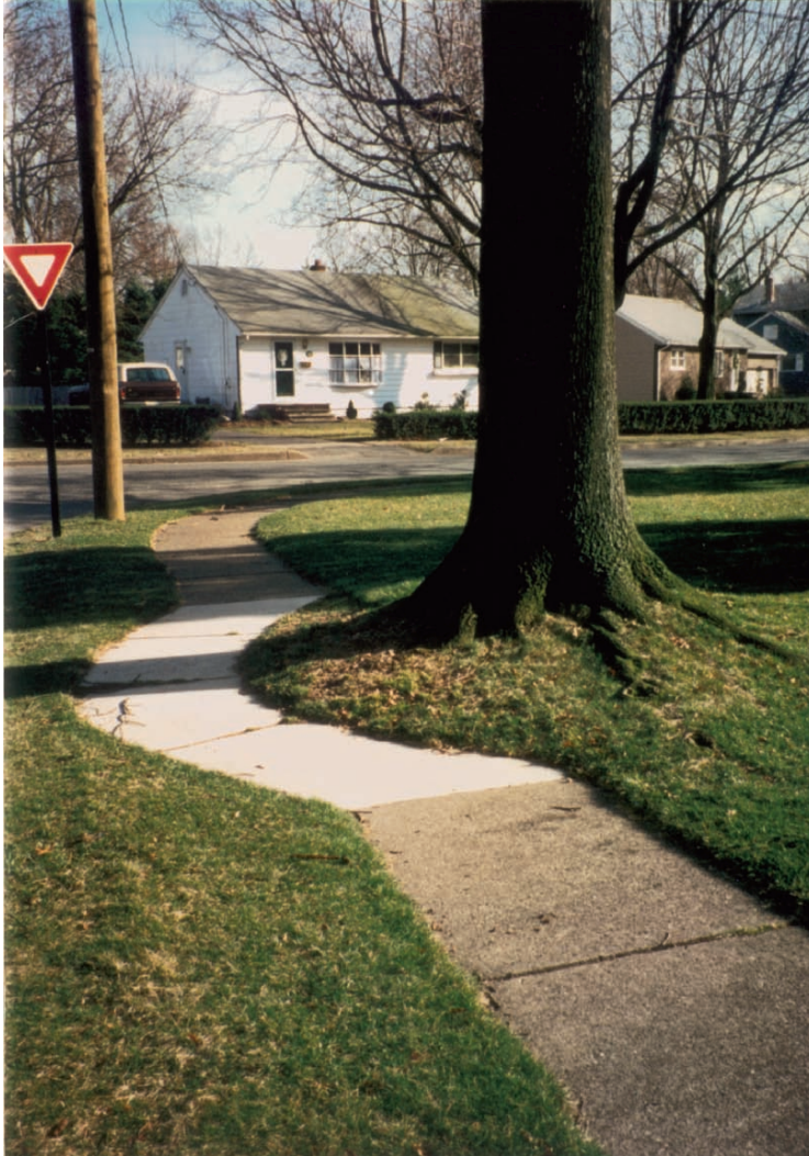
FIGURE 5. Example of contoured sidewalk installation. Who said must be straight and level? Sidewalks must be safe, functional, and appropriate for their location. Photo, William R. Comery.
