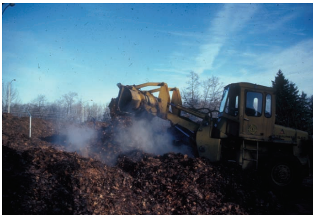
FIGURE 1. Combining two small piles using front-end loader. (Photo by P. F. Strom.)
