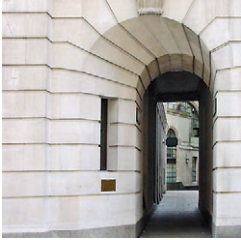
Entrance to alley, Cornhill.
