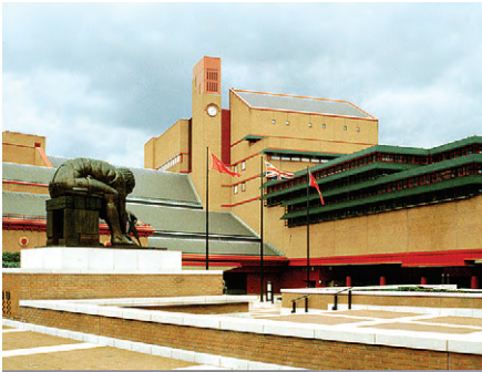
The British Library forecourt area — which is slowly being inhabited, with cafes, etc., thus hugely improving an original bleakness.
