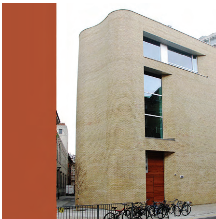
The Wild Street façade is comparatively that: a curvy, Aalto-esque piece of playfulness that nevertheless introduces a scale addressing the adjacent Freemason's Hall. Purists may object to the tectonics of 'floating' brickwork without lintels.
