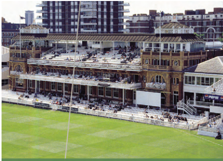
The Verity Stand is oldest on the site and remains the most prestigious because of its historical associations and continued use as the principal club house.
