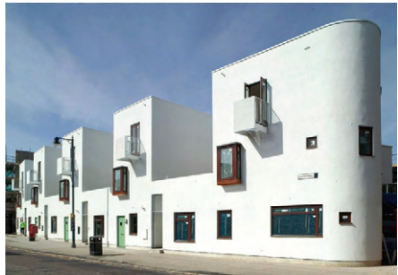
Images (top to bottom): Donnybrook; axo of Donnybrook scheme and two images of Tanner Street nearing completion. Note the inter-war mock 'tudorbethan' housing on the left.
