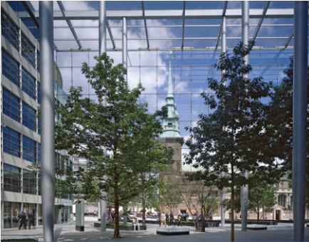
The atrium's wall of glass stops about 3-4m above the paving, producing a sheltered but still outdoor area.
