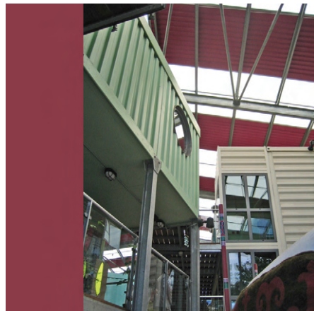
The internal pavilions are simply stacked steel pavilions accessed by spacious galleries. The spaces provided are there to serve an 'inclusive' grouping of children of all abilities.
