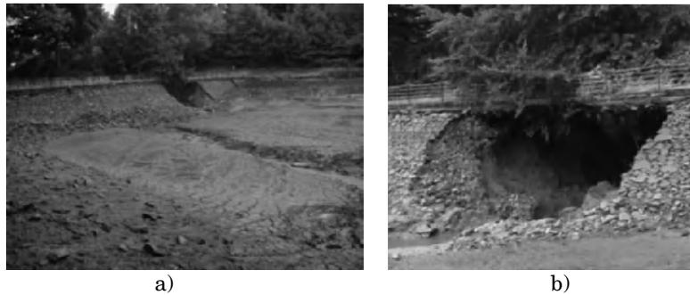
**Figure 4.2.** *Les Ouches dam built in the 18th Century (France), concentrated leak erosion occurred two centuries after construction in 2001: a) general view and b) close up view of the pipe*
