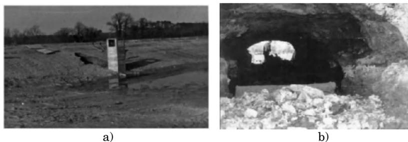
**Figure 4.1.** *Saint-Julien des Landes dam built in 1969 (France), concentrated leak erosion occurred during first filling: a) general view of the upstream slope and b) close up view of the pipe*
