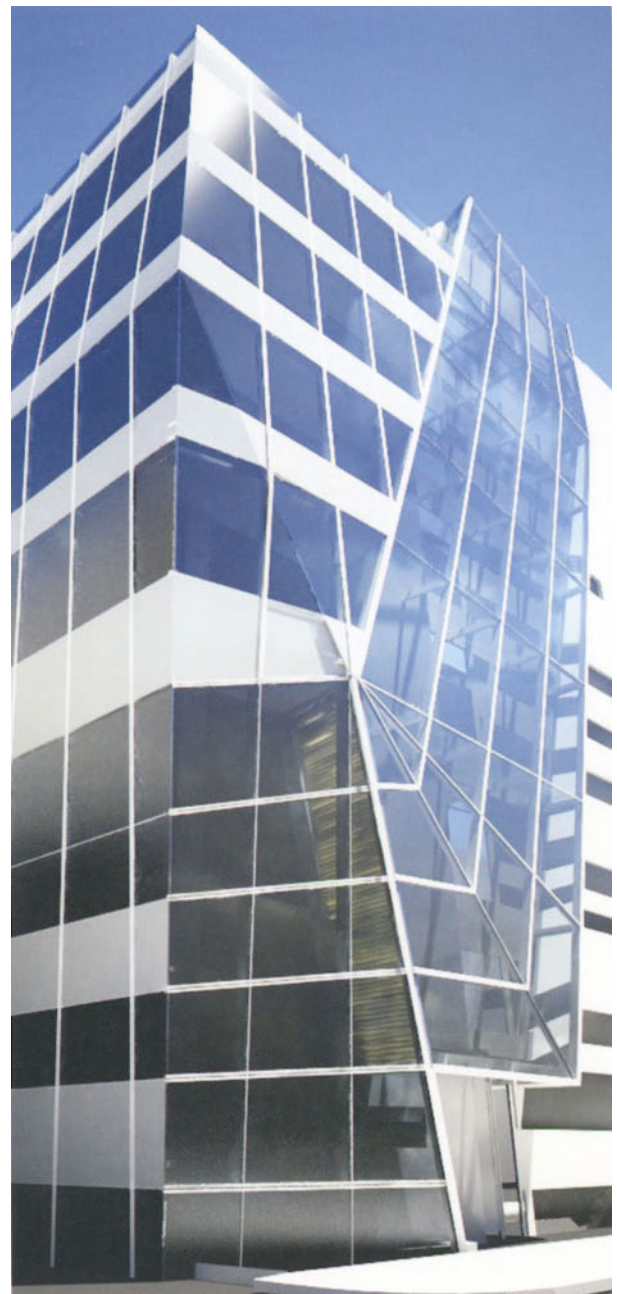
Flat pieces of glass fixed at varying angles to create a folded facade
