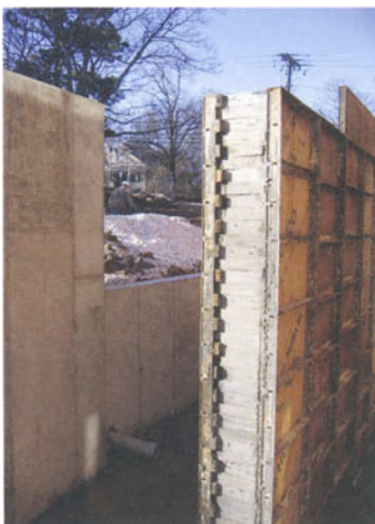
Timber formwork used to achieve decorative texture
