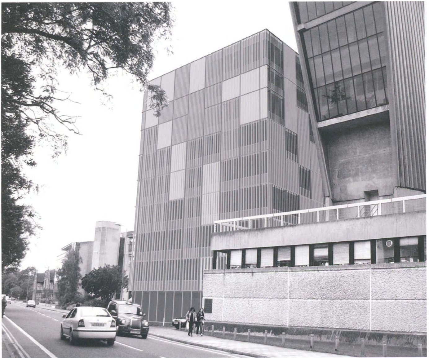
Rendered views a cladding system with integrated louvres
