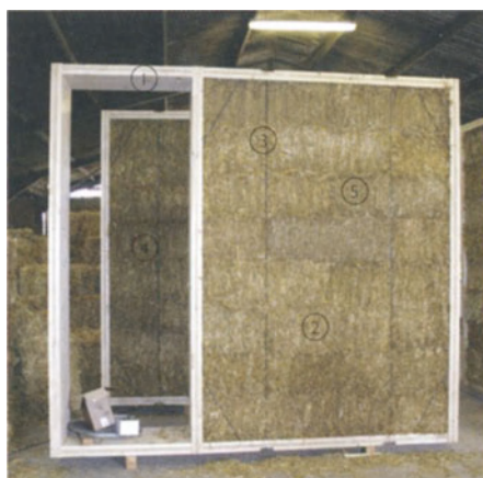
ModCell straw panel being constructed(left) and Modcell hemp (right)
