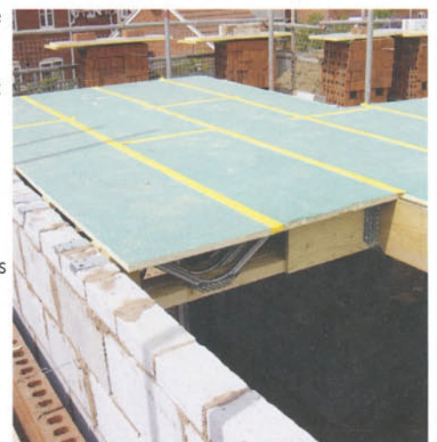
Typical timber floor construction with masonry structure. Timber boarding used for stiffness
