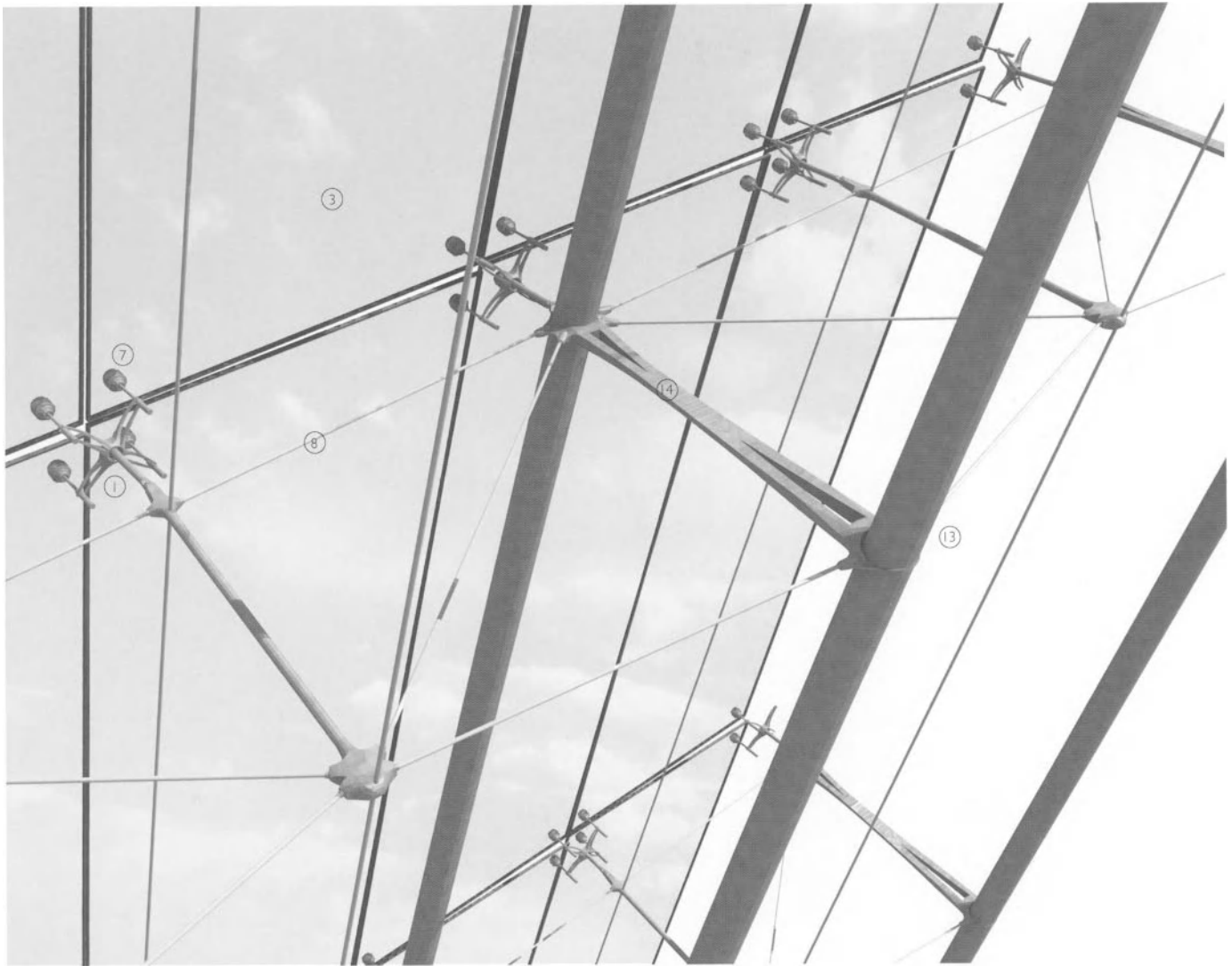
3-D view of bolt fixed wall system
