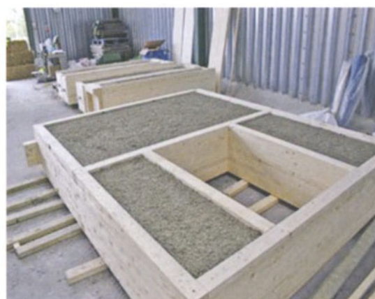
3-D view of modularised components that can be created using the modCell system
