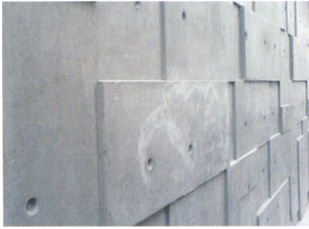
Photos illustrating texture that can be achieved through in-situ casting
