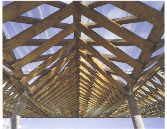
Timber trusses in tree-like arrangement.
