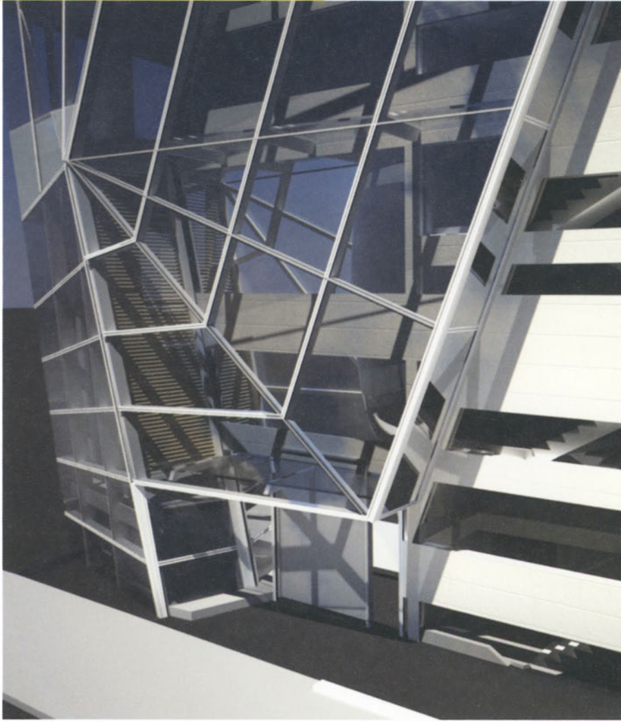
Flat pieces of glass fixed at varying angles to create a folded facade
