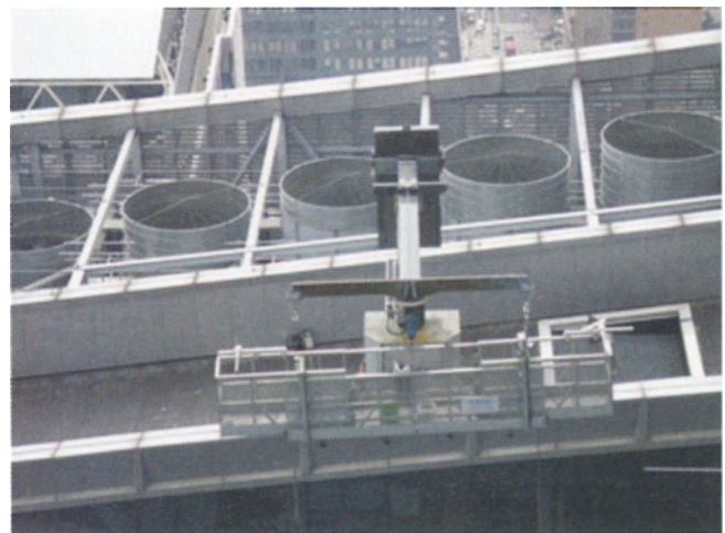
(Above). Cleaning cradle on trolley around Swiss Re building, London. Architect: Foster and Partners
