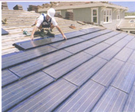
Photovoltaic or solar tiles being applied to timber roof
