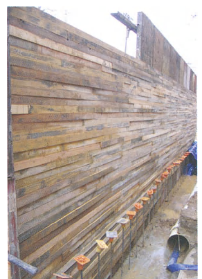
Timber formwork used to achieve texture
