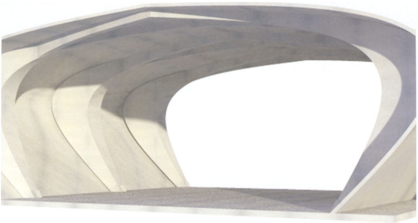
Rigid reinforced concrete portal frame
