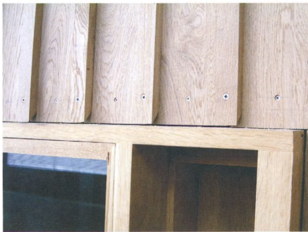
Examples of vertical and horizontal cladding arrangements
