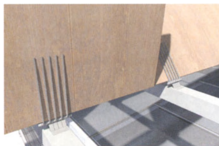
Above. Louvres can be perforated or solid to provide different amounts of shading Left. Wind animated tiles
