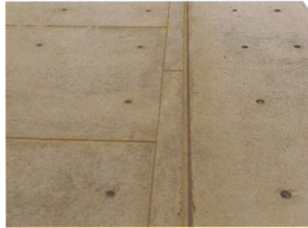
Photos illustrating texture that can be achieved through in-situ casting
