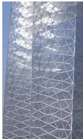
Studies where a complex geometry has been rationalised to allow it be made up of repeated triangular panels
