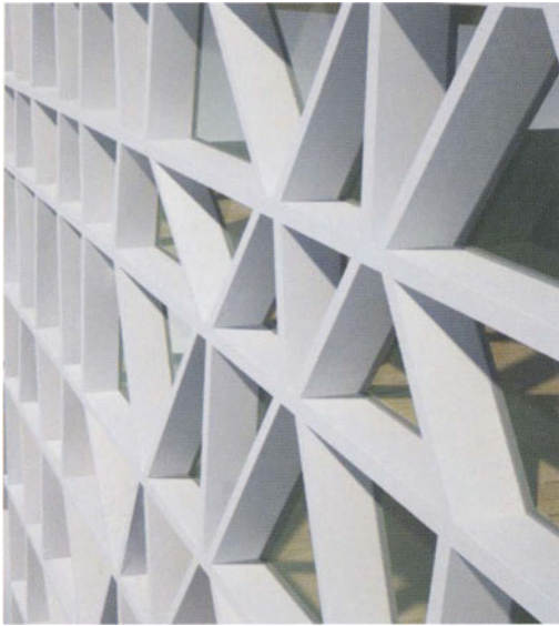
Structural facade solution where a regular column grid is skewed to provide varying amounts of shading where needed
