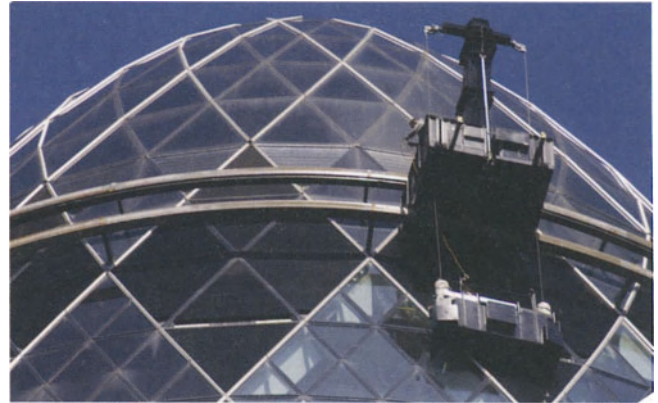
(Above). Cleaning cradle on trolley around Swiss Re building, London. Architect: Foster and Partners
