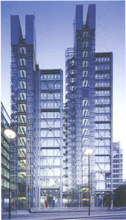
Braced steel framed construction. Wood Street, London. Architects: Richard Rogers
