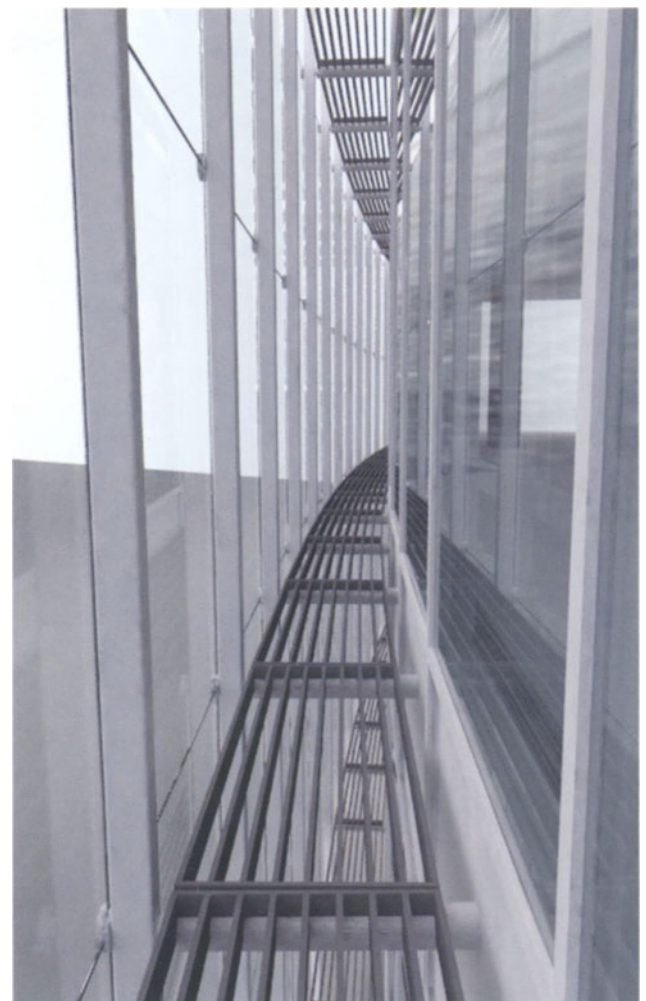
3-D view of twin wall cavity
