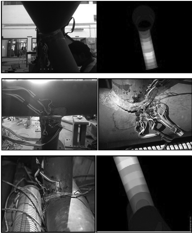
FIGURE 3.39 Failure mode of tubular T joint under out-of-plane bending.
