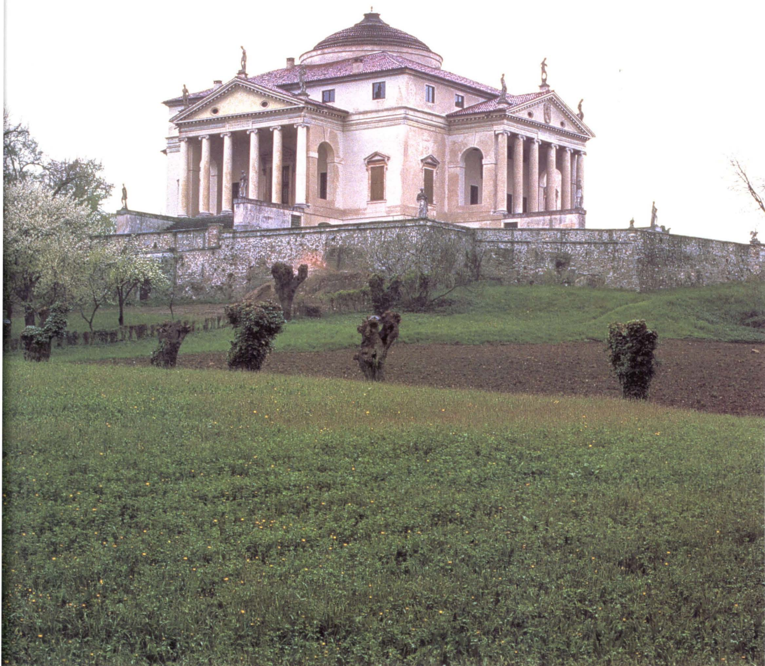
View from the south.
