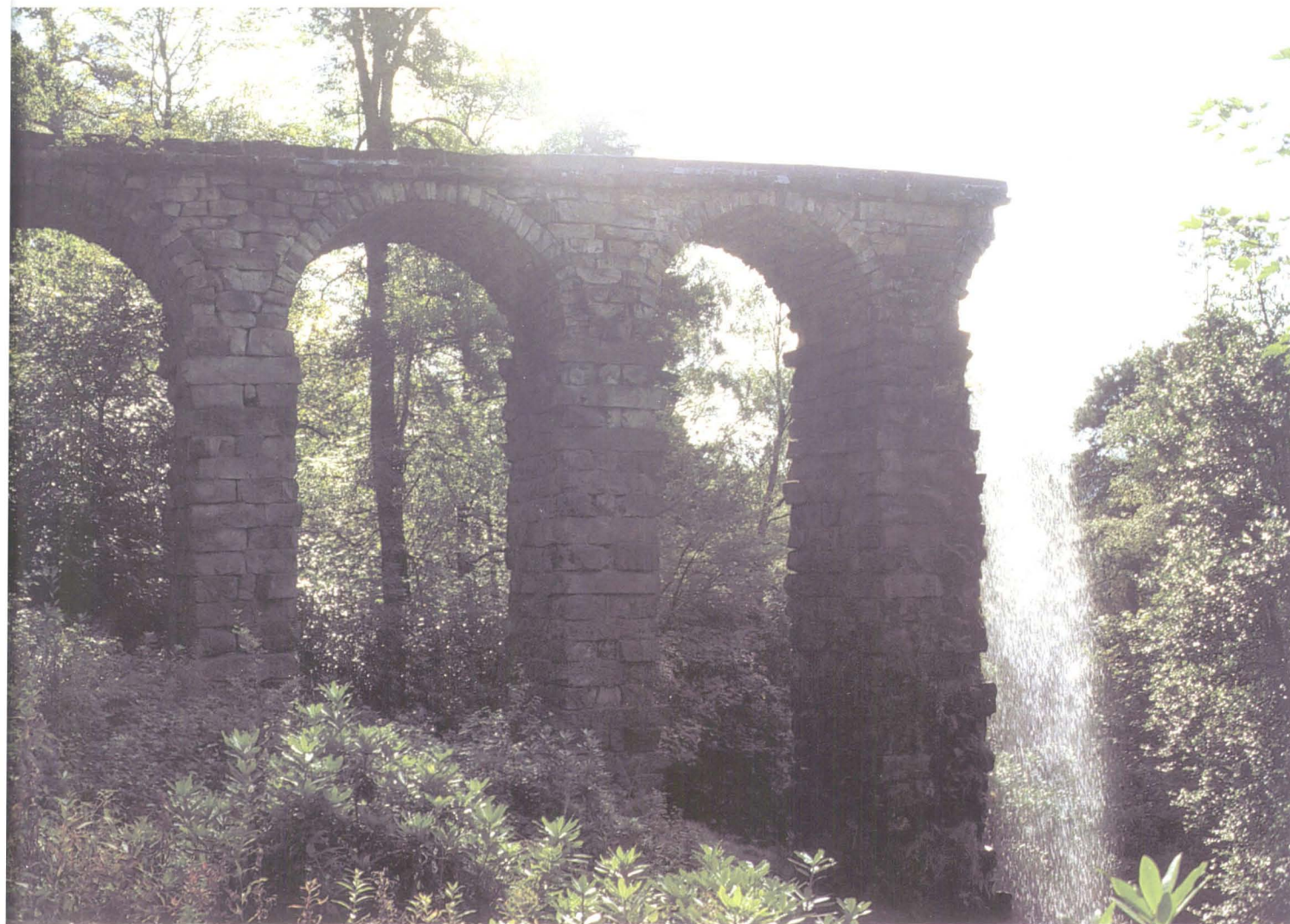
The Cyclopien Aqueduct with waterfall, from Stand Hill.
