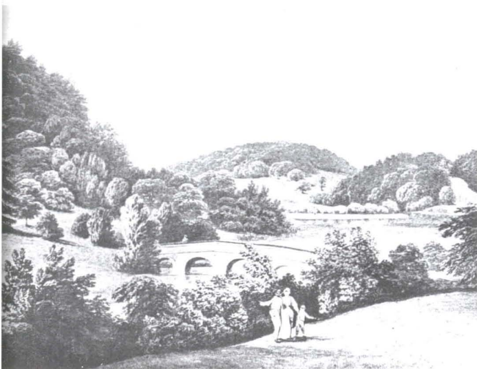
Bridge, lake and south bank. (F. Nicholson, 1813)
