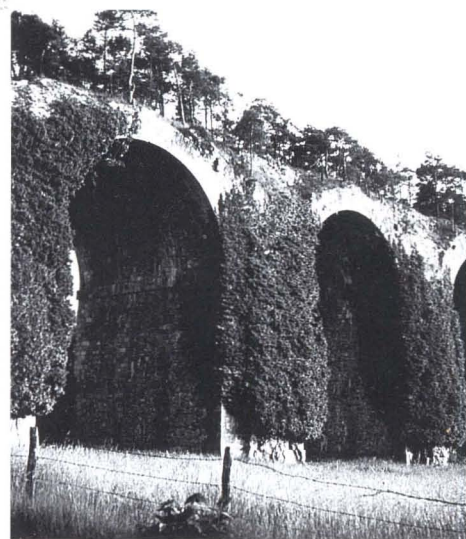
Aqueduct near Marly.
