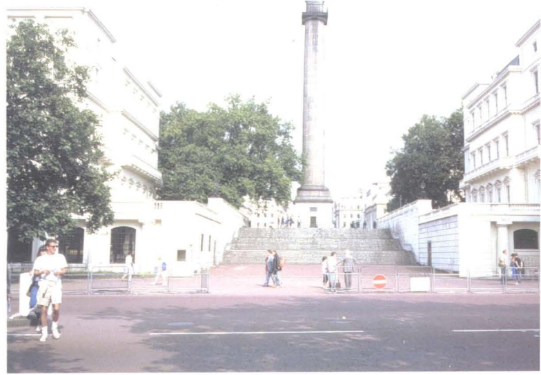
Stair near St. James's Park, on the site of the old Carlton House.
