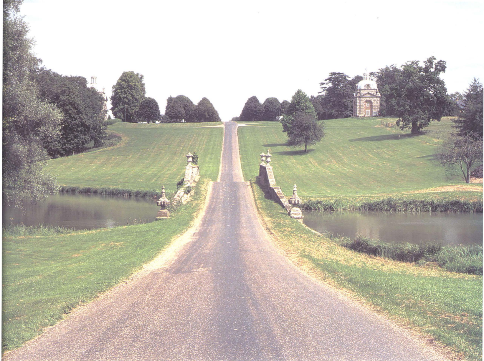
Oxford/Ladymead Bridge and Water, with the Boycott Pavilions in the background.
