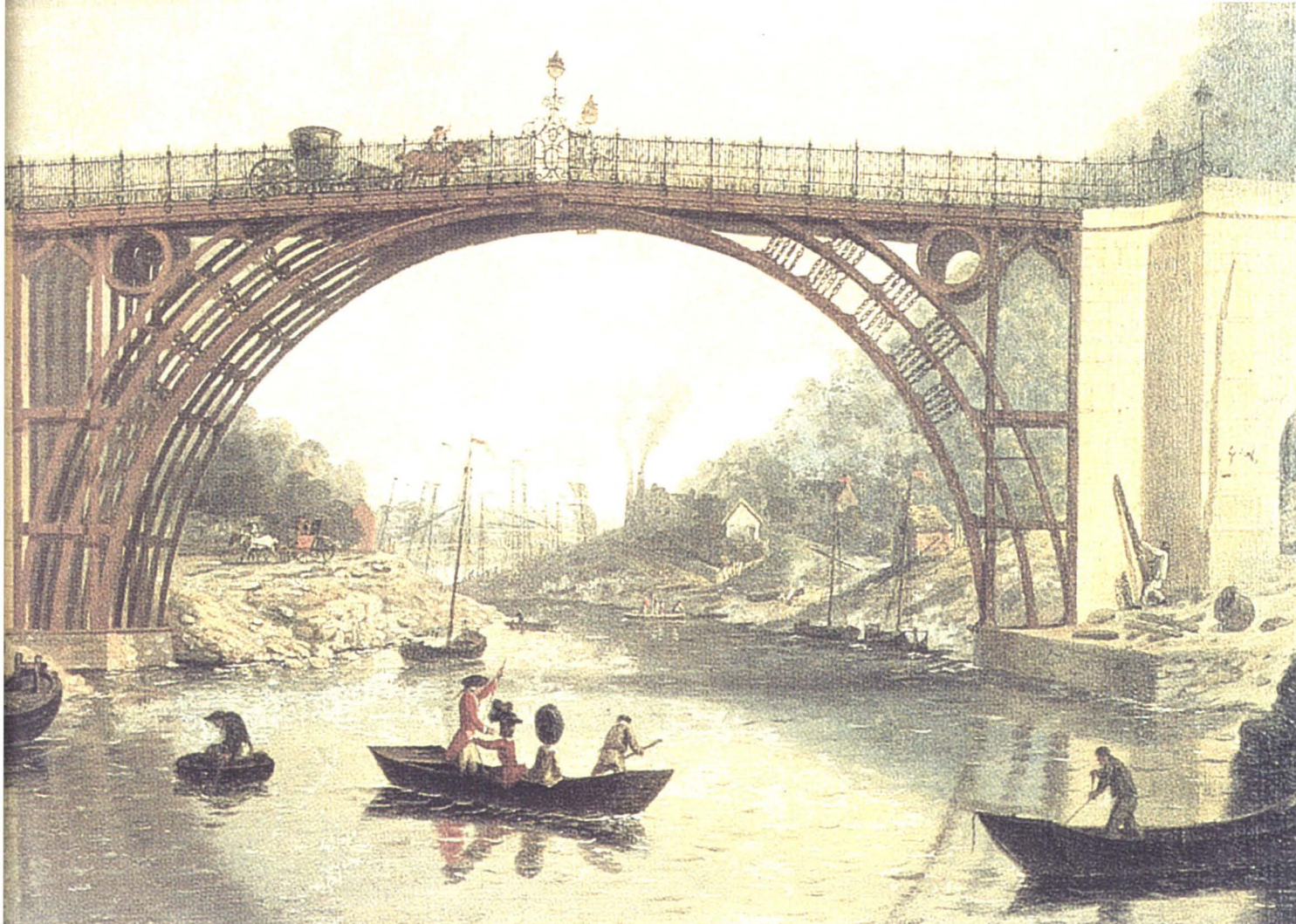
The first cast iron bridge, over the Severn, near Coalbrookdale, 1777-81.
