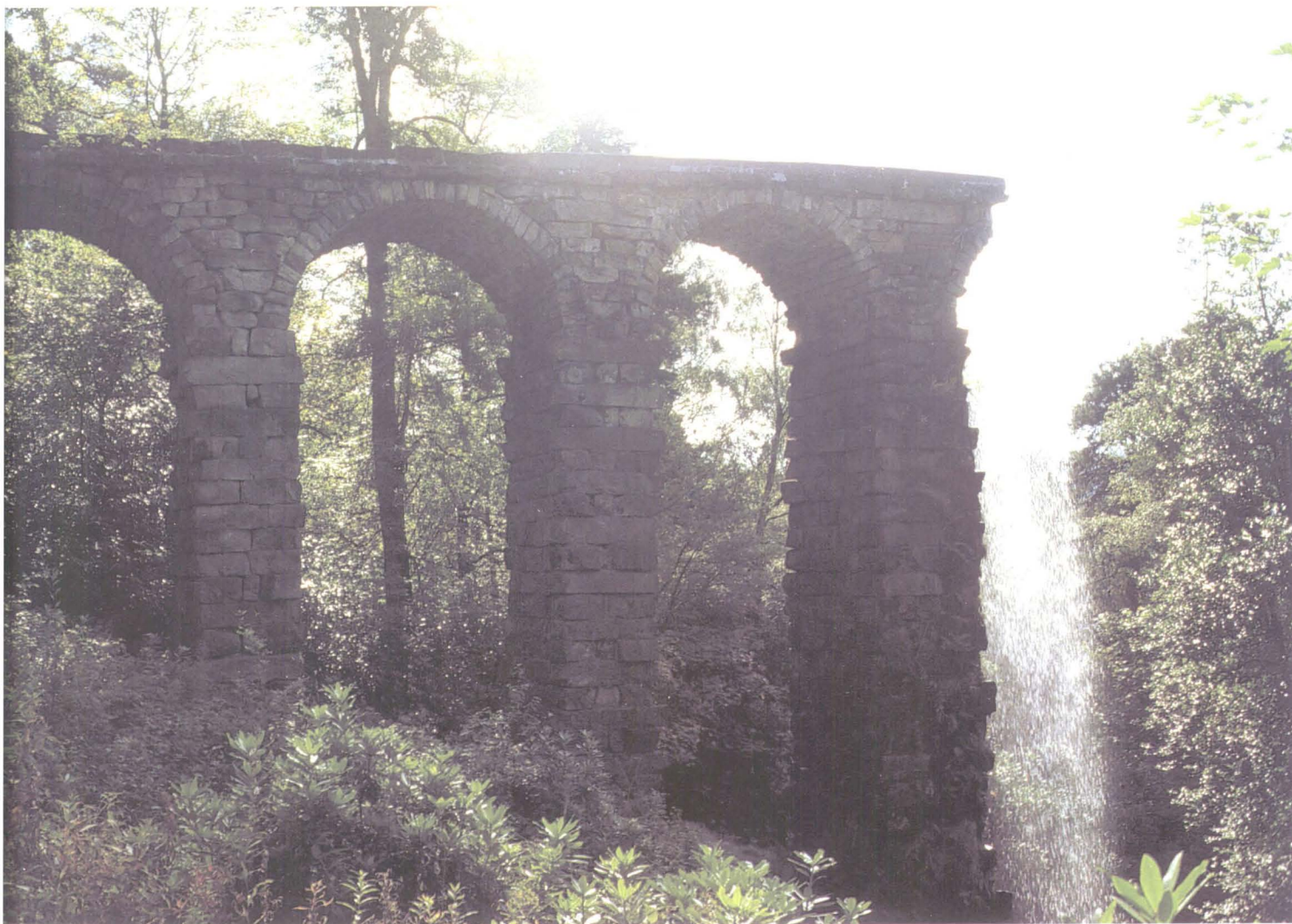
The Cyclopian Aqueduct with waterfall, from Stand Hill.
