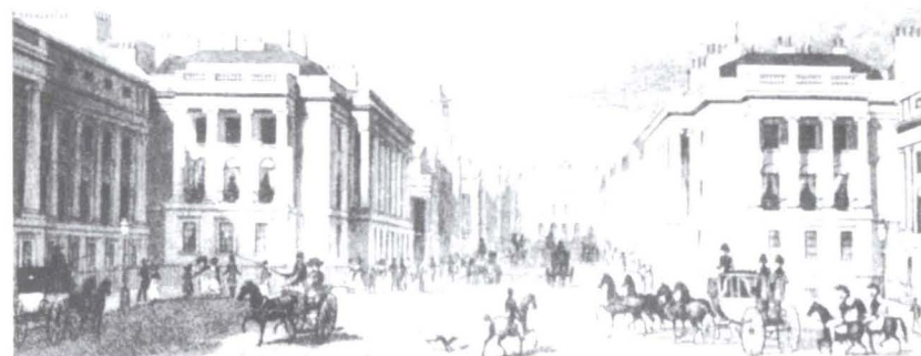
Waterloo Place seen in the direction of the County Fire Office.
