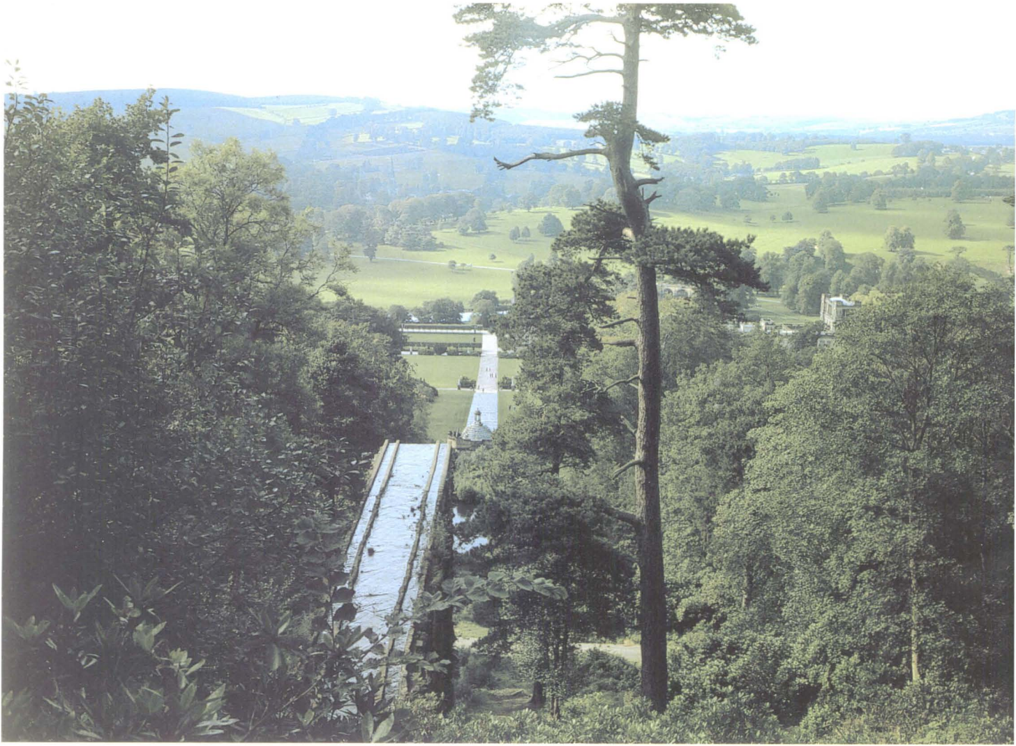
View over the Cyclopian Aqueduct across Brown's landscape.
