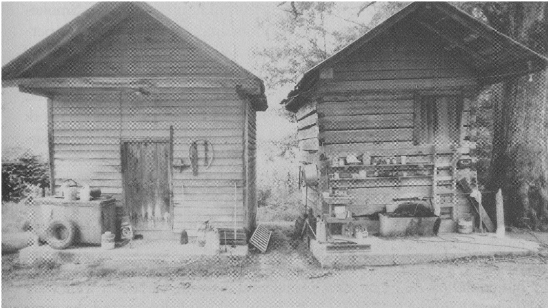
FIGURE 1.18 Two nearly identical Appalachian outbuildings reflect enduring traditions, while employing technologies and materials from different eras of construction. (Photograph courtesy of Tennessee Historical Commission, 1979.)
