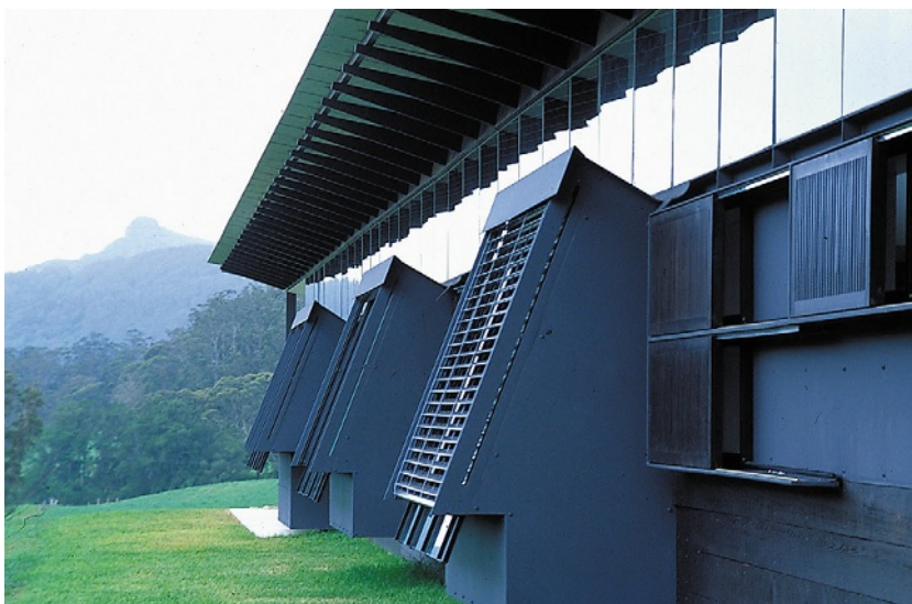
FIGURE 11.26 View of clerestory, light louvers, and sliding screens. (Photograph courtesy of Glenn Murcutt.)
