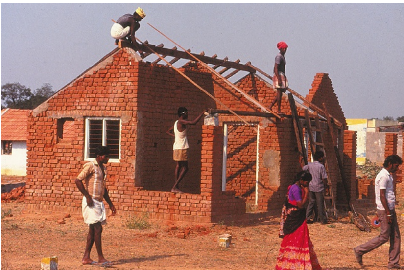
FIGURE 4.12 View of an experimental house during construction. Fired brick was transported by truck from another site that the NGO ran in an attempt to keep resources within the regional community. Though similar to the Mexicali Project under Christopher Alexander, where families designed their own houses, the Vellore settlement, in contrast, used local, well-understood, methods of construction. (Photograph courtesy of Howard Davis.)
