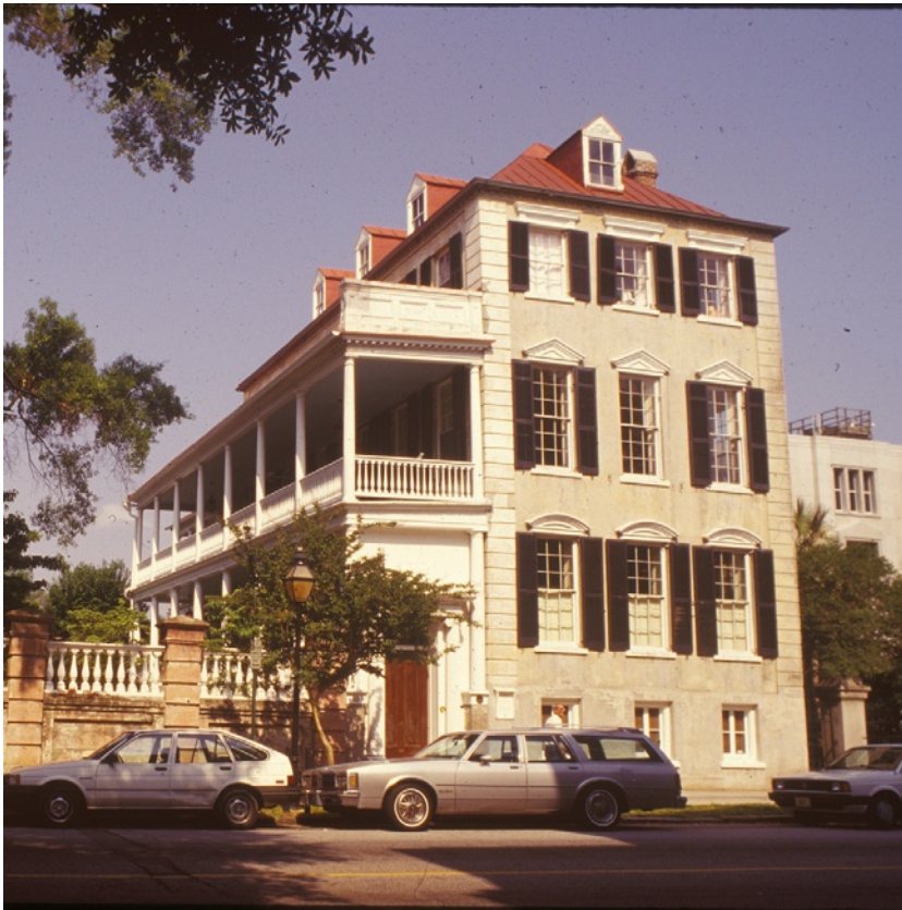
FIGURE 1.4 The Poyas-Mordecai House, an elite version of a Charleston, South Carolina, single house – a subregional building type in the Tidewater South. Its hall-and-parlor plan is oriented toward a side-yard condition and makes use of the porch or piazza as a circulation path, surveillance point, and climate response. (Photograph by the author, 1994.)
