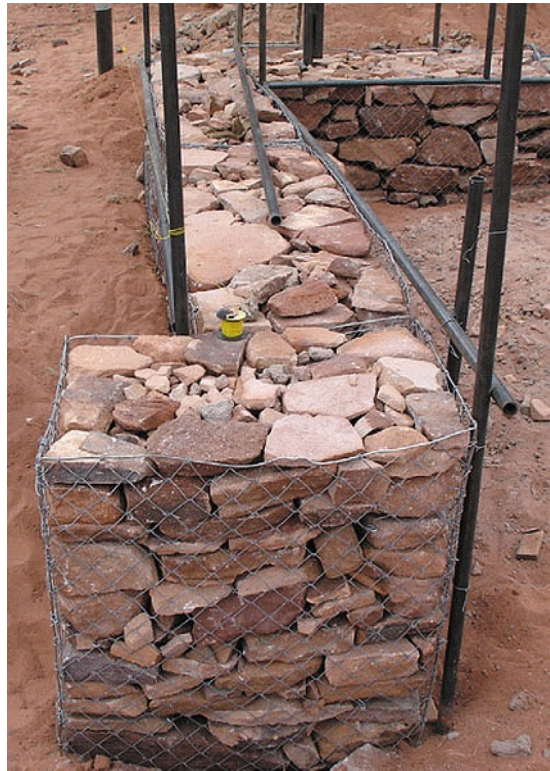
FIGURE 9.26 View of gabion wall baskets hand made on the site. The load-bearing tubular steel frame aided the laying out of the gabion baskets used as a free walling system. (Photograph courtesy of Nina Maritz.)
