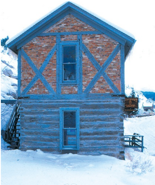
FIGURE 1.10 The Kluge House (circa 1873), a folk housing form culturally transferred from Germany into a mining camp context in Helena, Montana. It is the sole example of this traditional housing type in the state. (Photograph by the author.)
