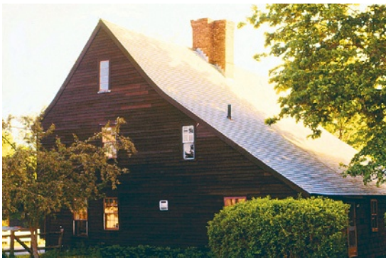
FIGURE 1.14 William Boardman, a successful joiner, constructed his home in 1687 in Saugus, Massachusetts. By 1696, a lean-to or 'out-shot' and fireplace flue were added to the rear of this New England hall-and-parlor traditional form, creating a separate room for cooking. This five-room plan is referred to in New England as a Cape Cod house. (Photograph by the author, 1978.)
