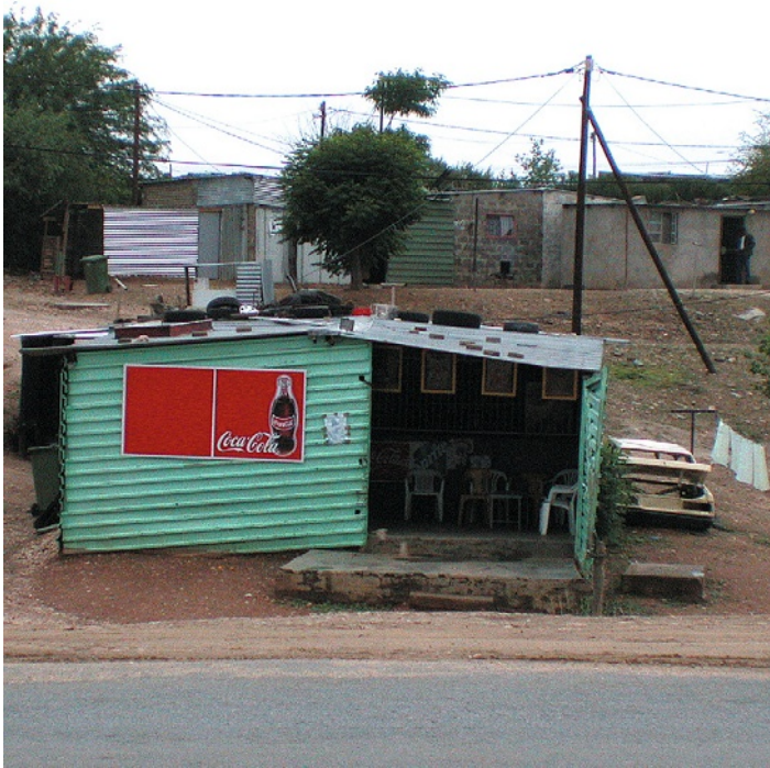
FIGURE 9.12 Corporate metal signage is hung on a steel pole frame to enclose domestic space in a Namibian town context. (Photograph courtesy of Nina Maritz.)
