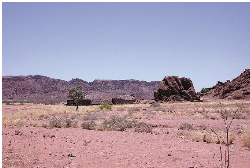
FIGURE 9.27 The materials, building form, coloration, and rhythms are consciously selected to camouflage the building in its desert context. Note the low, irregular form of the museum to the left of the taller rock outcropping. All building elements are completely reversible. (Photograph courtesy of Nina Maritz.)
