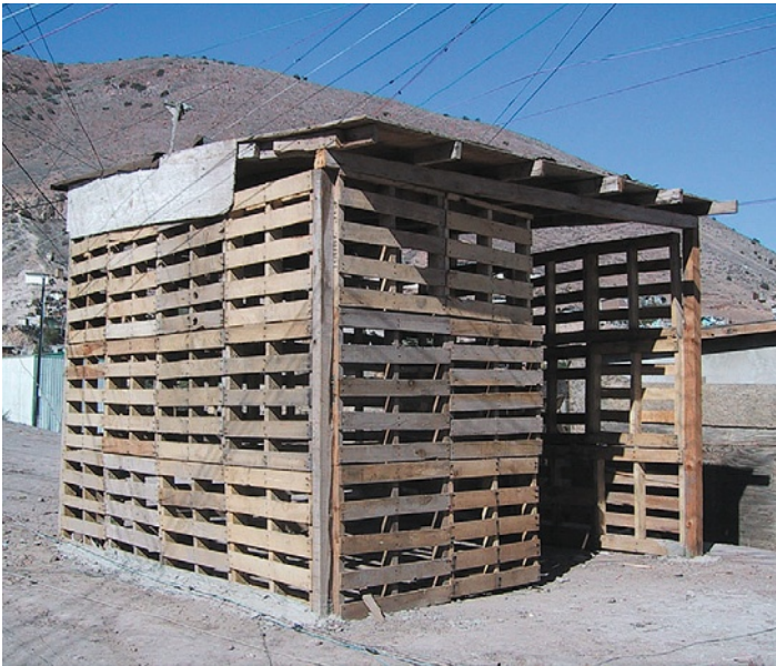
FIGURE 7.4 Improvisation: A dwelling made out of discarded packing crates and corrugated sheet metal erected on the eastern edge of Tijuana. (Photograph courtesy of Teddy Cruz.)
