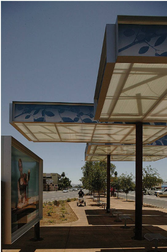
FIGURE 8.29 Daytime site condition as built. Note the shaded sitting areas below the canopies and installed art/sign-shadescreen panels. (Photograph courtesy of Darren Petrucci, 2008.)
