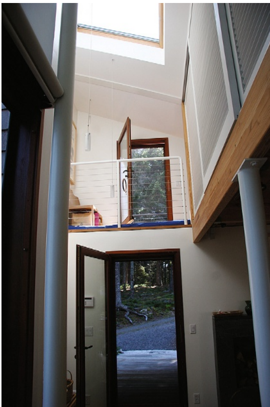
FIGURE 10.15 Interior view looking west, showing the steel columns running through the interior space. (Photograph by the author.)
