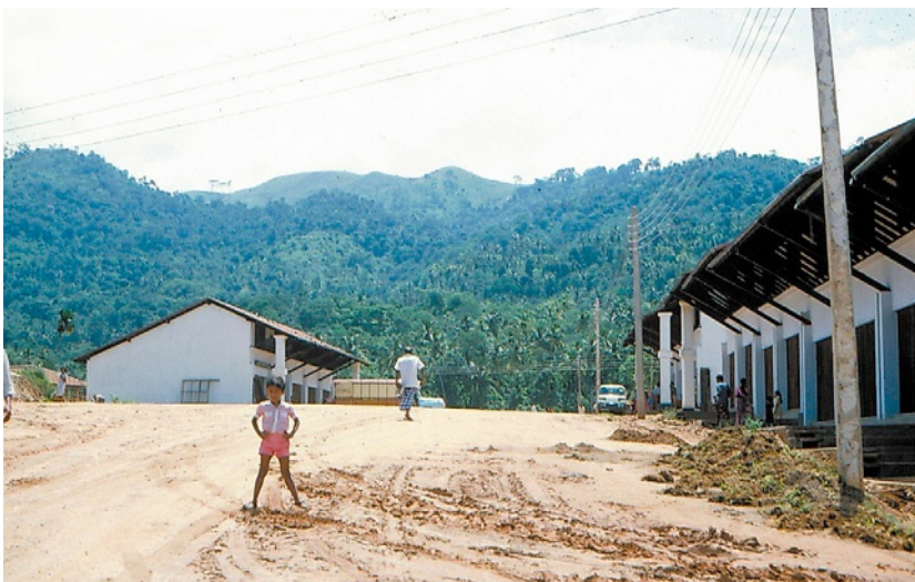
FIGURE 5.8 Structural shells under construction in the center of the town of Teldiniya. (Photograph courtesy of Nihal Perera.)
