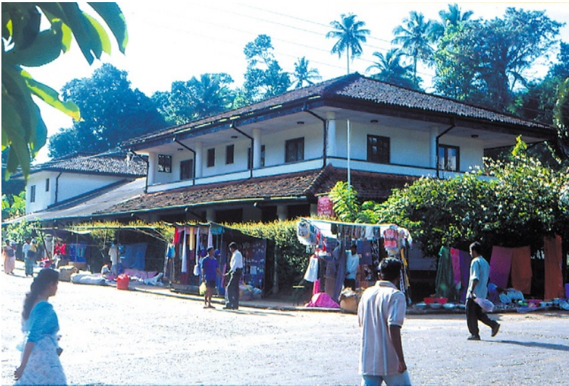
FIGURE 5.11 Three-quarter view of the double-story post office in the new town center of Teldeniya after storeowners and clients responded to Perera's loose-fit design, and reclaimed the building and foreground spaces in a manner meaningful to them. (Photograph courtesy of Nihal Perera.)
