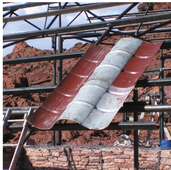
FIGURE 9.9 Construction photograph showing roofing tiles made from quartering recycled 200 liter oil drums. The tiles were sandblasted prior to assembly to remove paint and to enhance rusting for aesthetic effect. The metal cladding (applied in a manner similar to Roman tiles) was then attached to a roof structure made of tubular steel sections welded into curved roof trusses. A layer of sisalation was placed between the steel roof tiles as a waterproof barrier. Hand-made reed mats form a ceiling underneath of mesh-reinforced foil insulation. (Photograph courtesy of Nina Maritz.)
