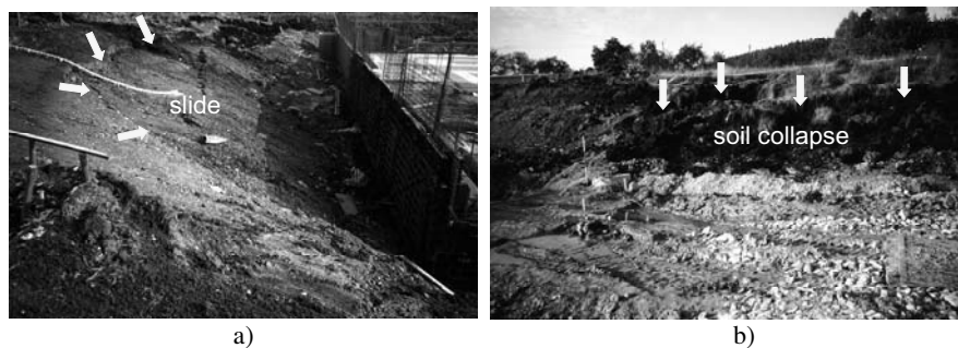
Fig. 4.4. Slope slide and collapse of unprotected slope in soft soil: a) in lacustrine soils; b) in alternate peat and clay layer
