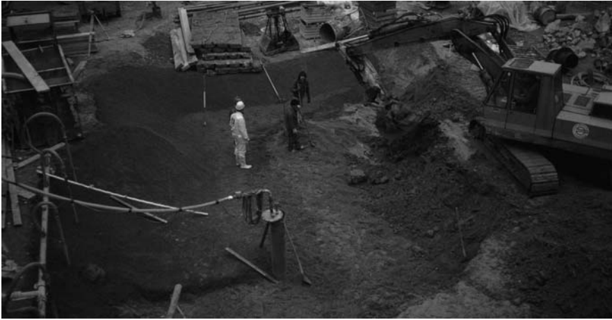
Fig. 4.2. Slope protection using single-grained concrete
