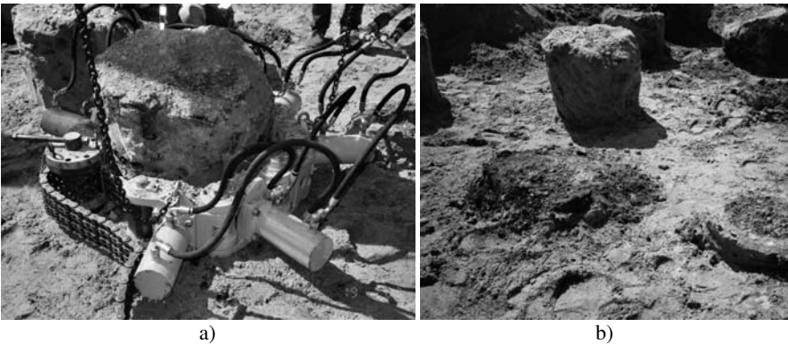
Fig. 7.40. Cutting column heads
