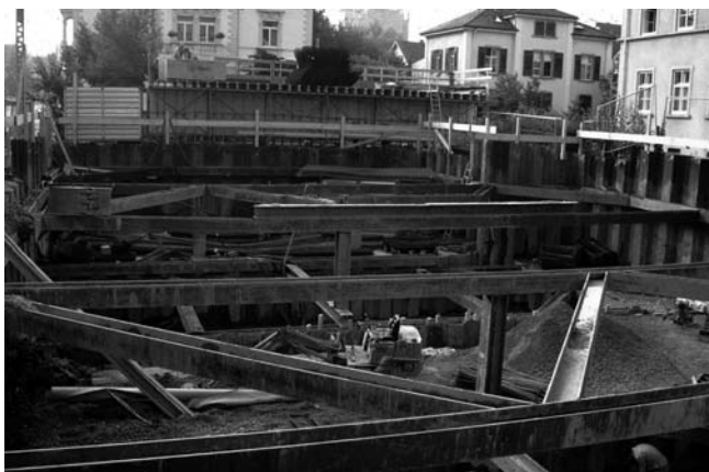
Fig. 4.6. Braced sheet pile wall
