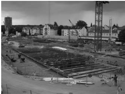
a) Execution of the middle strip
