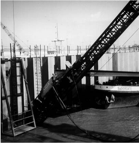
Fig. 6.4. Anchor pile for sea wall, driven with an hydraulic pile driver
