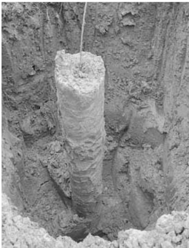
Fig. 7.20. Excavated lime column (after Kempfert and Raithel 2005)
