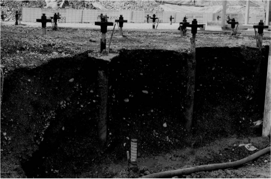
Fig. 6.23. Completed GEWI piles with postgrouting hoses
