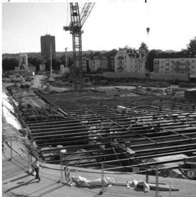
c) Execution of the strip on hafen street side
