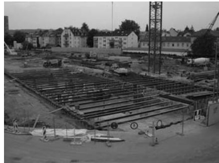
b) Execution of the strip next to part II
