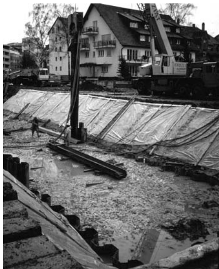
Fig. 4.1. Sloped excavation with surface protection
