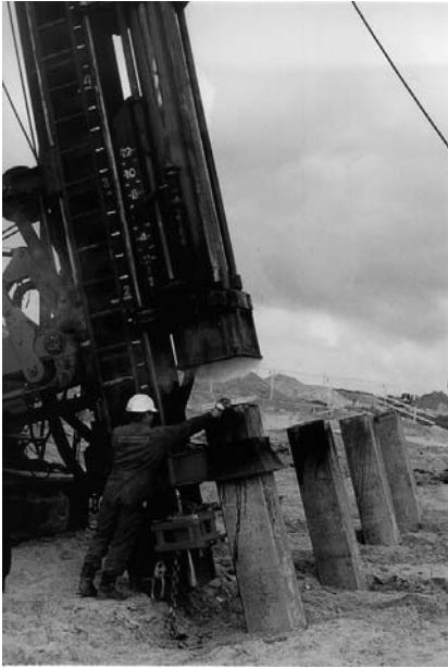
Fig. 6.6. Driving of a reinforced concrete piles on a batter with an hydraulic pile driver (photo: "Centrum Pfähle")
