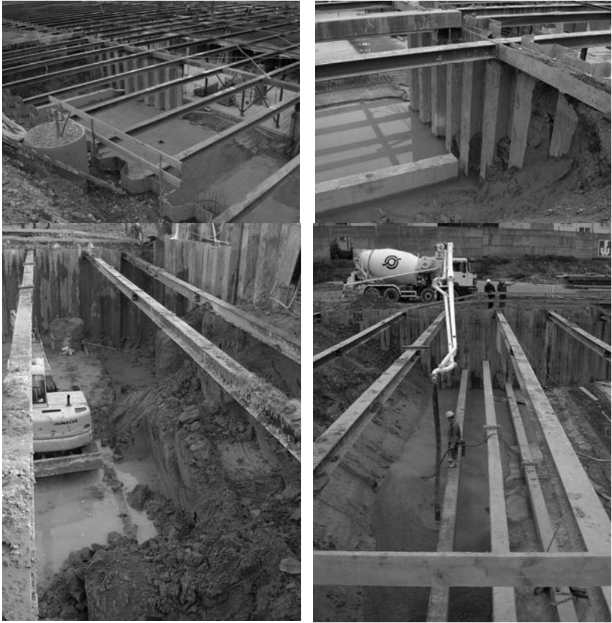
Fig. 4.130. Some details of construction works with blockwise excavation and bottom slab placement
