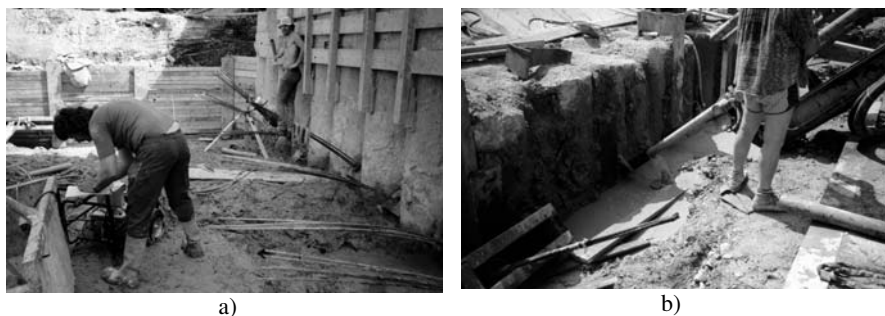
Fig. 4.9. a) Back anchored pile wall for protection of existing building near an excavation (see also Fig. 4.7); b) anchor boring with the help of casing for the part of the anchor hole in the soft soil layer
