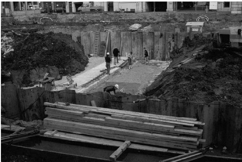
Fig. 4.87. Excavation and placement of the bottom slab in slices
