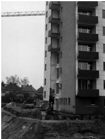
Fig. 6.90. a) Existing building with excavated injection piles, b) Injection pile head and stepwise installation of the raft foundation (project IV)
