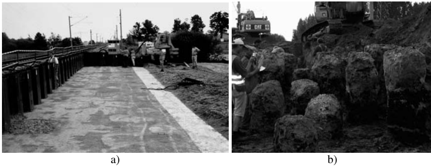
Fig. 7.38. Test field: a) Temporary sheet pile walls and excavated embankment; b) excavated columns with different heights
