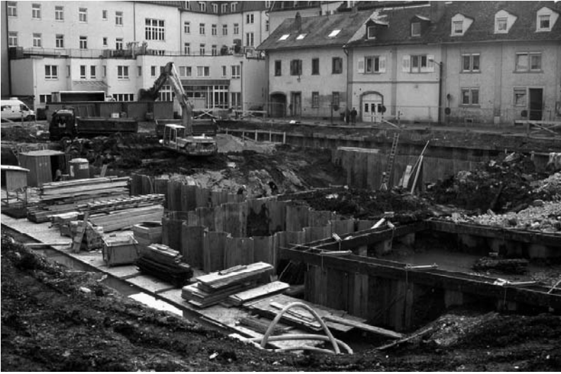
Fig. 4.86. Overview of the excavation site
