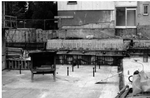
Fig. 6.90. a) Existing building with excavated injection piles, b) Injection pile head and stepwise installation of the raft foundation (project IV)
